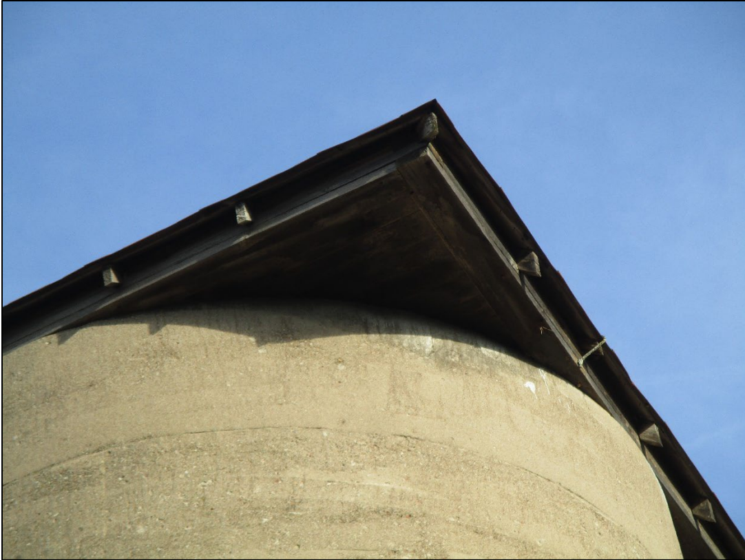
Figure 9: Detail View showing roof construction
