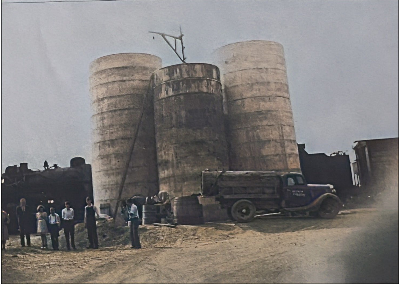
Figure 11: Harris Grain Elevation under construction, 1943 (Rymal Station Heritage)
