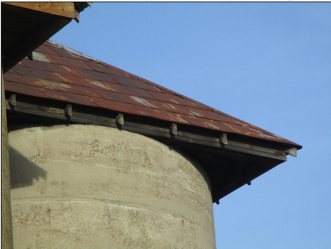
Figure 8: Detail View showing roof construction
