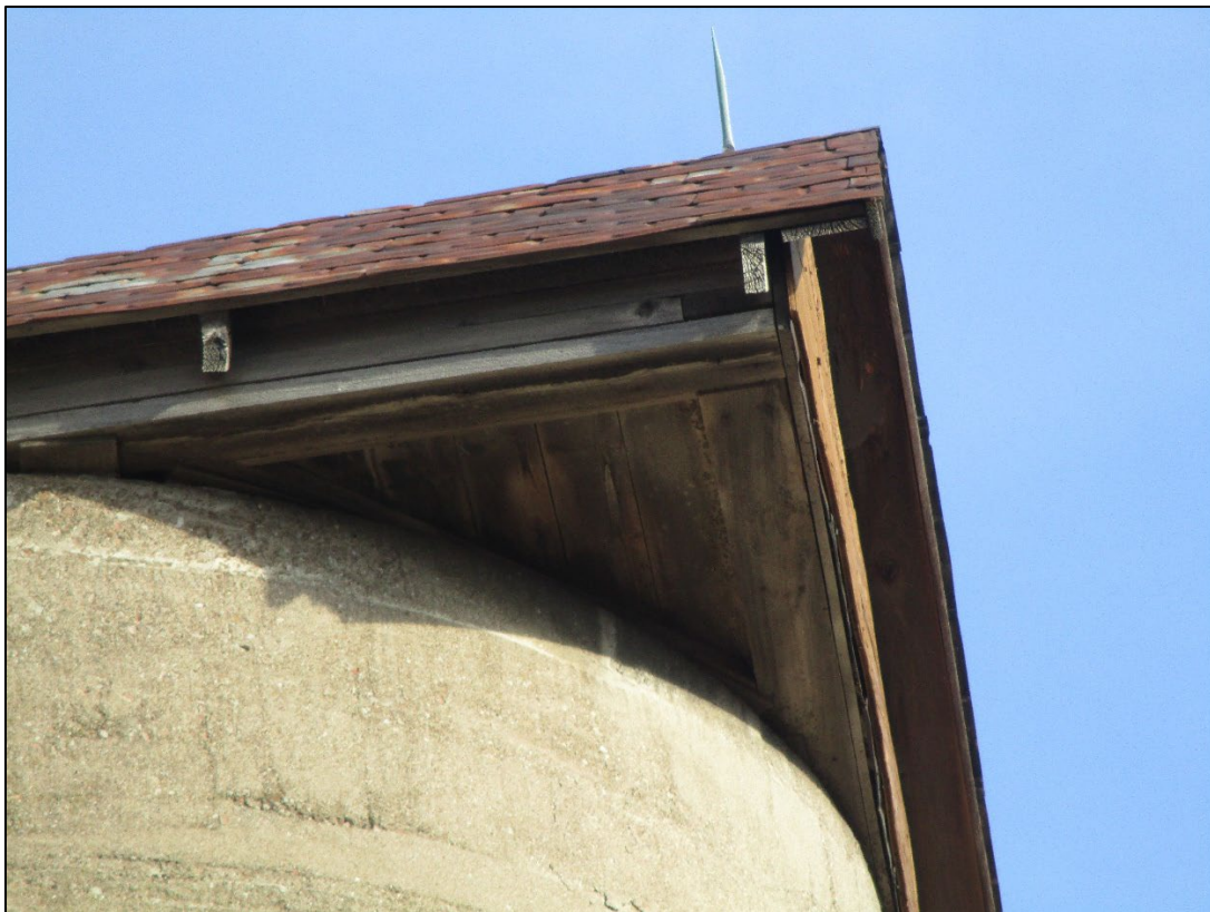
Figure 10: Detail View showing roof construction
