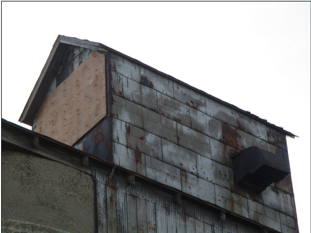
Figure 6: Detail View of Headhouse
