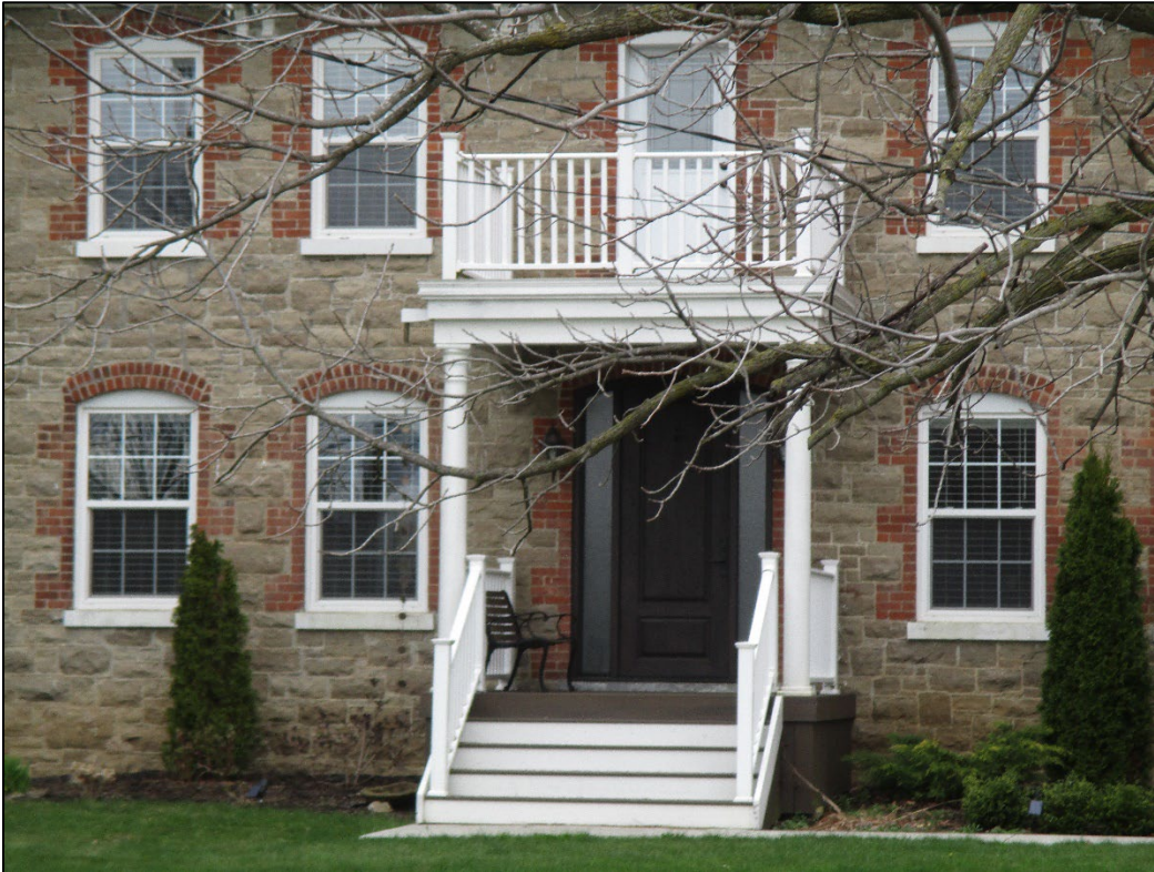
Figure 7: Detail view of front porch and entrance
