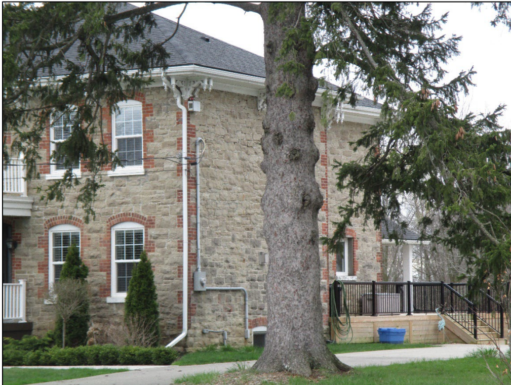
Figure 4: Detail view of north elevation
