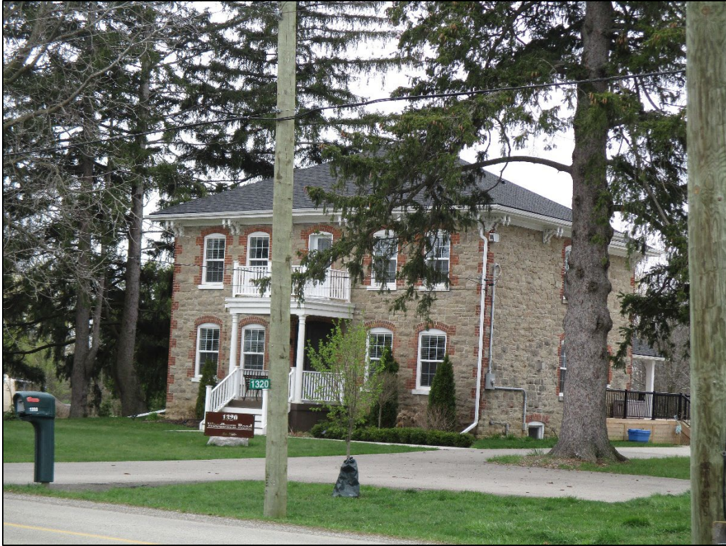
Figure 2: View of northeastern elevation
