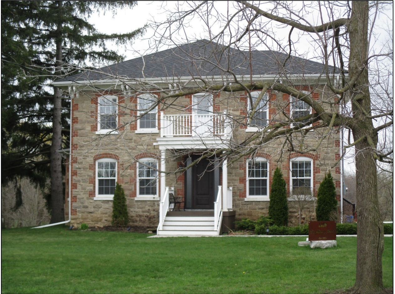
Figure 1: Front Elevation of Subject Property
