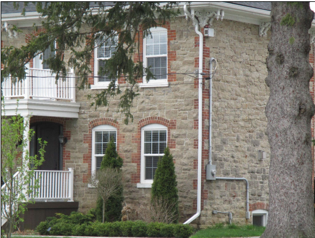
Figure 5: Detail view of brickwork
