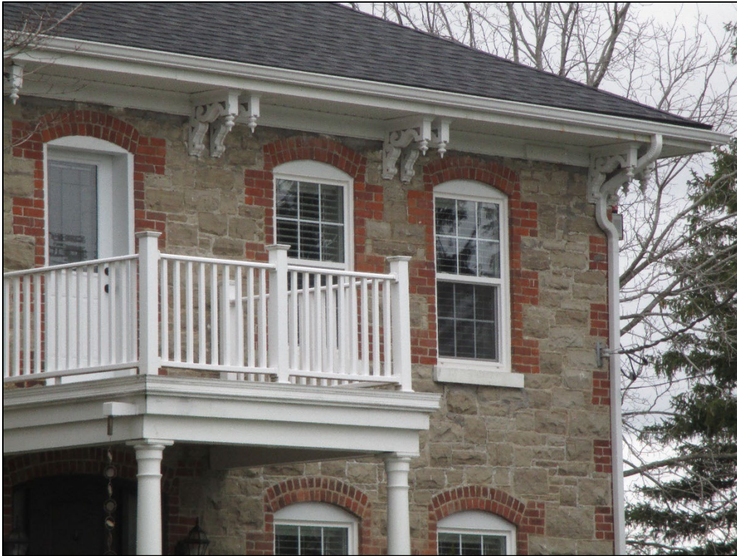
Figure 6: Detail view of brickwork and decorative brackets
