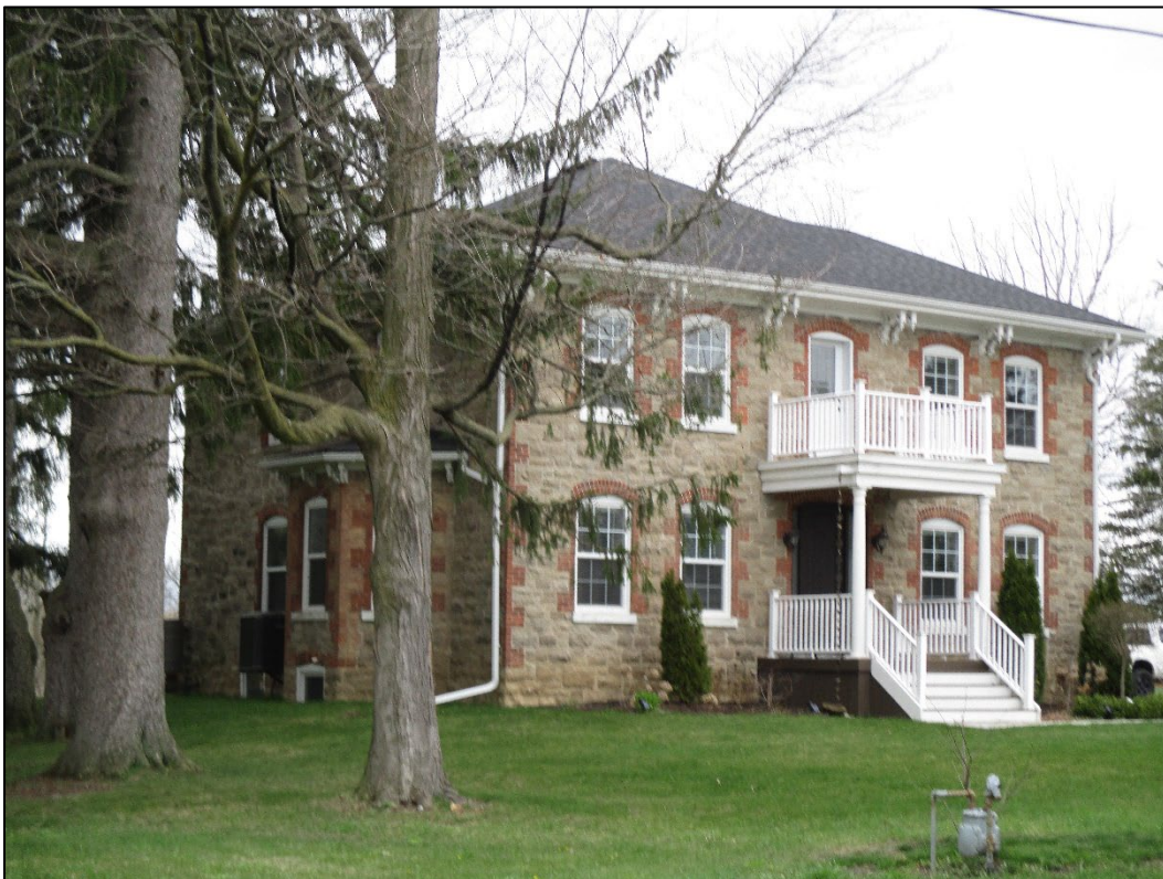
Figure 3: View of southwestern elevation
