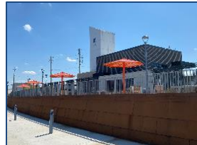
Pier 8 Sanitary Pumping Station
