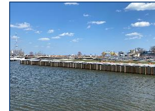
Pier 6&7 Shorewall & Public Boardwalk
