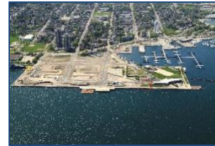
Shorewall Infrastructure Renewal
