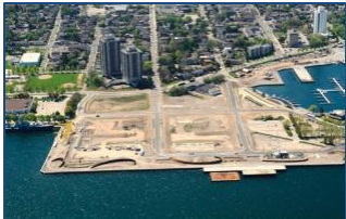
Pier 8 Servicing Infrastructure
