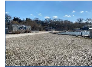
HPS Marine Unit & Rehabilitation
