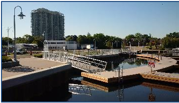
Pier 7 Shorewall, Boardwalk & Boat Slips
