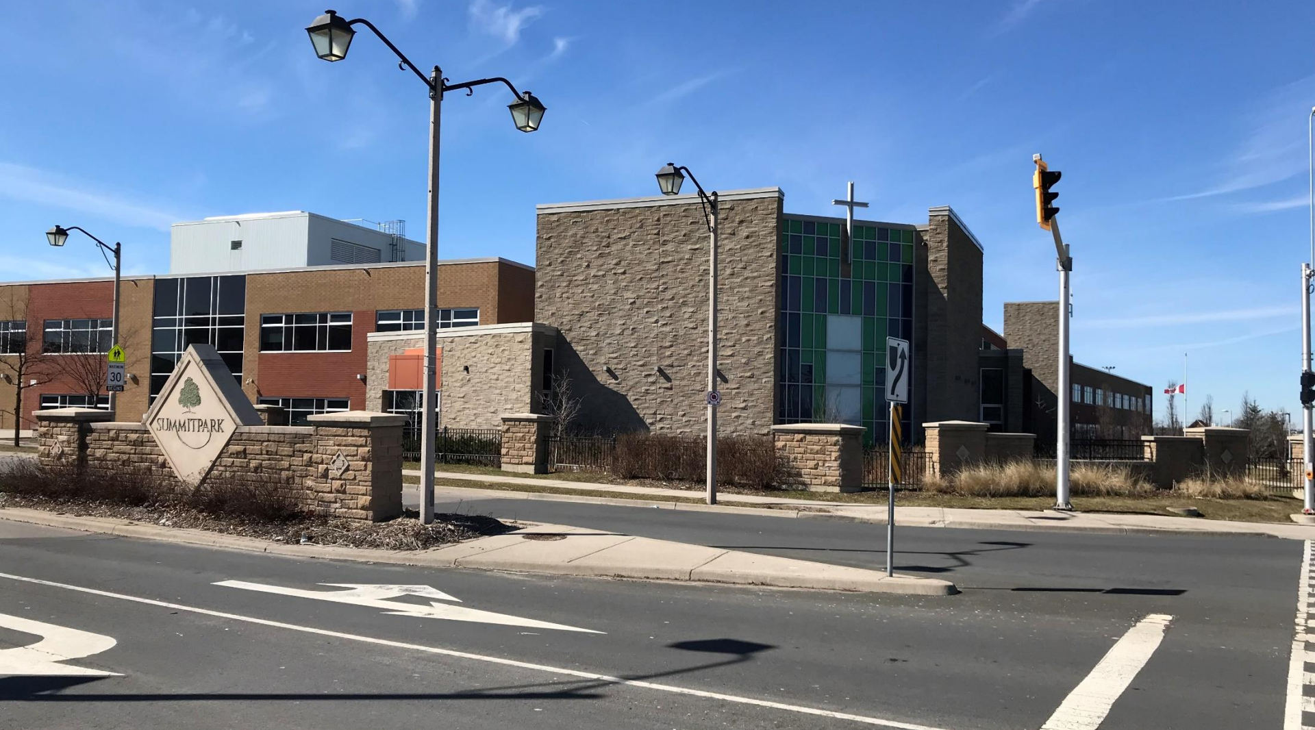
Bishop Ryan Catholic Secondary School, located to the west
