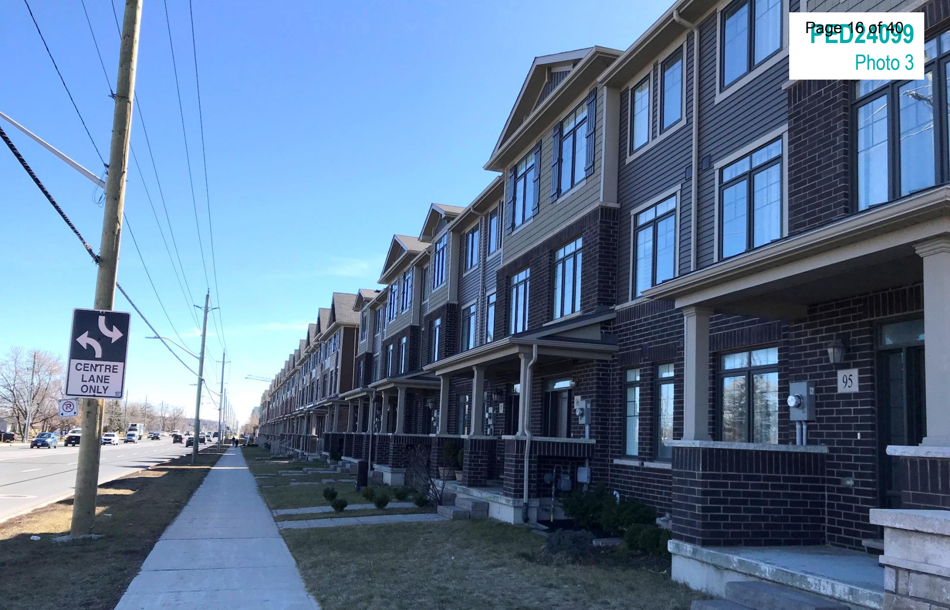
Adjacent development to the east
