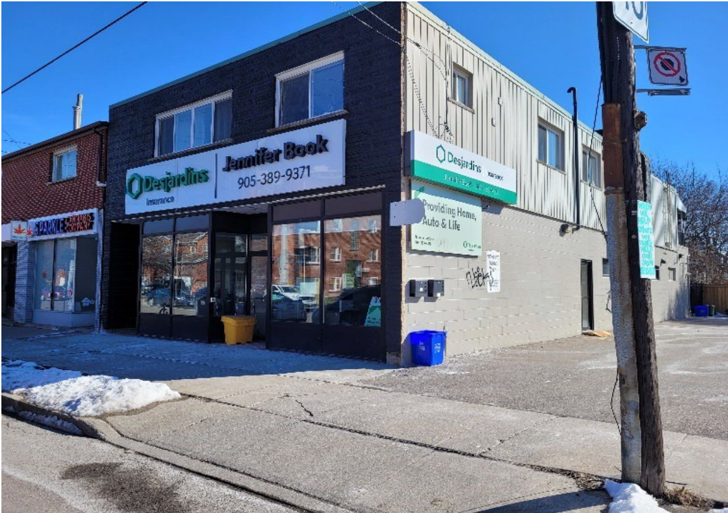
776 Concession Street, Hamilton (Source: CDSB Staff)
