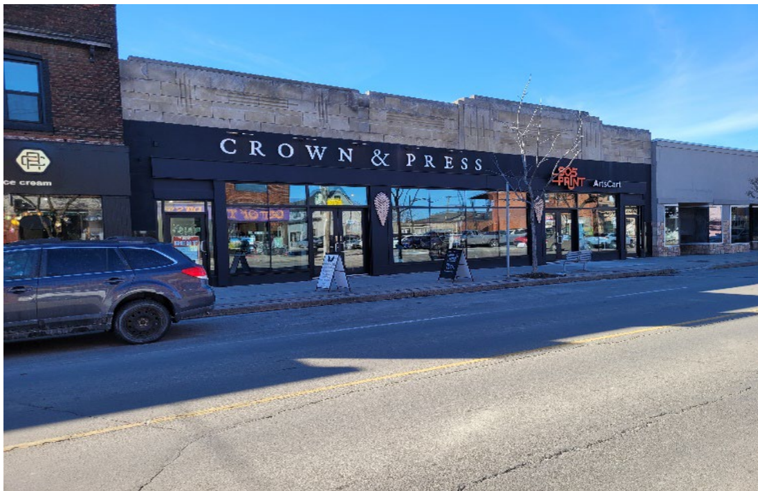
304 Ottawa Street North, Hamilton (Source: CDSB Staff)
