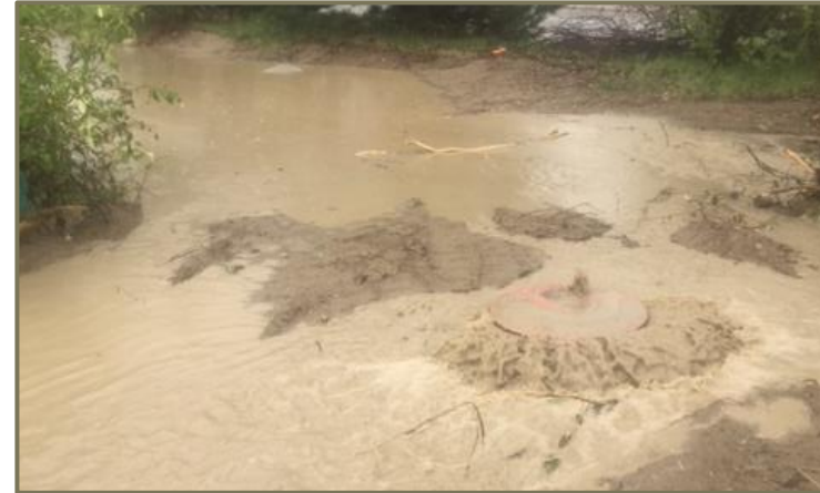
System Surcharge/ Basement Flooding
