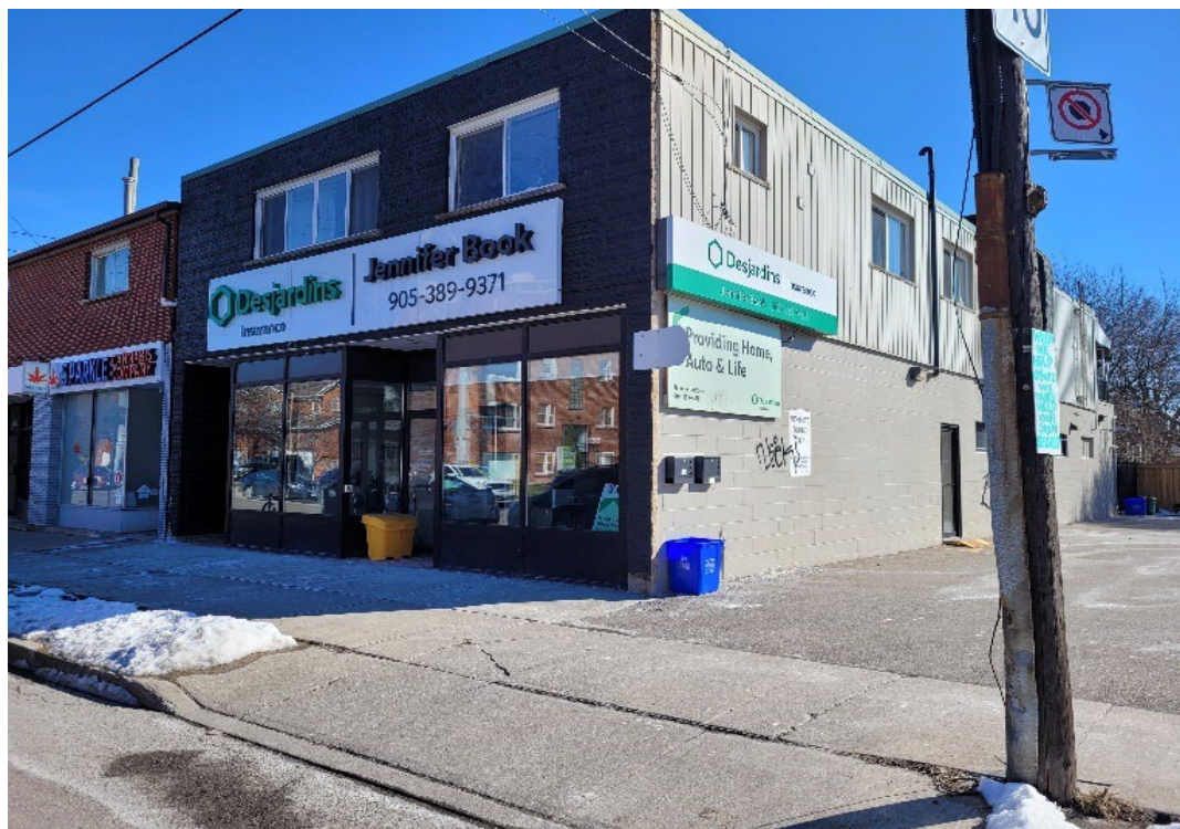
776 Concession Street, Hamilton (Source: CDSB Staff)
