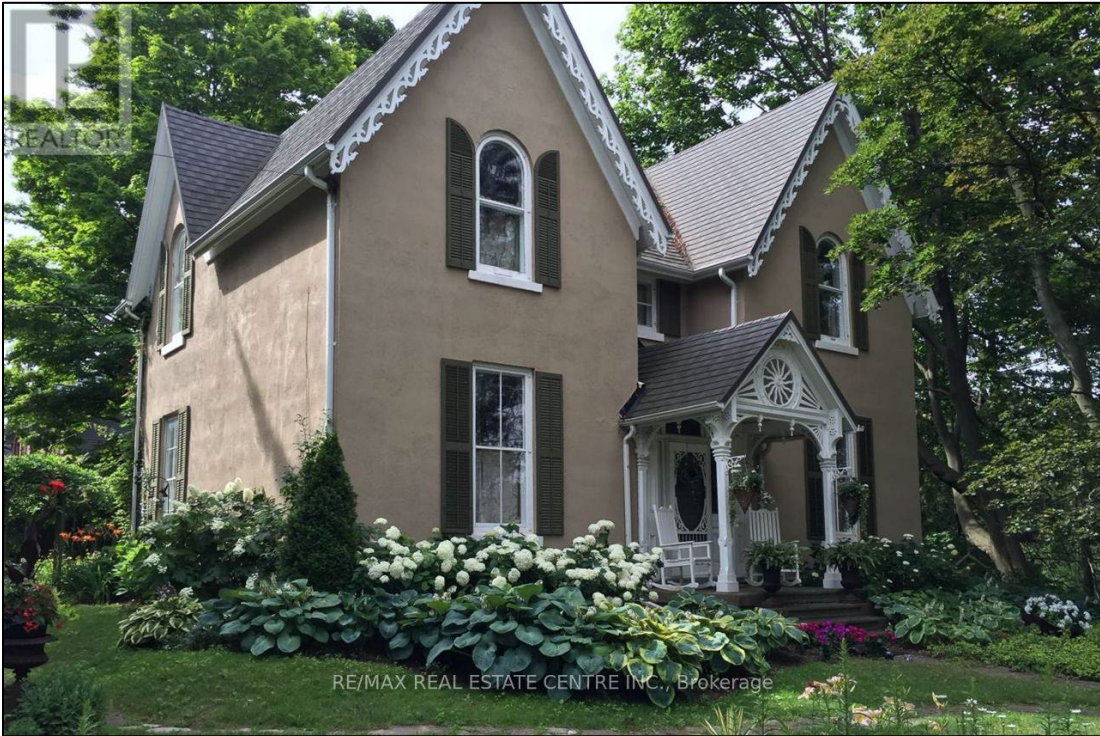
Figure 3: Front (north) elevation (Royal LePage, 2024)
