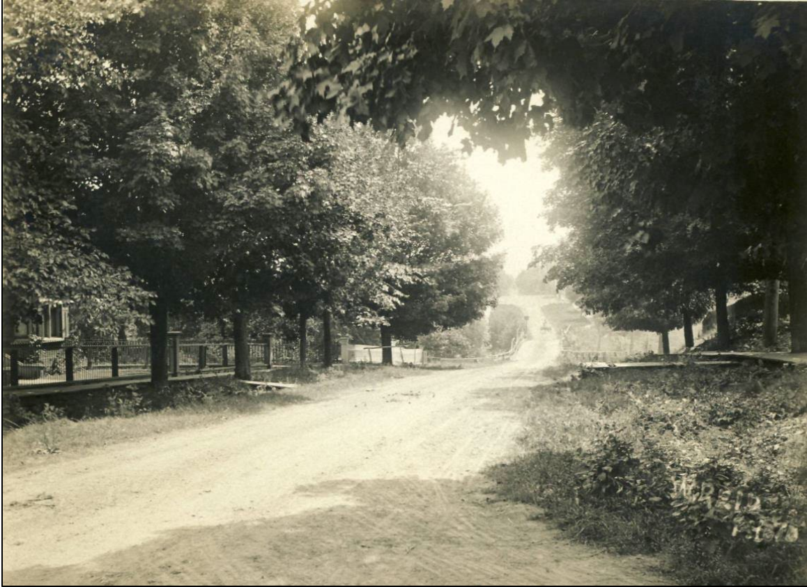
Figure 11: Looking west along Dundas Street to Bridge, c. 1907 (Flamborough Archives)
