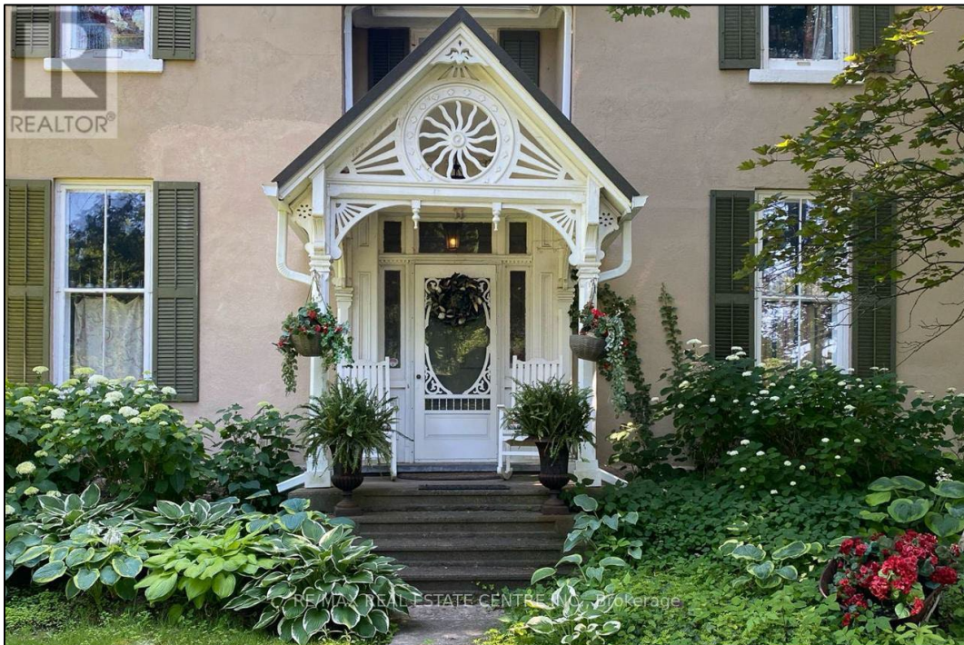
Figure 4: Detail view of front porch and entryway (Royal LePage, 2024)
