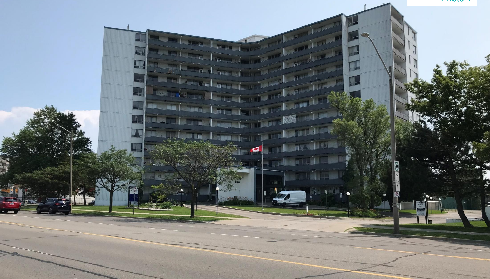
Subject site – existing apartment building
