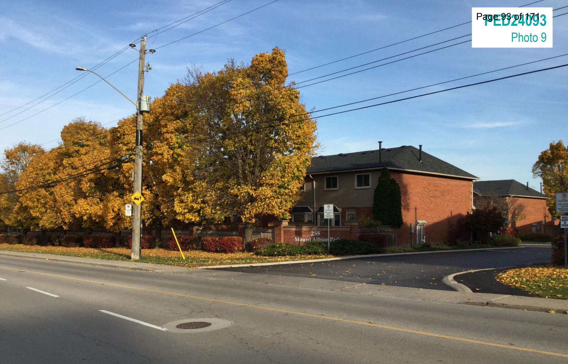
Existing townhouse dwellings located to the east of the subject property, as seen from Mount Albion Road looking north east
