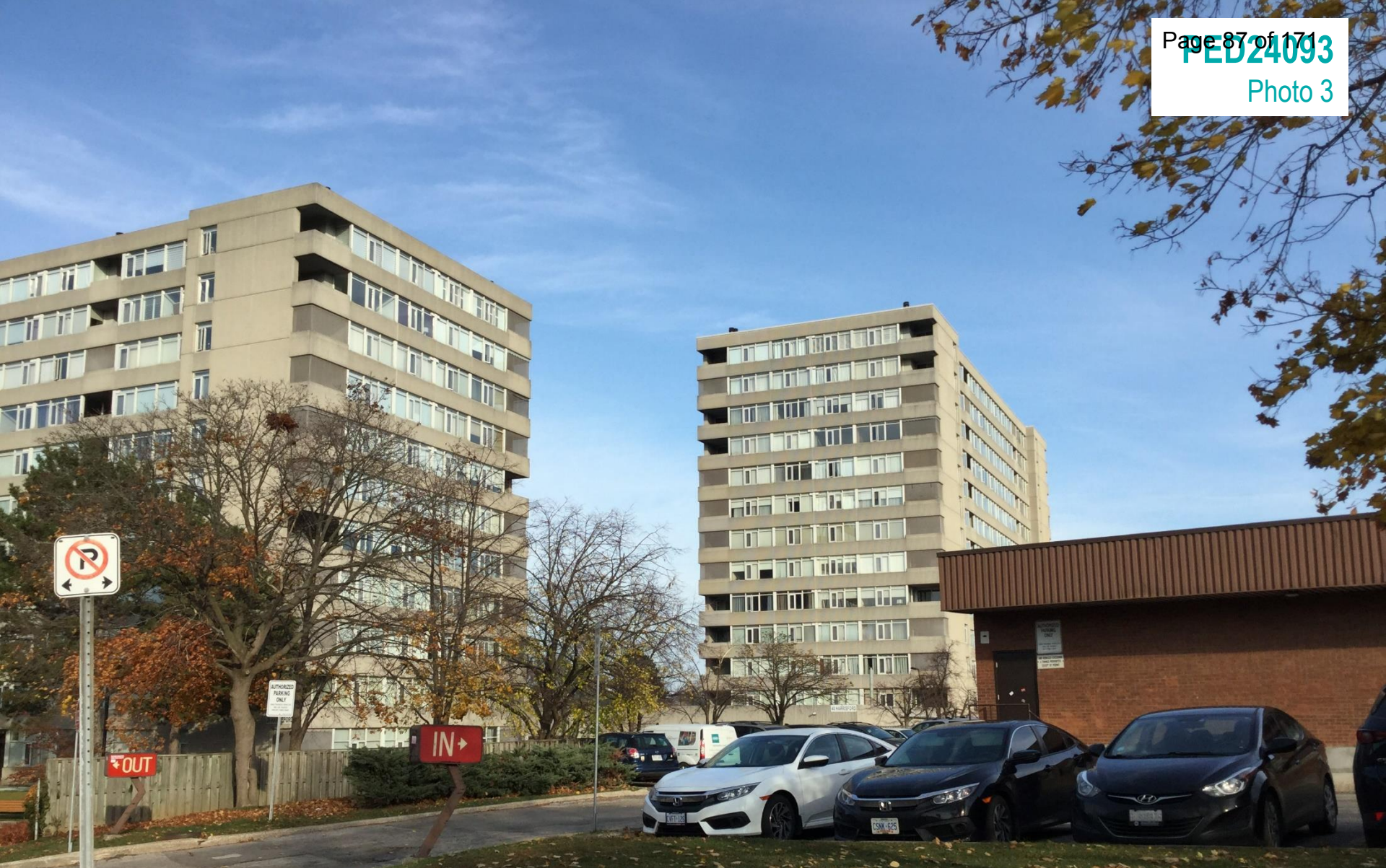
Subject property and the existing 12 storeys multiple dwelling at 30 and 40 Harrisford Street located to the north of the subject property, as seen from Harrisford Street looking north east
