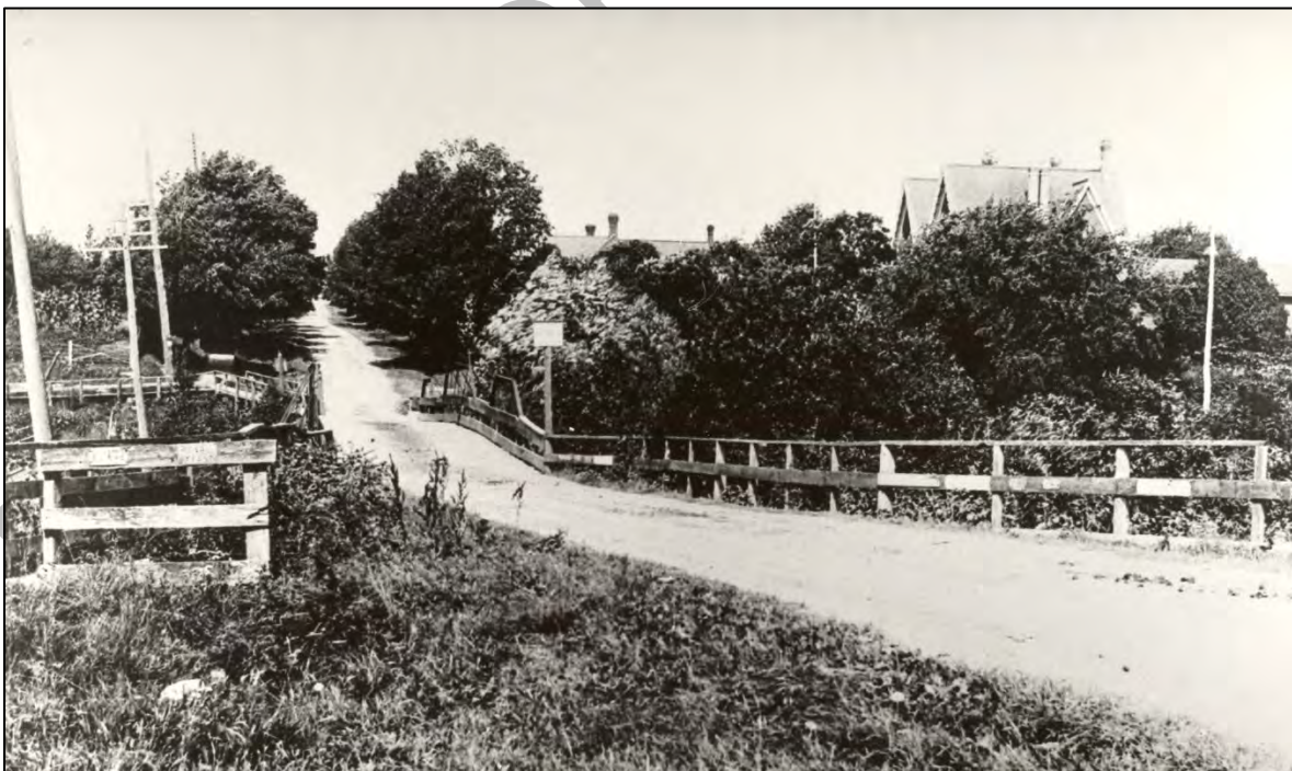
Image 10: Looking east across the Dundas Street Bridge into Vinegar Hill, showing the Eager House on the right, c.1900, Source: Flamborough Archives, BW 771
