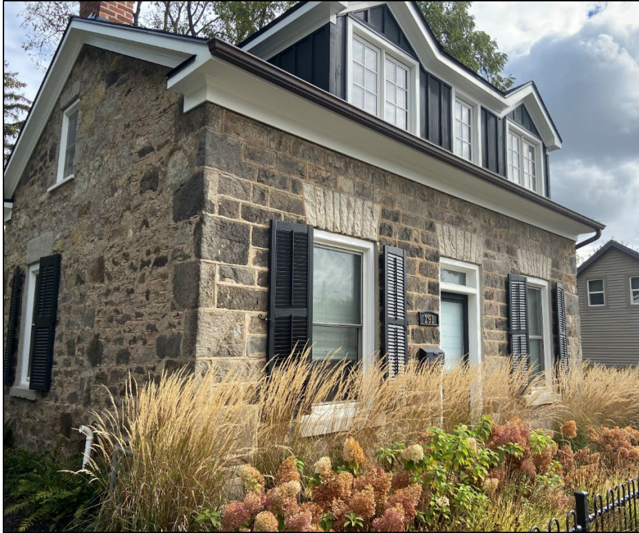
Image 2: Front (southern) and side (western) elevations, from the southwest.
