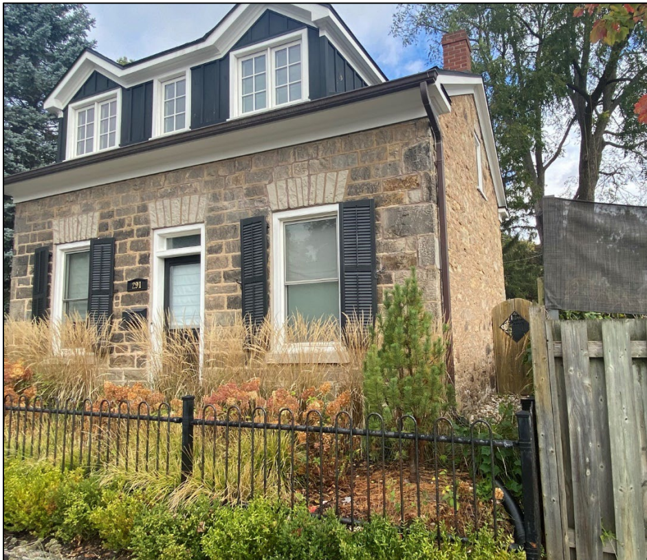
Image 3: Front (southern) and side (eastern) elevations, from the southeast.
