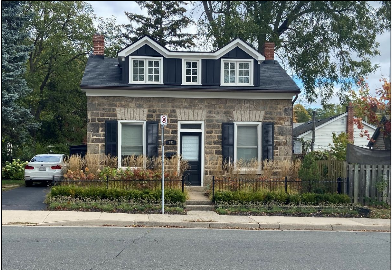
Image 1: Front (southern) elevation, from the south.
