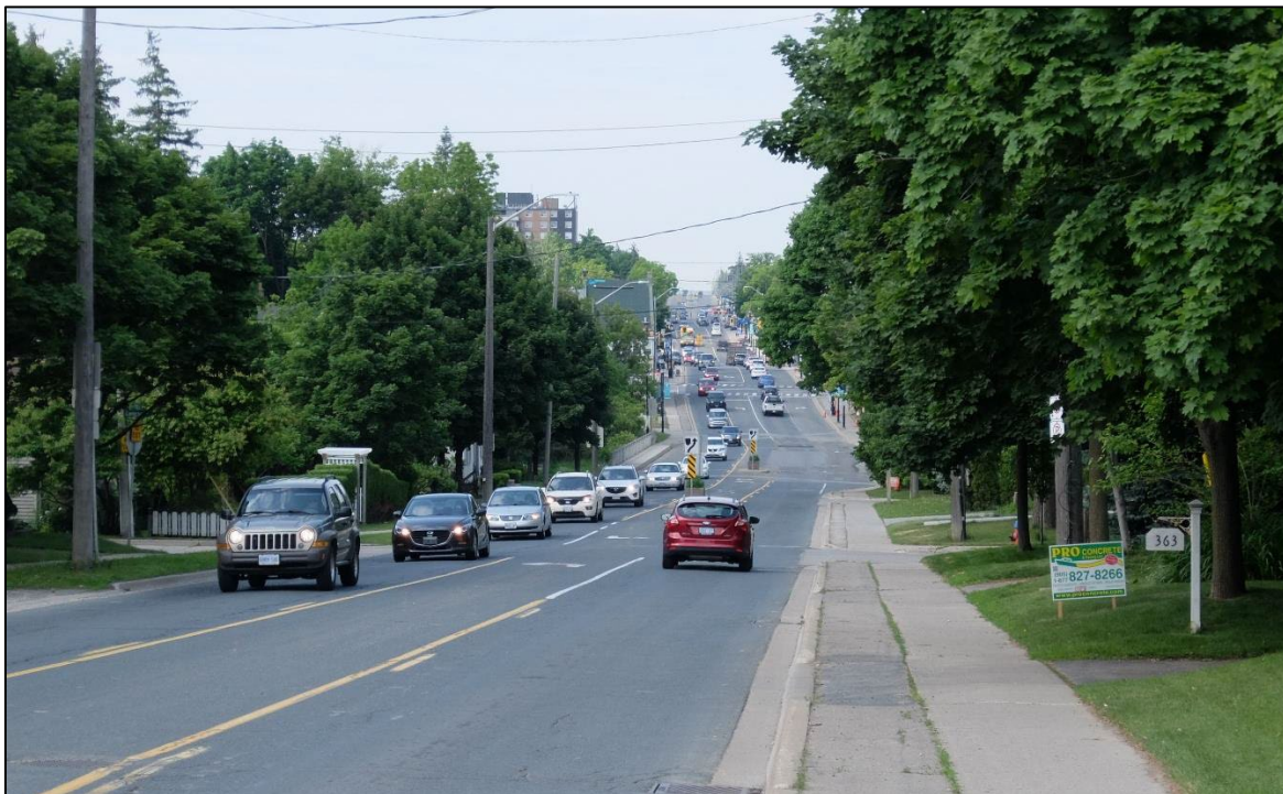
Figure 10: Looking west along Dundas Street to Bridge
