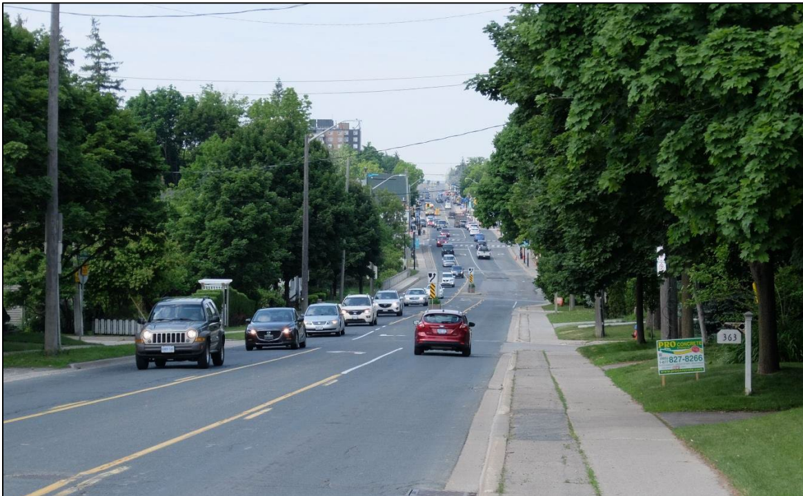
Figure 10: Looking west along Dundas Street to Bridge
