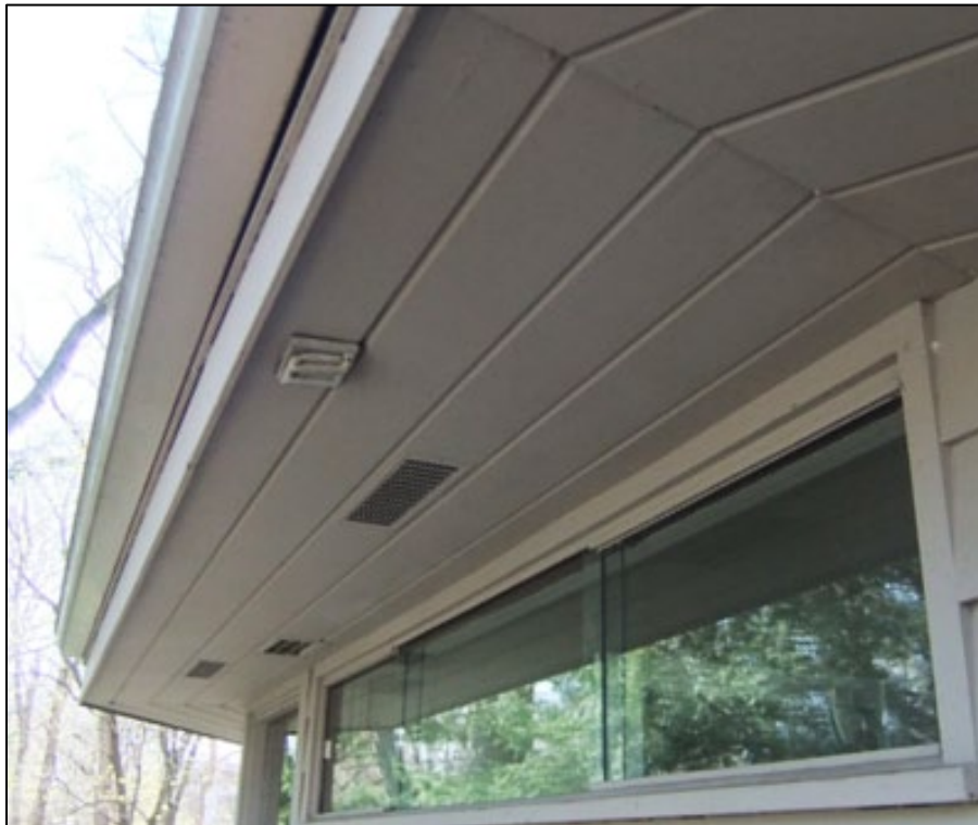
Image 6: Close-up detail of the second storey soffits and transom windows.
