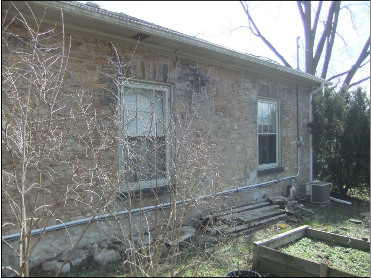
Image 5: Western elevation from a northern vantage point.
