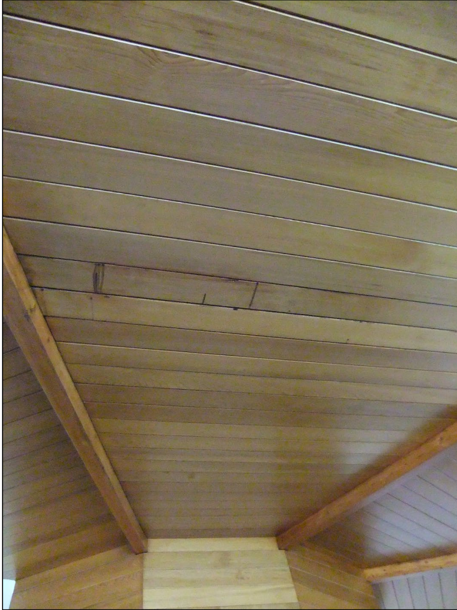
Image 17: Close up detail of the stained cedar ceiling.
