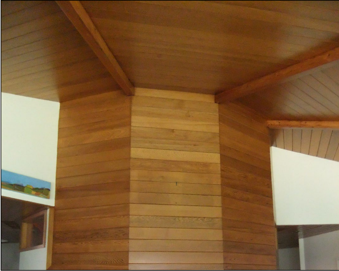
Image 15: Image of the stained cedar ceiling, radiating from the center of the building.
