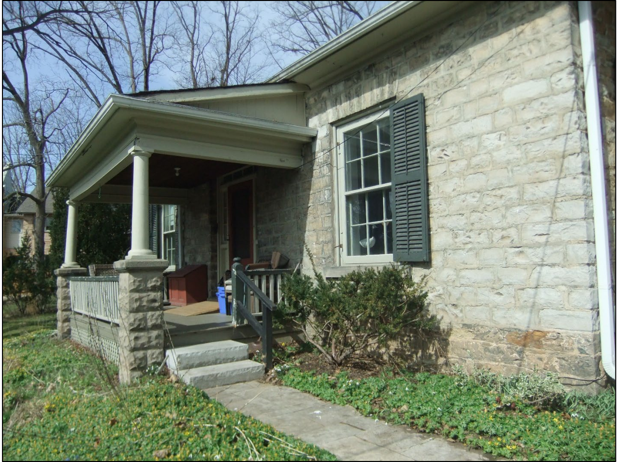
Image 4: Front (southern) elevation from an eastern vantage point.
