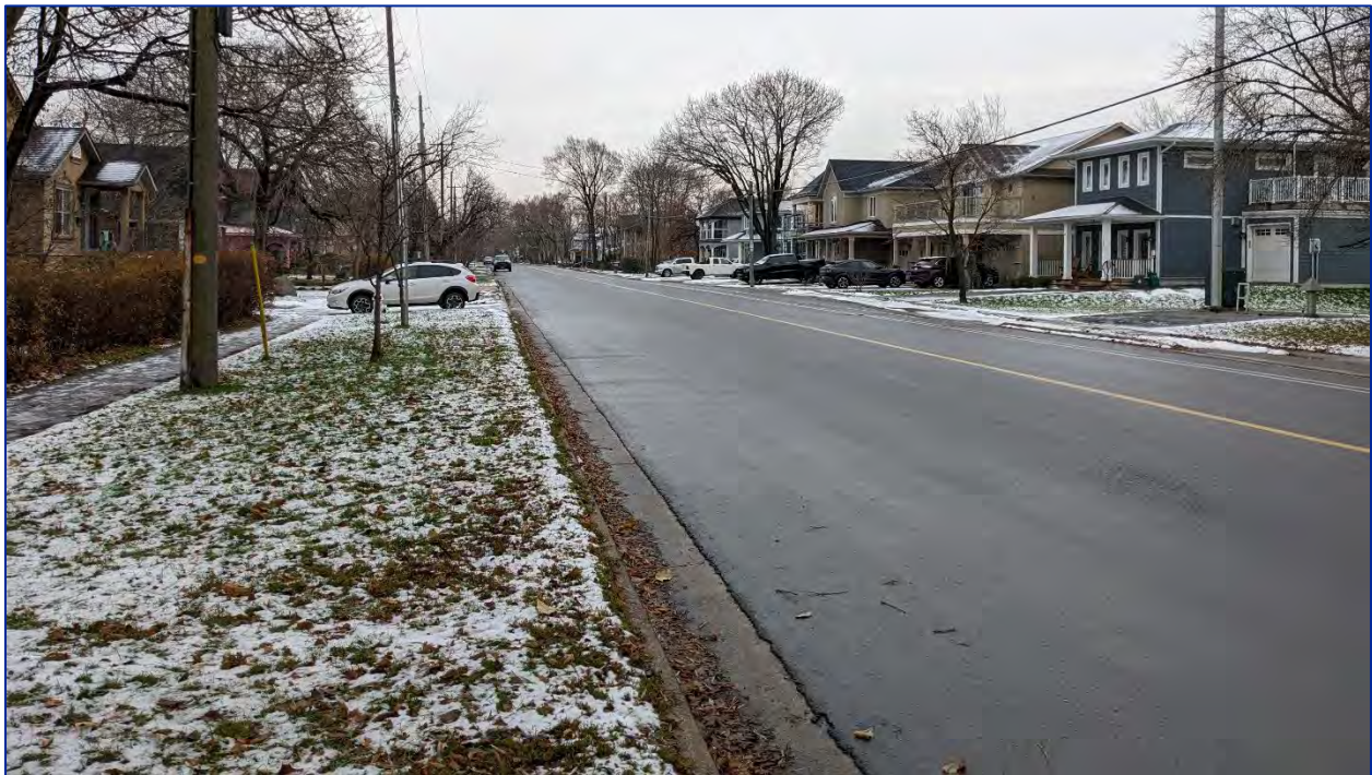
Figure 30: View south along Beach Boulevard from in front of 957 Beach Boulevard
