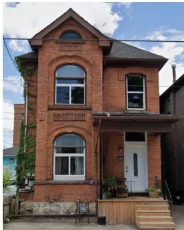
Figure 28. 148 Catharine Street North (Google Maps, 2022).
