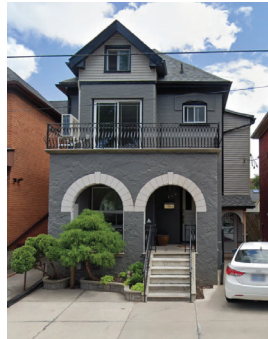
Figure 27. 146 Catharine Street North (Google Maps, 2022).
