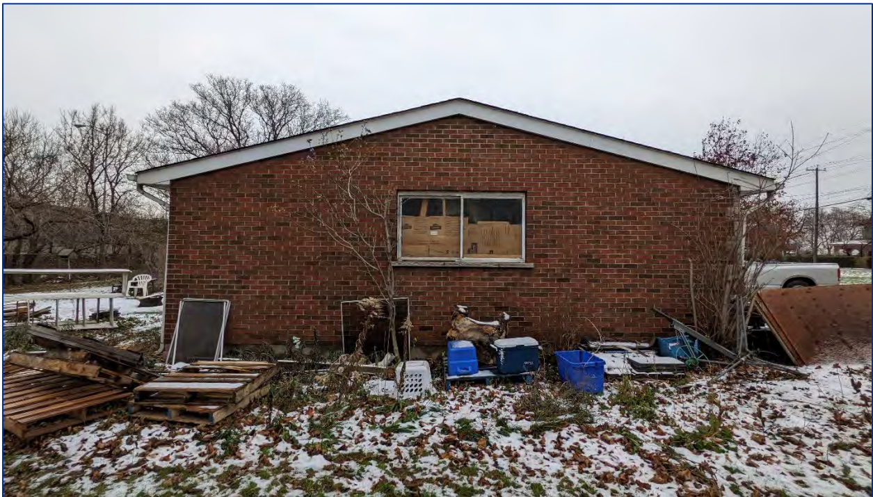
Figure 22: View of the south elevation of the detached garage
