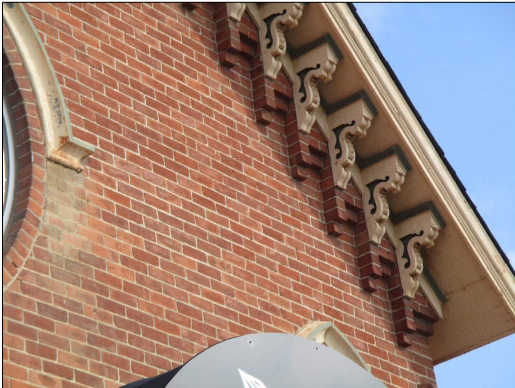
Figure 7: Detail view of carved brackets on south elevation.
