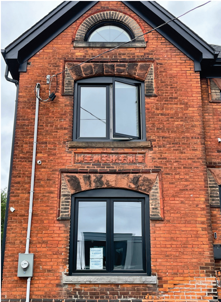
Figure 16. Primary (east) elevation of the residential building located at 89 Catharine Street North showing the windows and rectilinear hood moulds. Page 22
