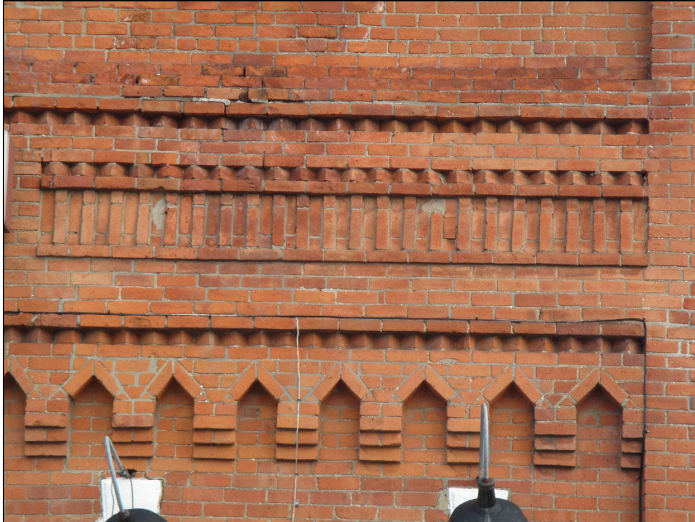
Figure 9: Detail view of decorative brickwork elements.
