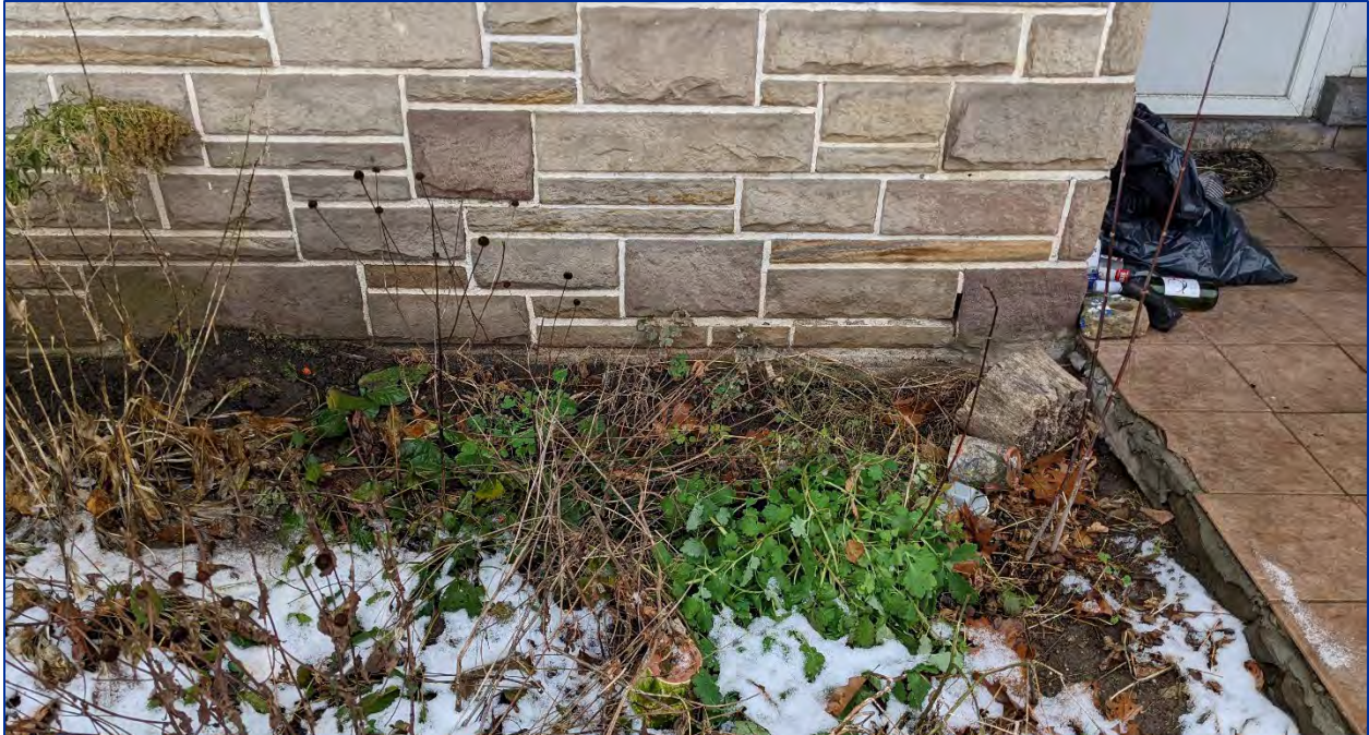
Figure 16: View of the residence's concrete foundation
