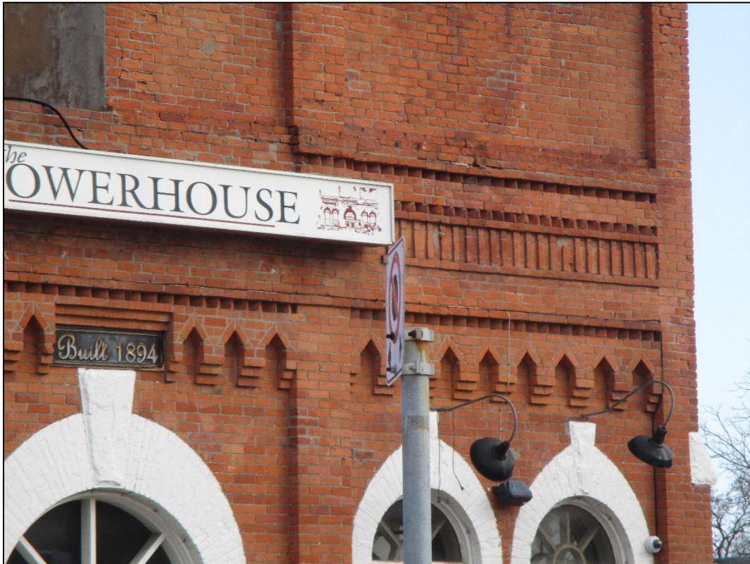
Figure 8: Detail view of decorative brickwork elements.
