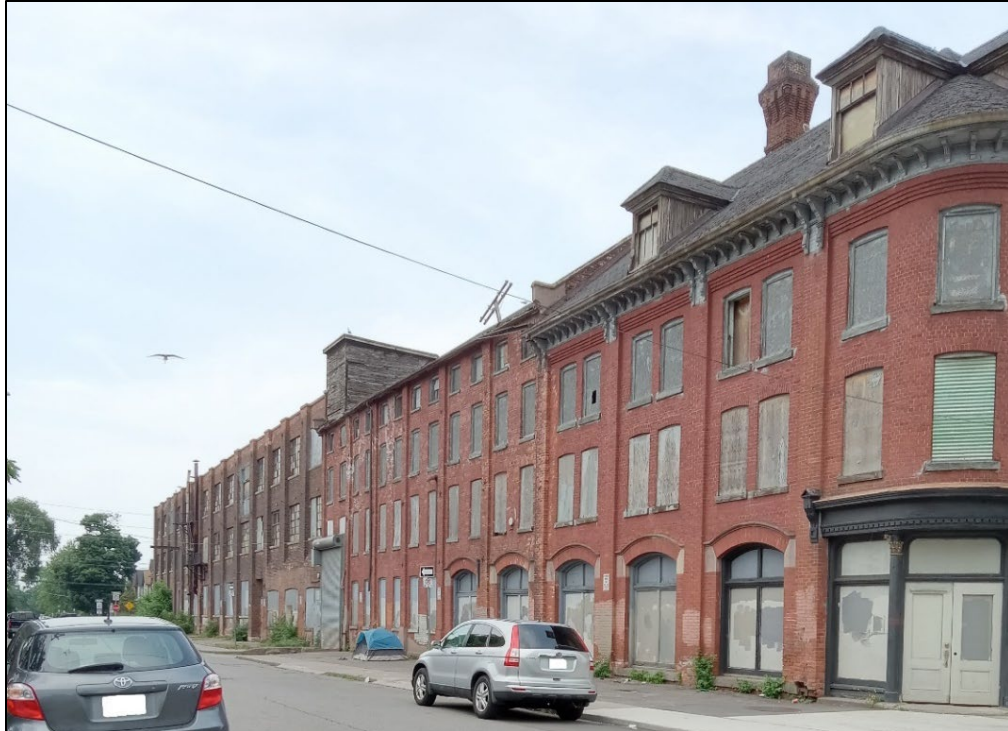
Figure 13: West elevation looking north along Mary Street, including 122 Mary Street (Structure 2, right), 130 Mary Street (Structure 1, middle right) and 140-146 Mary Street (Structure 4, left).
