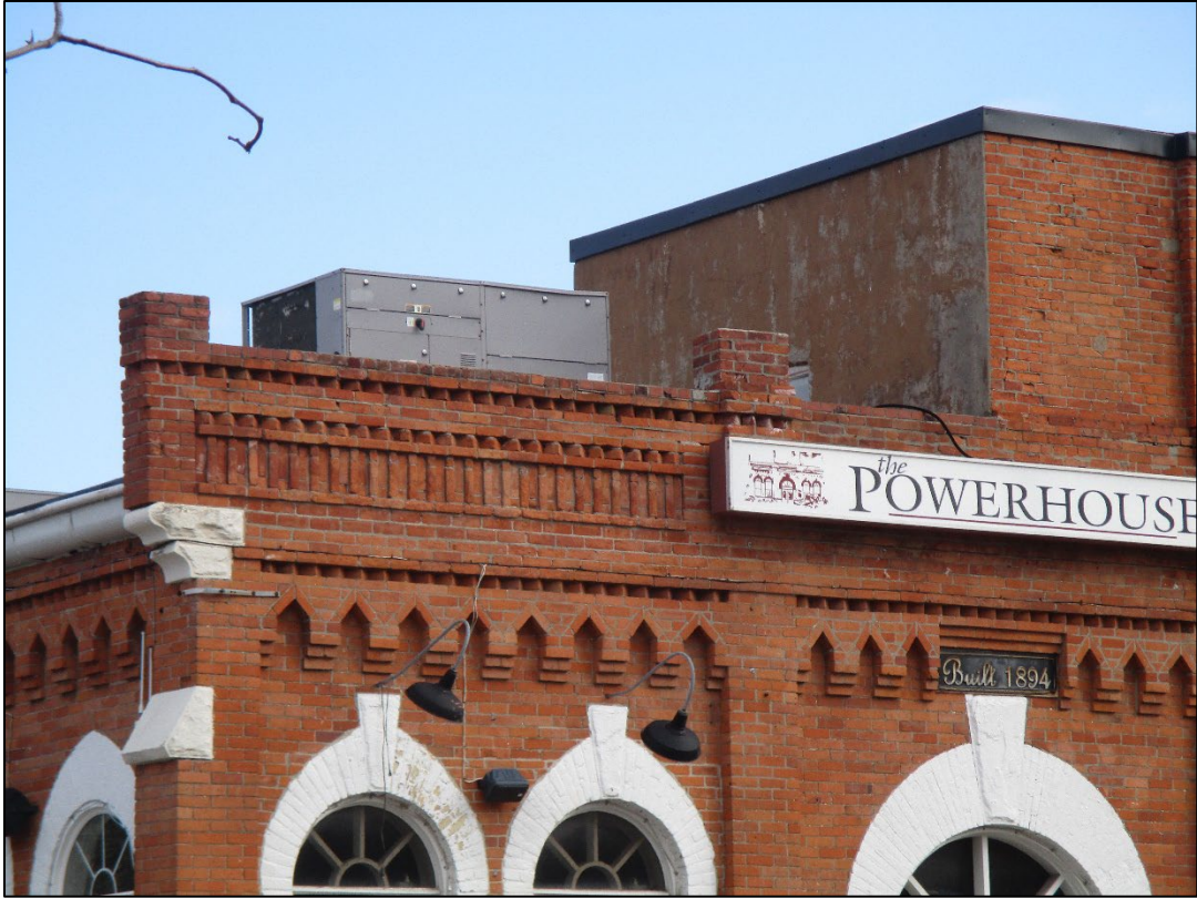
Figure 7: Detail view of parapet with decorative brickwork.
