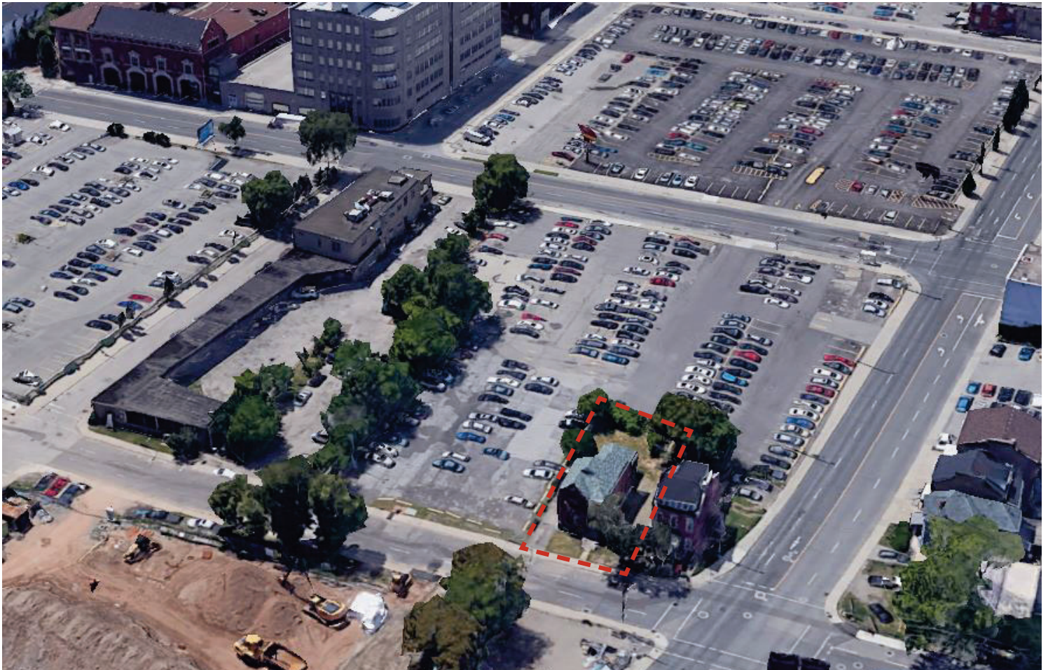
Figure 11. Aerial view of 85 Catharine Street North, looking towards the west. The property is outlined in red (Google Earth, 2024, annotated by mcCallumSather).
