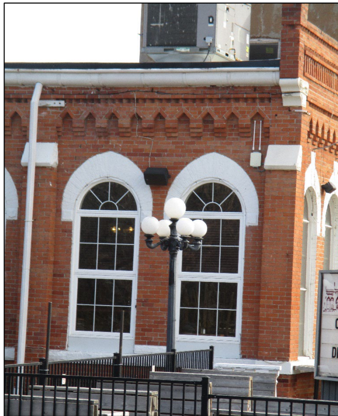
Figure 10: Detail view of windows and buttresses on west elevation.
