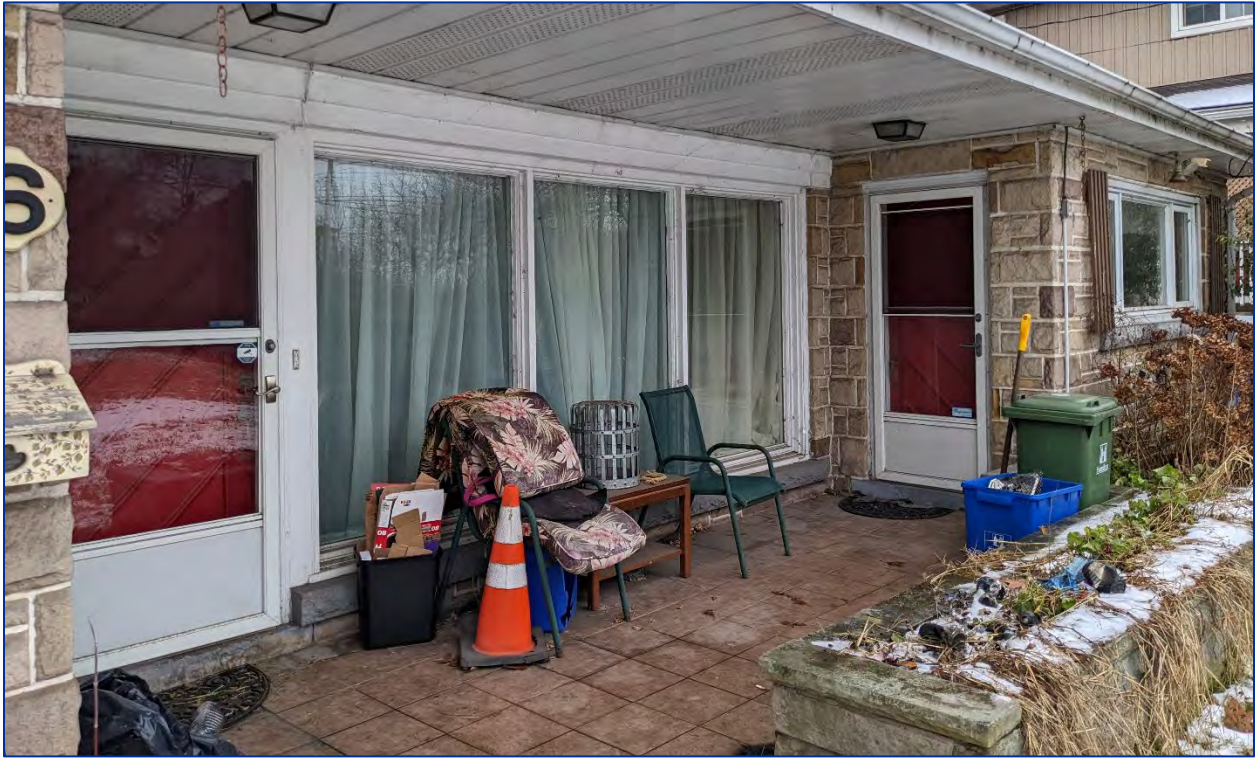
Figure 19: View of the inset covered porch
