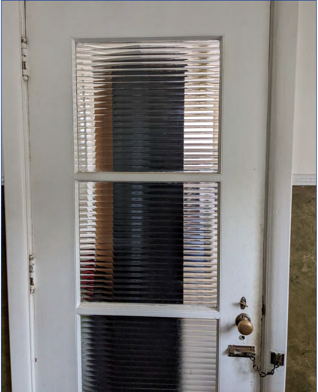
Figure 20: View of the interior of the boarded-up door
