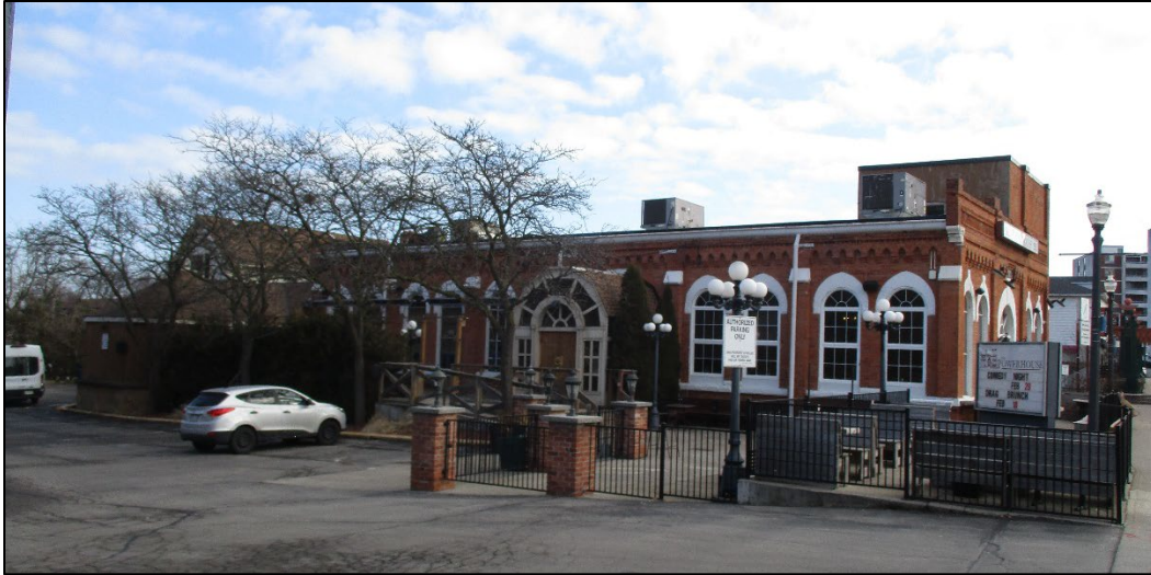
Figure 3: West elevation showing modern entrance.
