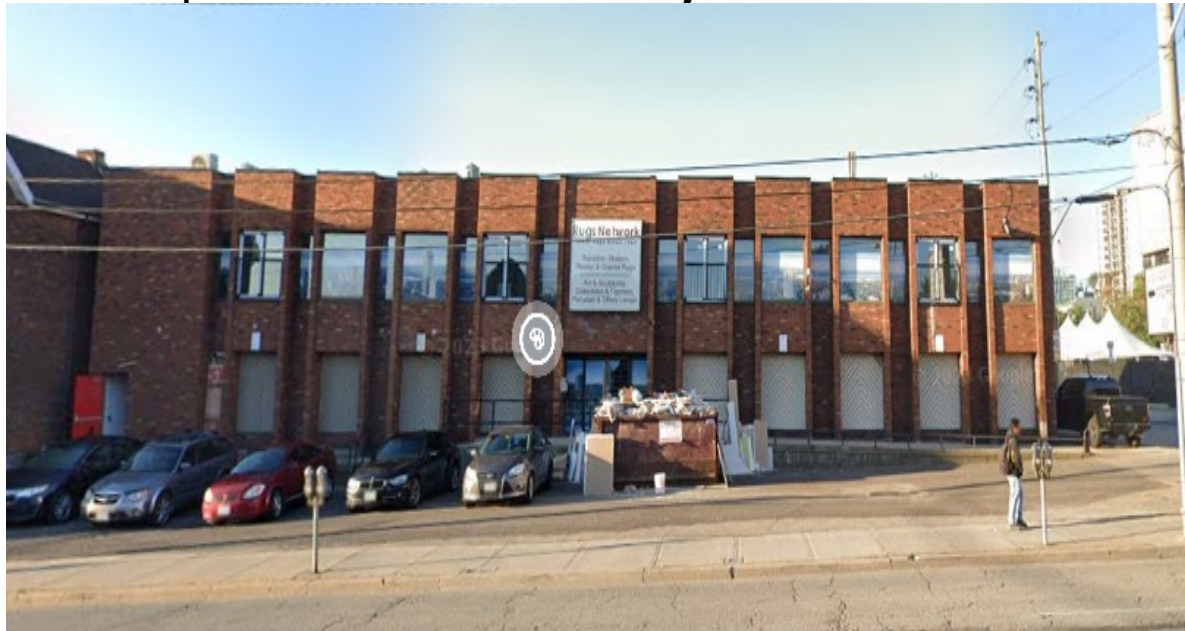
View looking south toward the northern elevation
