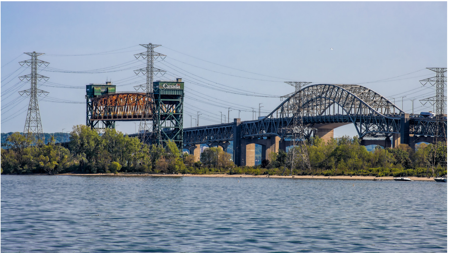
Burlington Canal Lift Bridge. STOCK PHOTO
