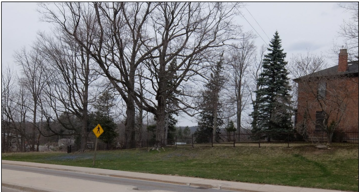
Figure 14: Looking west from Governor's Road, April 11, 2023
