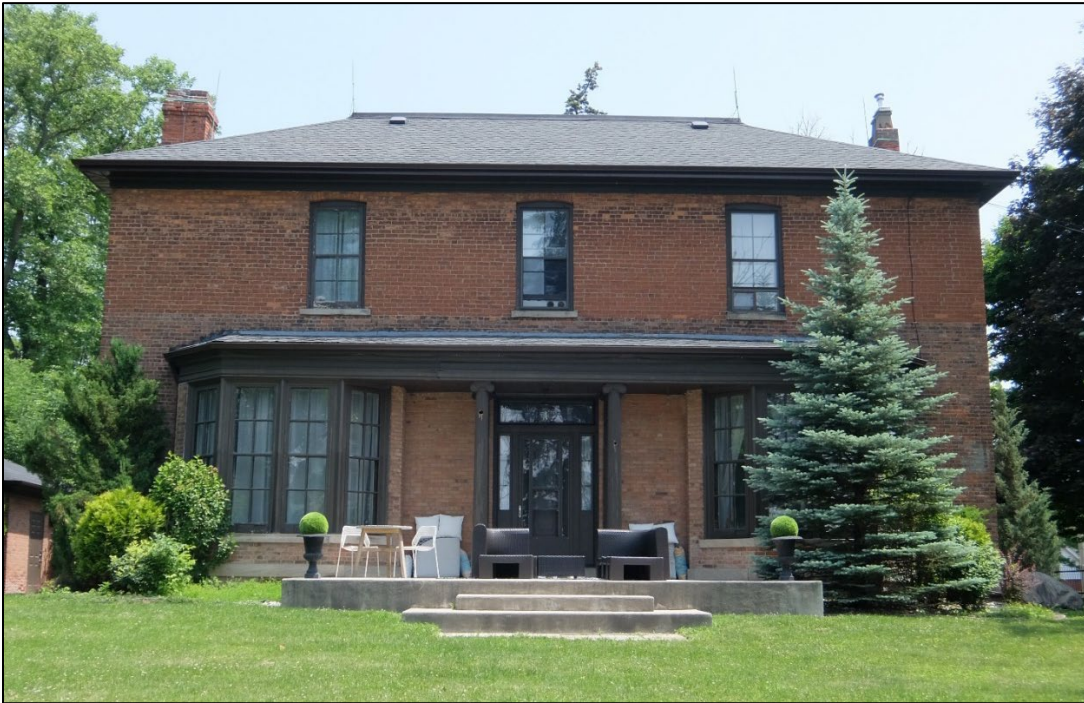
Figure 1: 223 Governor's Road, west elevation
