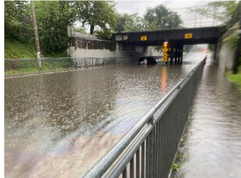
August 2023 – Birch Avenue flooding
