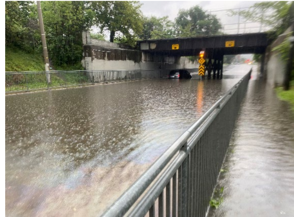
August 2023 – Birch Avenue flooding
