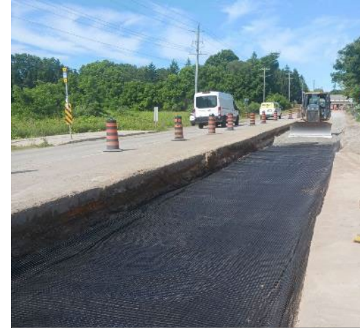
Garner Road: geo-grid installation
