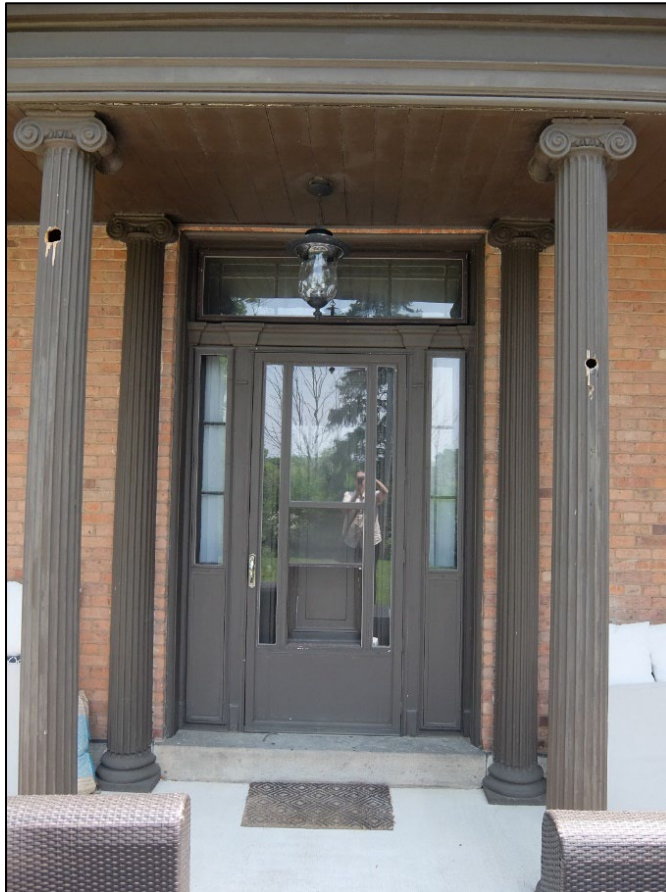
Figure 8: Closeup of front entryway on west elevation
