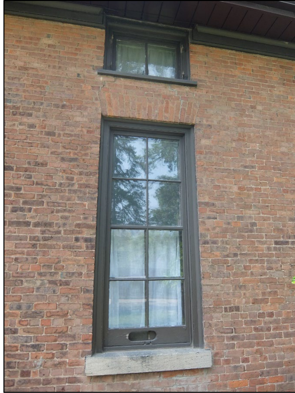
Figure 11: Closeup of east elevation windows
