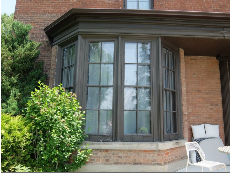
Figure 7: Closeup of bay window on west elevation
