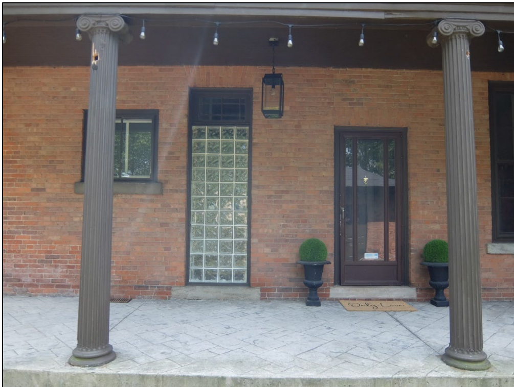
Figure 12: Closeup of northeast elevation entryway
