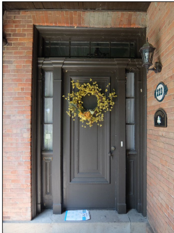
Figure 10: Closeup of southeast elevation entryway
