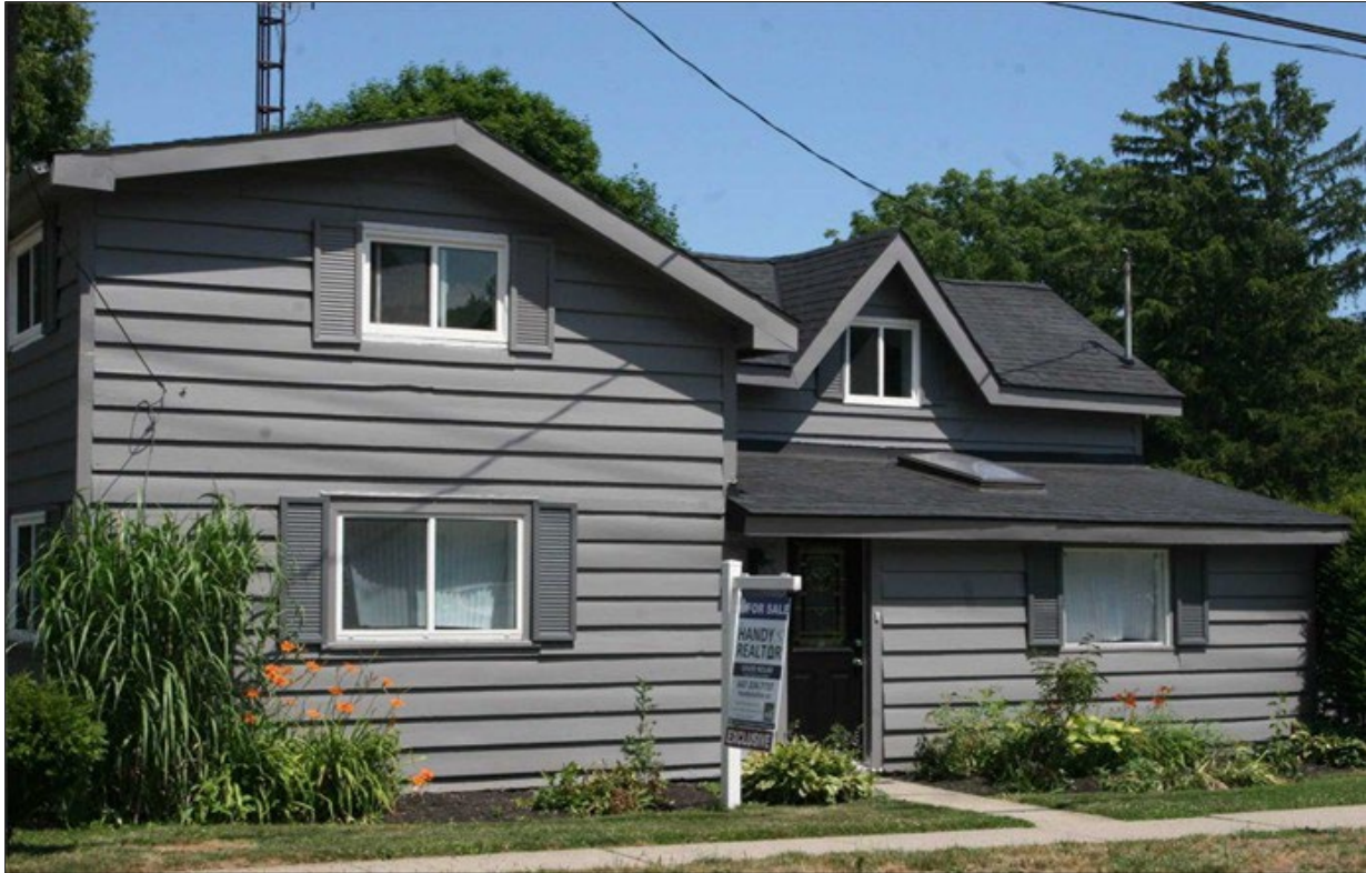
Figure 5: Side (west) elevation of 2 Griffin Street, fronting onto Main Street South (Submitted by Applicant)
