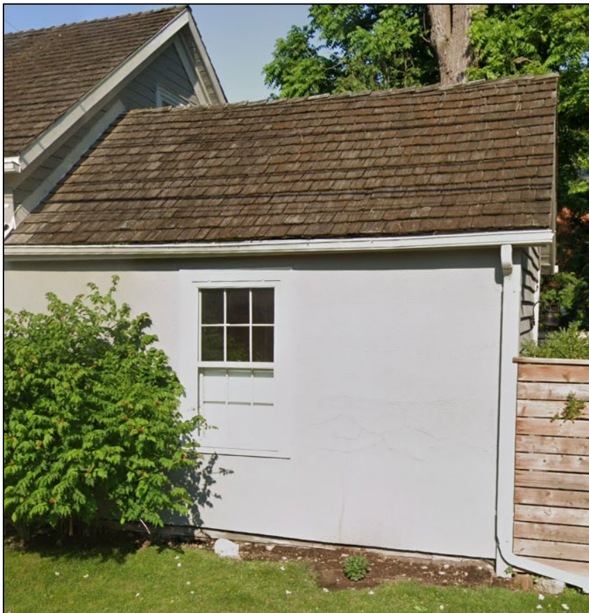
Figure 3: West elevation, back portion of roof to be replaced
