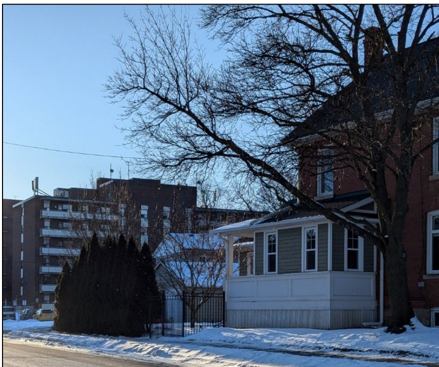
Figure 2: View of the Property and Existing Garage from South corner of the John Street North and Main Street North intersection (c.o. Site Visit, January 14, 2025)
