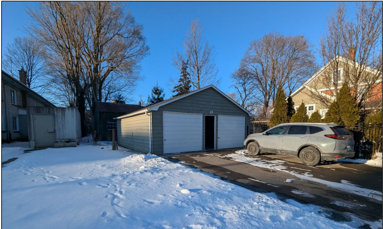
Figure 3: View of the Existing Garage and shed behind as seen from John Street (c.o. Site Visit, January 14, 2025)
