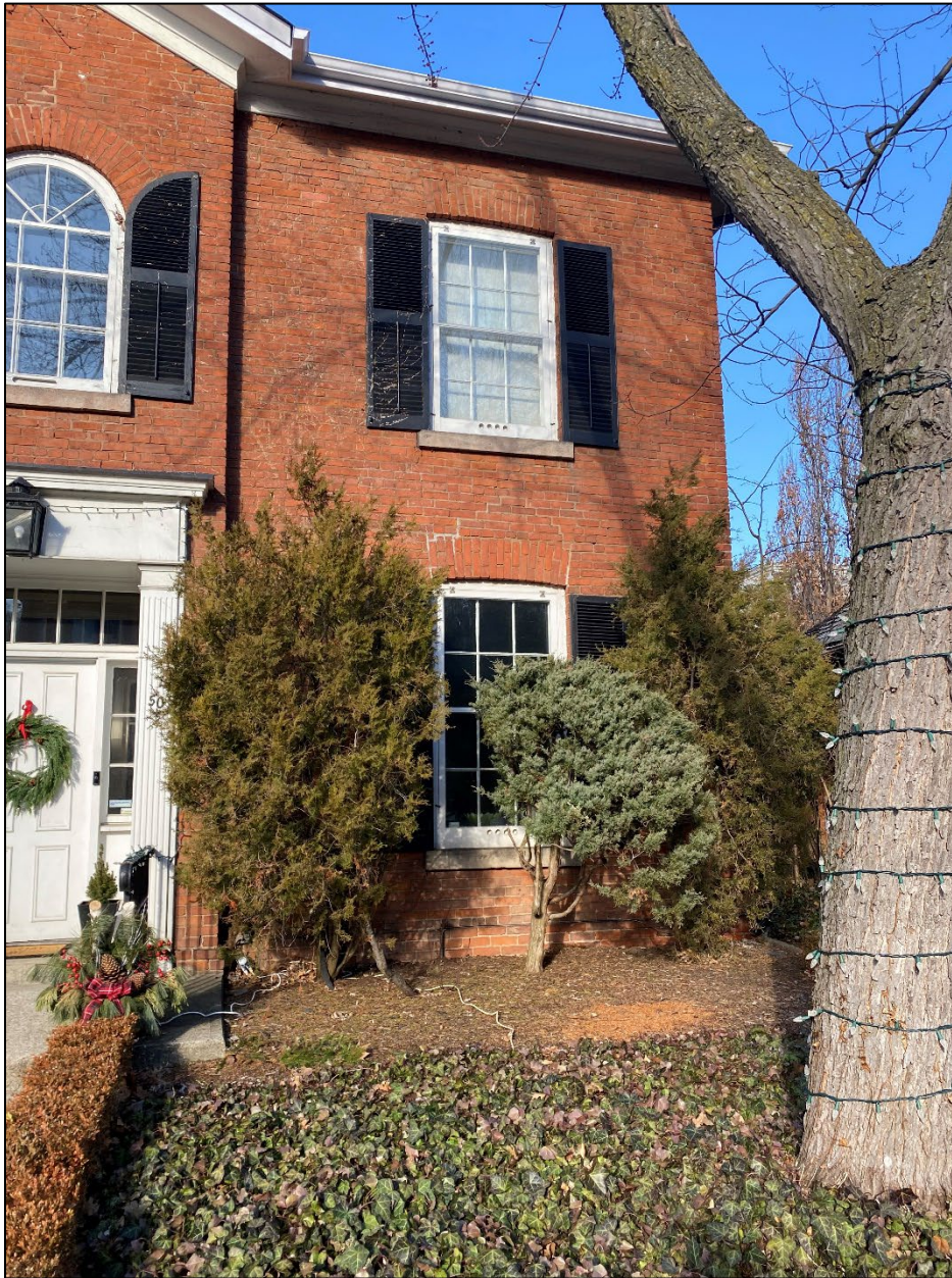
Figure 4: View of the Property from Markland Street (c.o. Site Visit, February 13, 2023)
