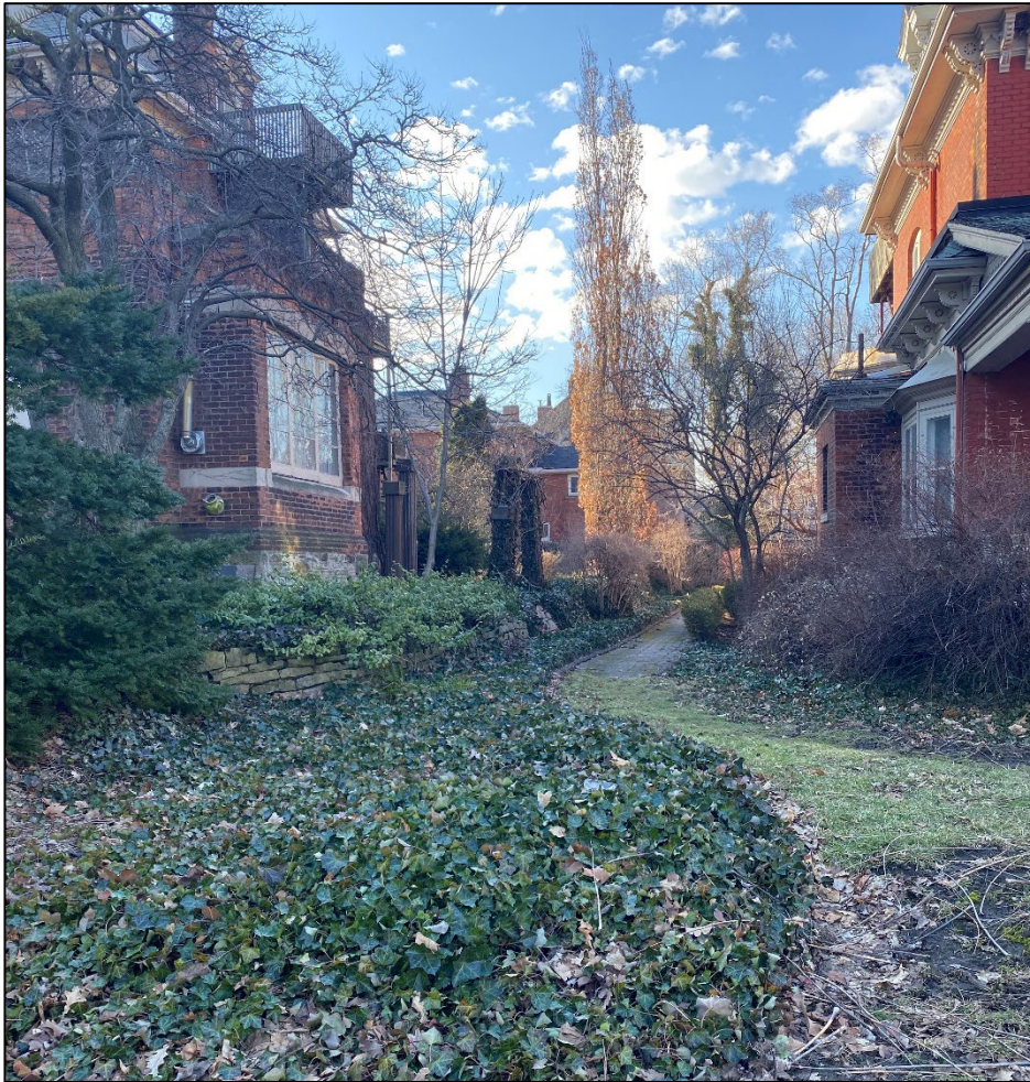
Figure 5: View of the existing rear addition from MacNab Street (c.o. Site Visit, February 13, 2023)
