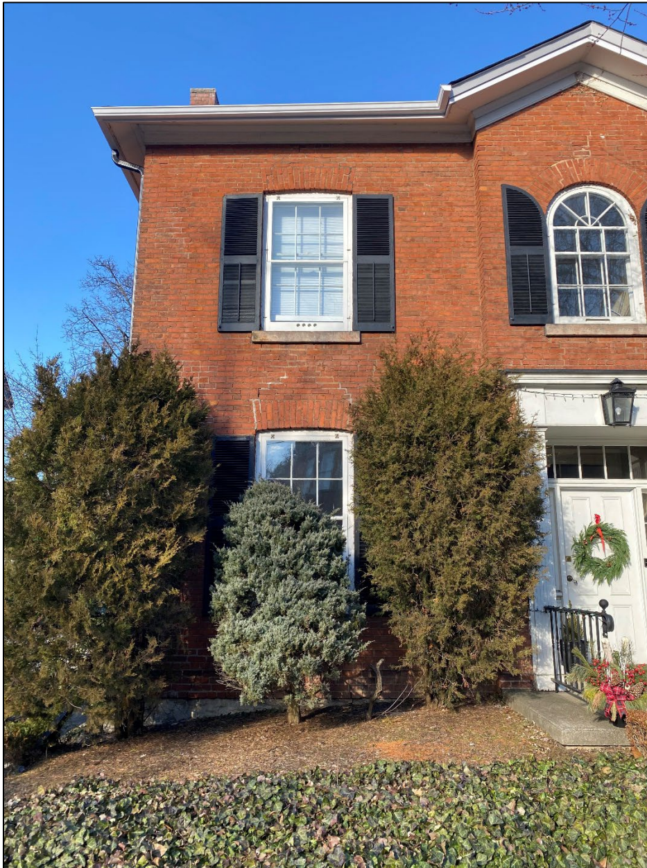
Figure 3: View of the Property from Markland Street (c.o. Site Visit, February 13, 2023)
