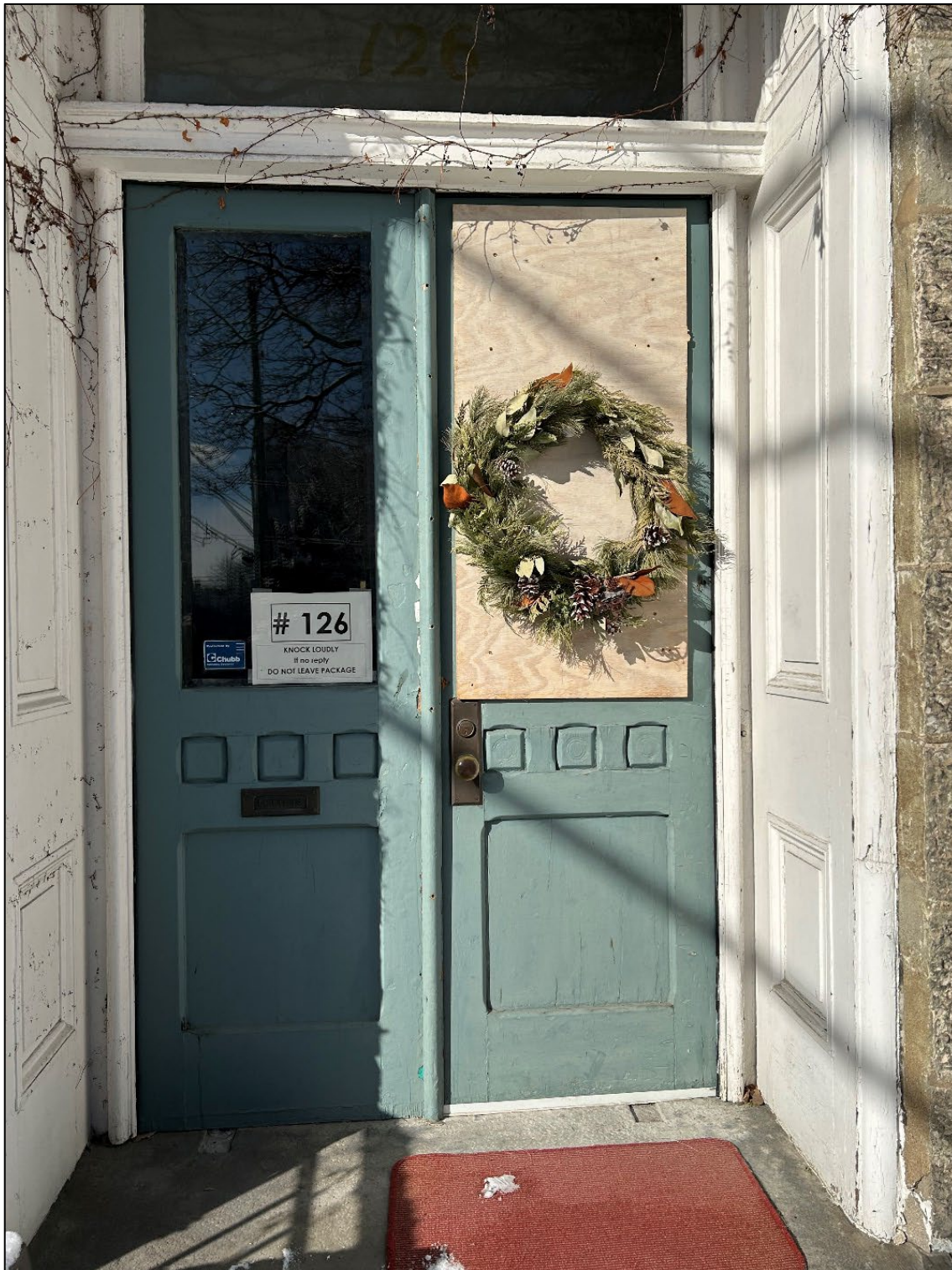
Figure 3: View of the front entry's existing condition.
