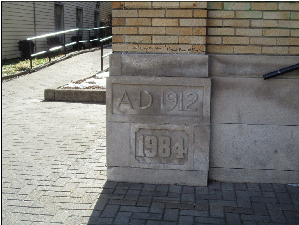
Figure 10: Detail view of date stones.
