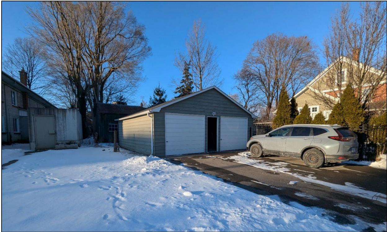
Figure 1: View of the Existing Garage and shed behind as seen from John Street (c.o. Site Visit, January 14, 2025)
