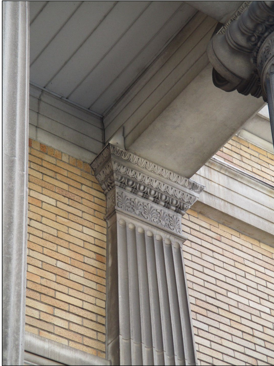
Figure 7: Detail view of pilaster.
