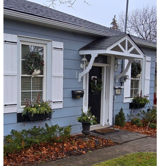
Front entry roof covering (Owner, 2024)
