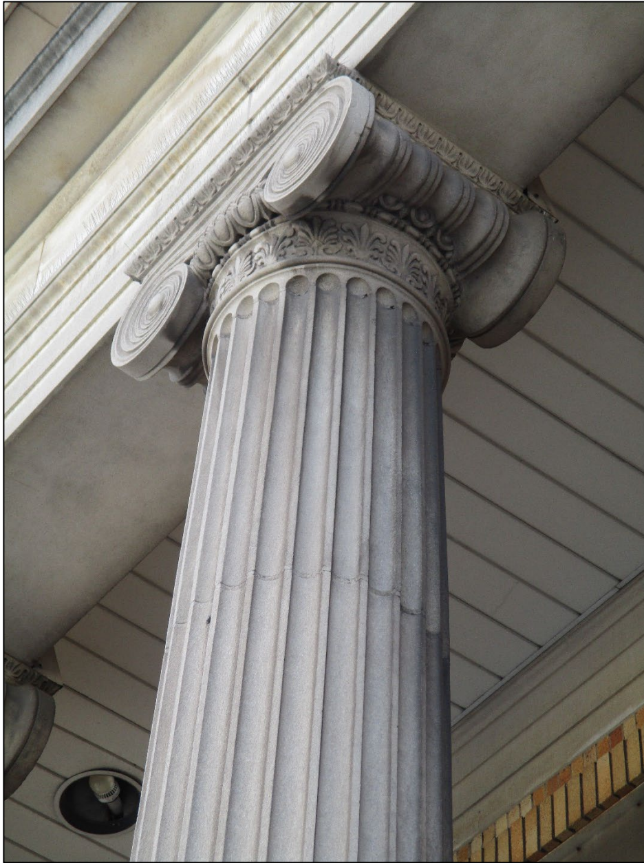
Figure 8: Detail view of Ionic capital.
