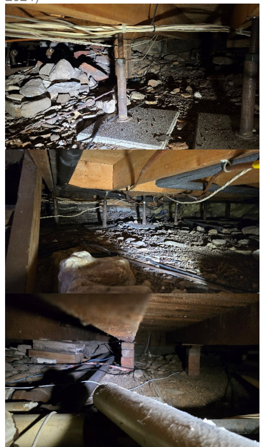
Basement & crawl space (Owner, 2024)
