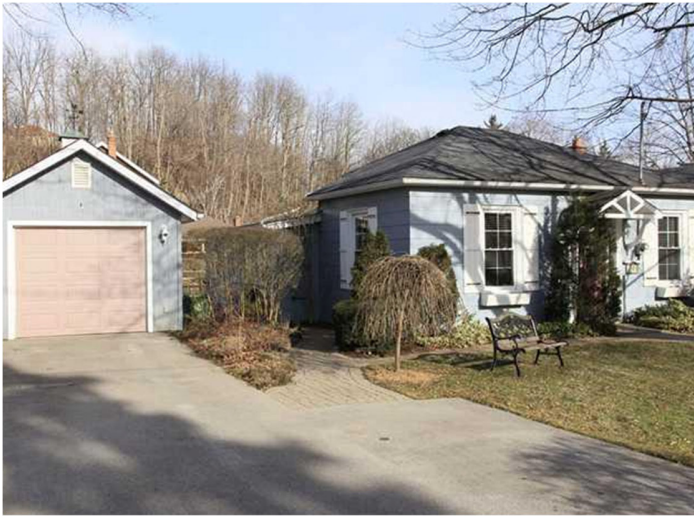
North/East exterior front elevation including detached accessory building (photo, 2013)
