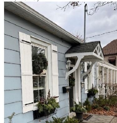
Front elevation covered roof at entry (Park Eight, 2024)
