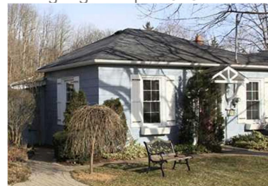
North/East exterior front elevation (photo, 2013)
