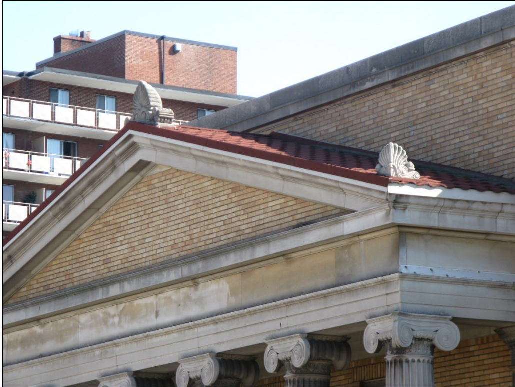
Figure 9: Detail view of pediment and acroterion. City of Hamilton staff, September 2011.
