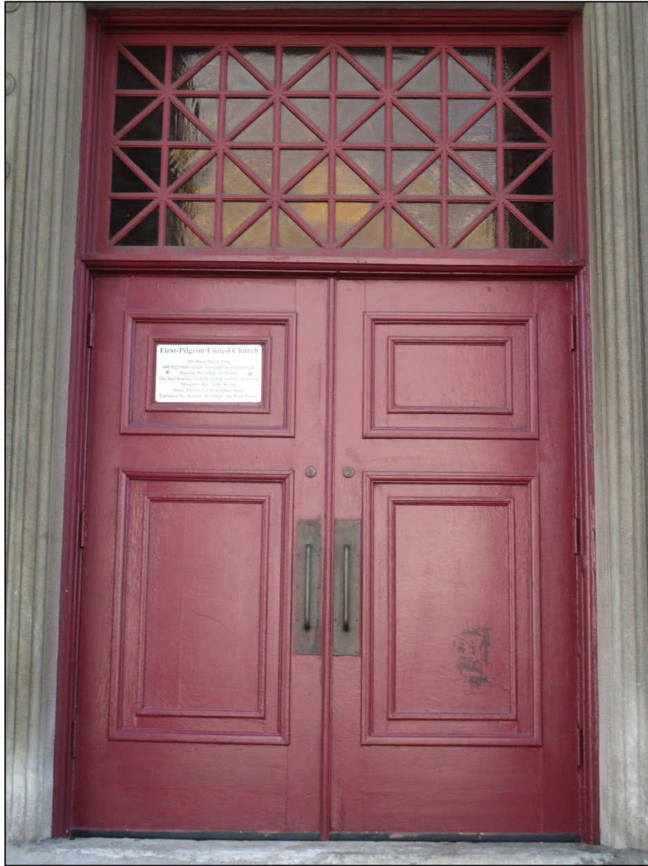
Figure 4: Detail view of doorway.
