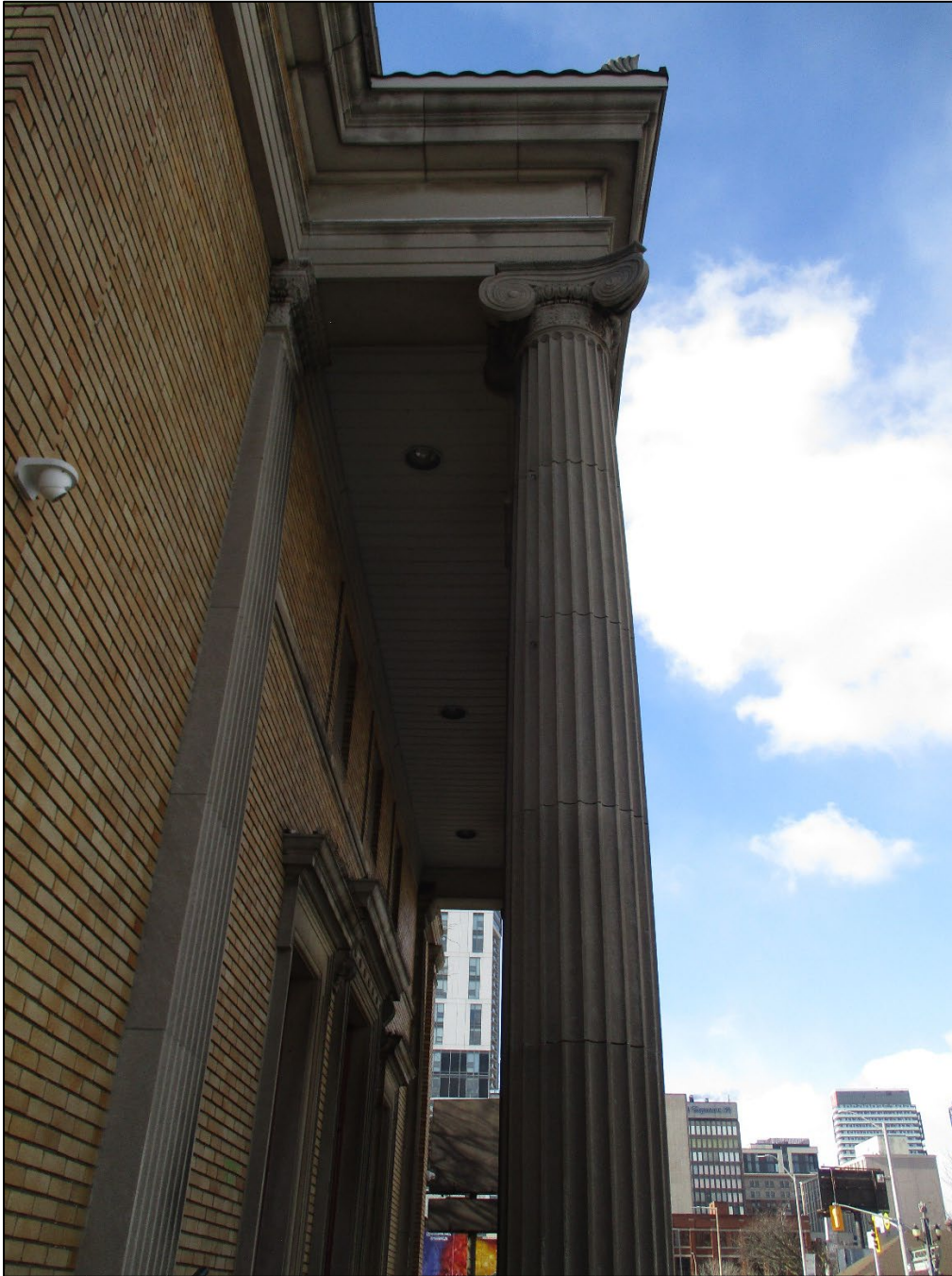
Figure 2: Detail view of front (north) elevation.
