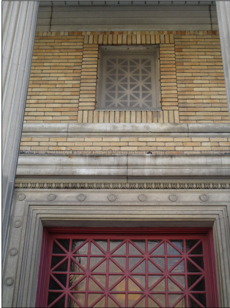
Figure 5: Detail view of windows.
