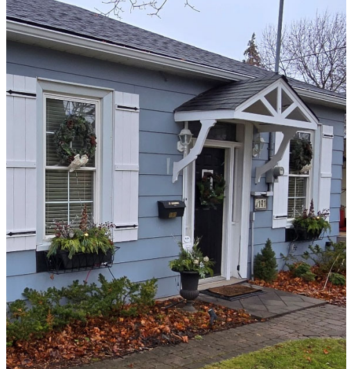
Front entry roof covering (Owner, 2024)
