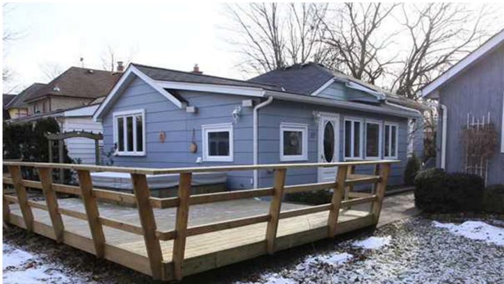
South/East exterior elevation (2013)
