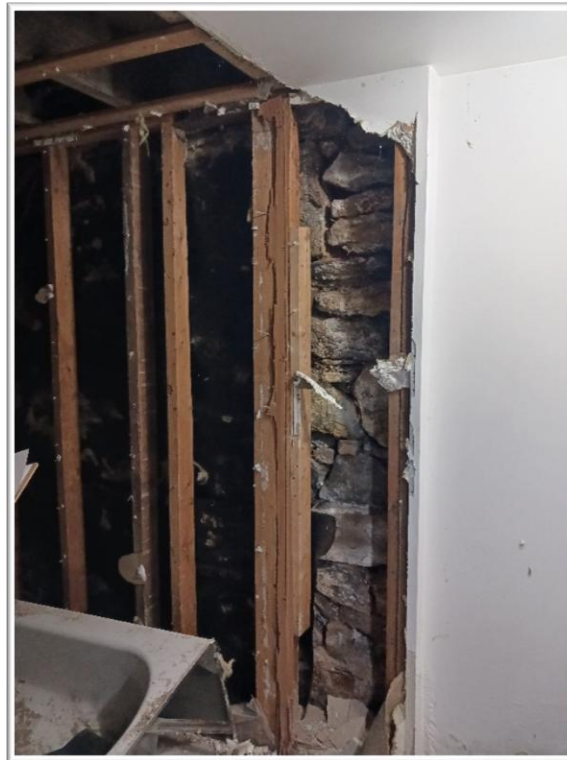
Figure 3: Damaged Foundation wall
