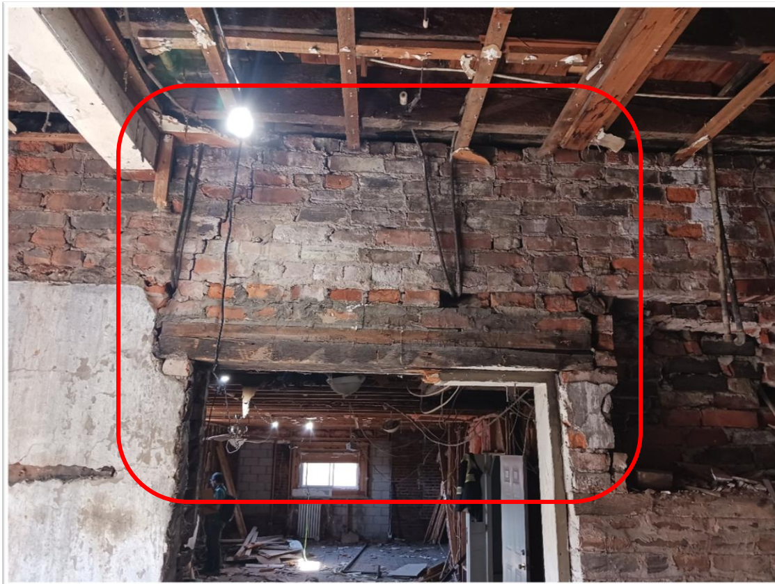
Figure 12: Deflected Lintel with Compromised Supports and Cracked Masonry Wall
