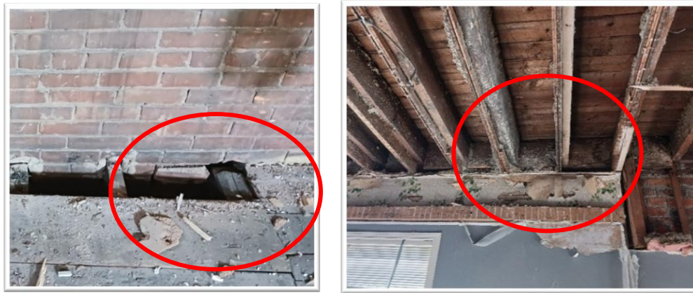
Figure 8: Inadequate Joist Bearing on Load-Bearing Wall
