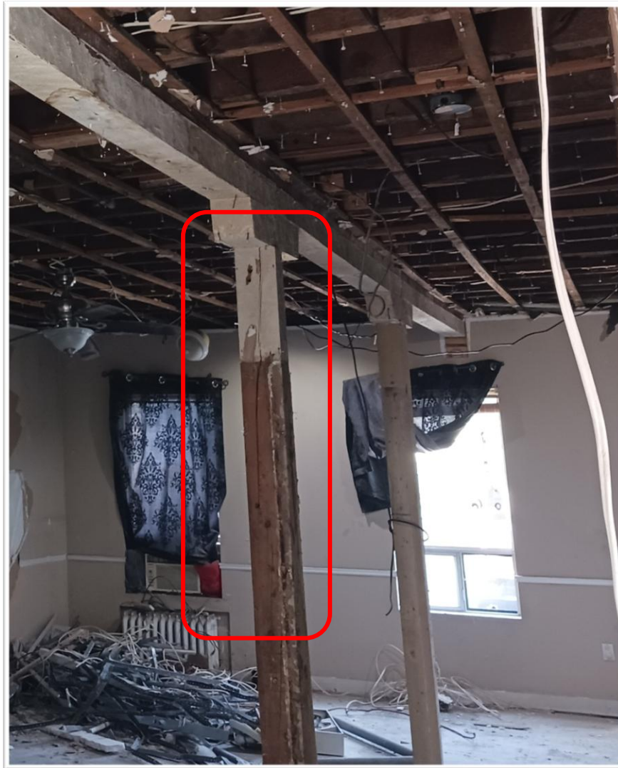
Figure 11: Cracked Structural Column
