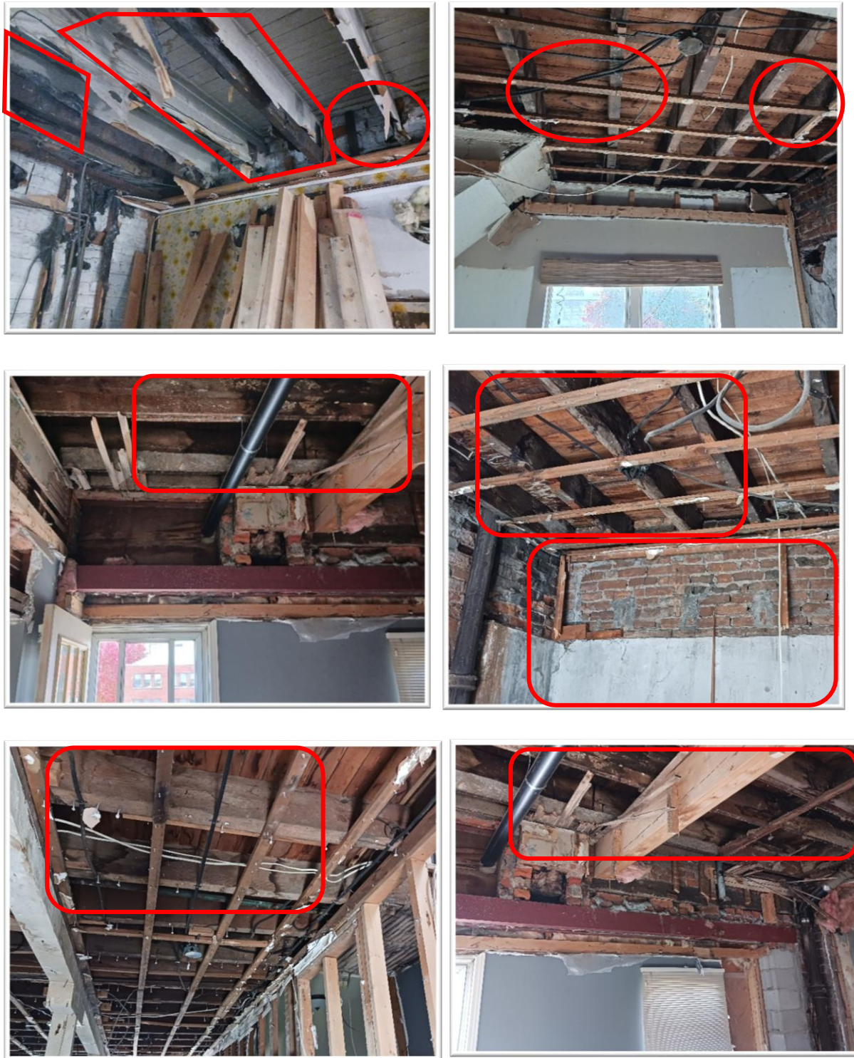
Figure 9: Joist deterioration due to water infiltration and load bearing wall cracks
