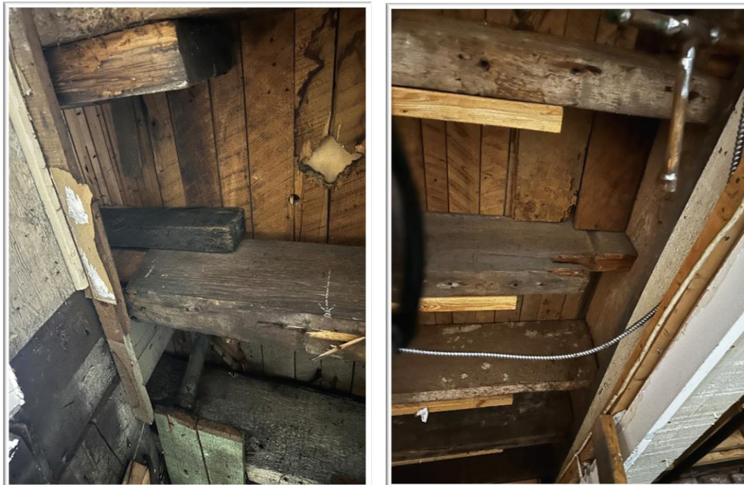
Figure 4: Inadequate Joist Bearing
