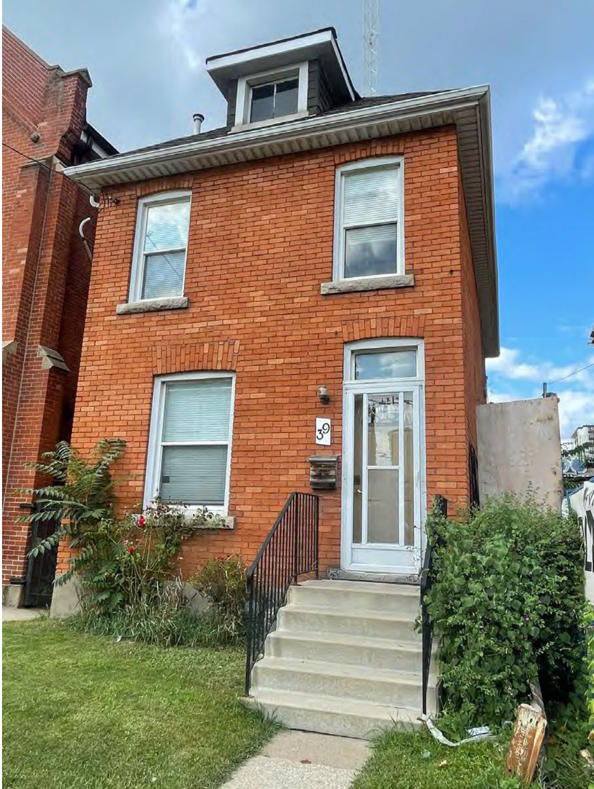
1902 Caretakers House, 39 Wilson Street – brick veneer – windows and doors have brick arches and cut stone sills – doors and windows have been replaced and concrete stairs have been installed at the front entrance on Wilson Street – foundation is parged
