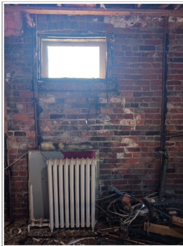
Figure 7: Crack on Exterior Load Bearing Wall and Lintel
