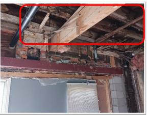
Figure 9: Joist deterioration due to water infiltration and load bearing wall cracks
