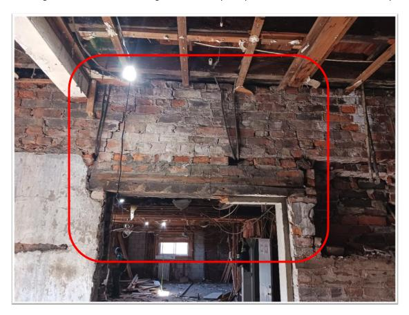
Figure 12:Deflected Lintel with Compromised Supports and Cracked Masonry Wall
