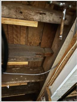
Figure 4: Inadequate Joist Bearing
