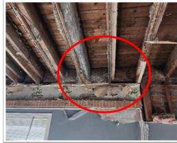
Figure 8: Inadequate Joist Bearing on Load-Bearing Wall
