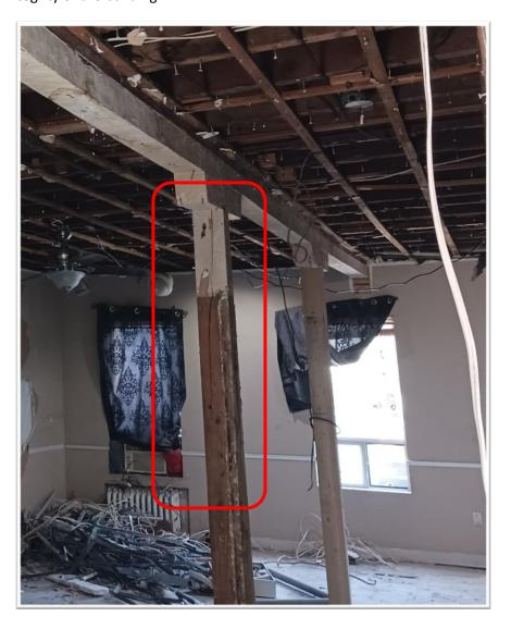
Figure 11: Cracked Structural Column
