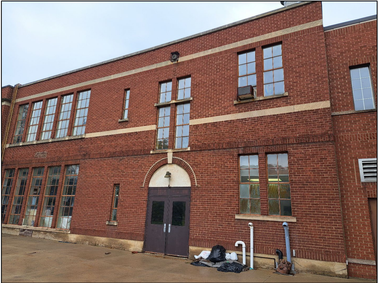
Figure 4: South elevation of the former Princess Elizabeth School, (City files).
