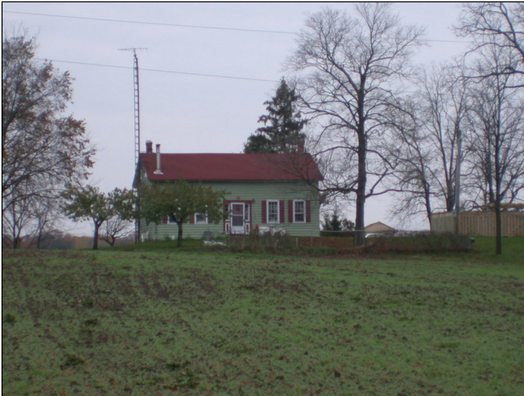
Figure 6: South elevation of designated structure on the property (circa 2002, city files)
