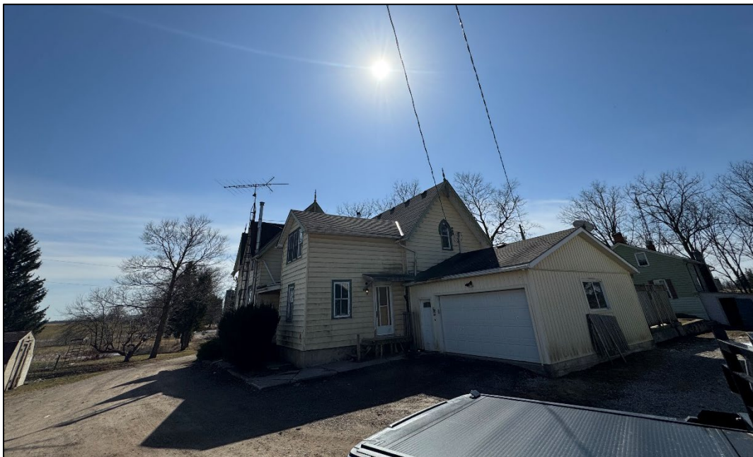
Figure 5: North elevation of house proposed for demolition (Submitted by consultant)
