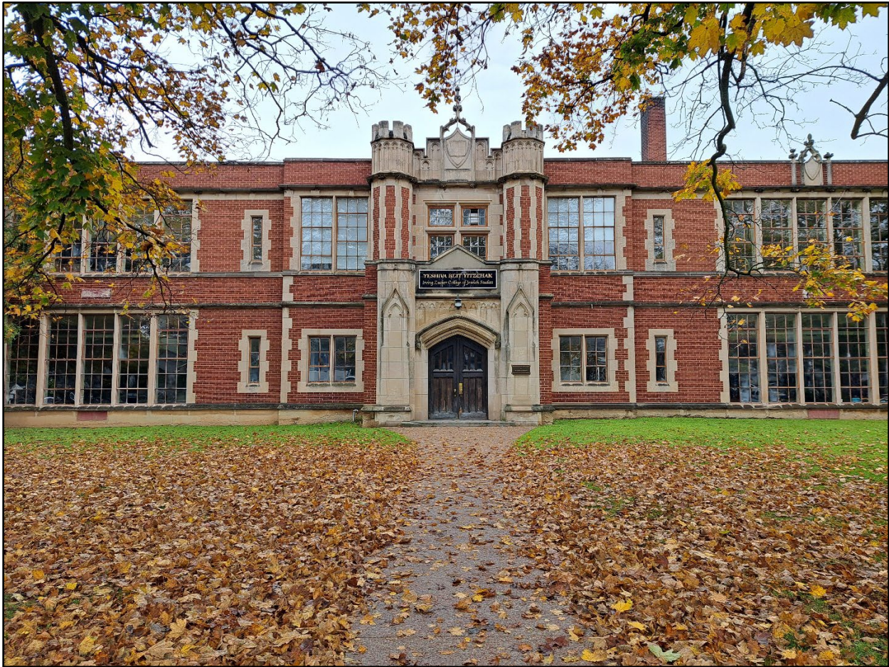
Figure 1: Image of the front elevation of the former Princess Elizabeth School, (City files).
