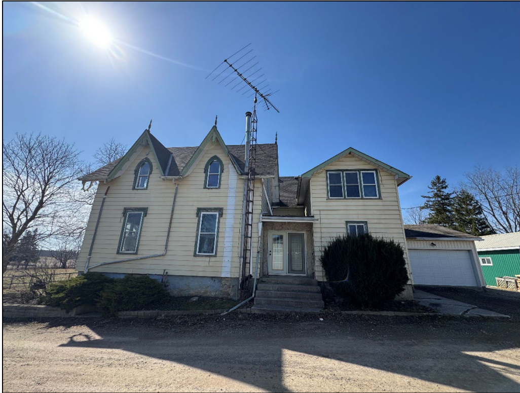
Figure 4: East elevation of house proposed for demolition (Submitted by consultant)
