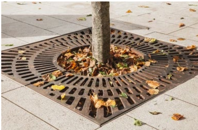
Figure 7: Tree grate with large inner ring and square outer perimeter.
