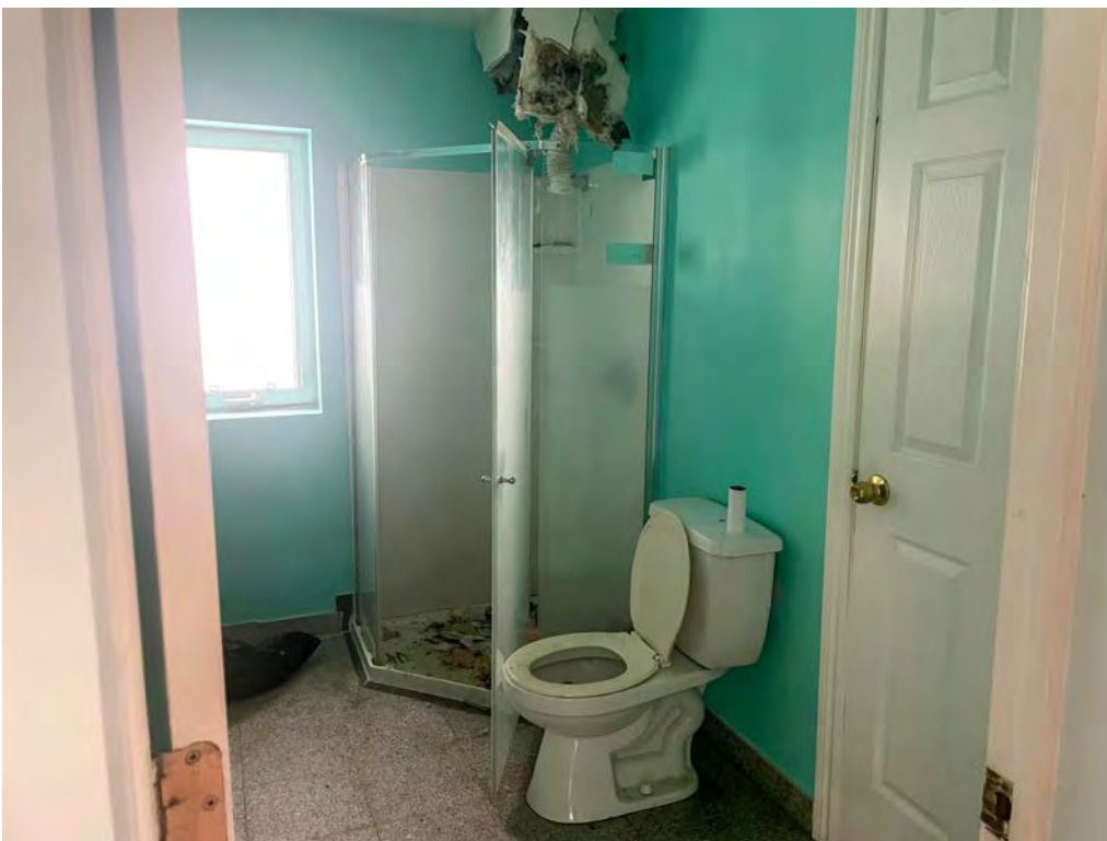
Interior – 1 st floor bathroom – a portion of the ceiling has collapsed - modern finishes – no historic features or finishes
