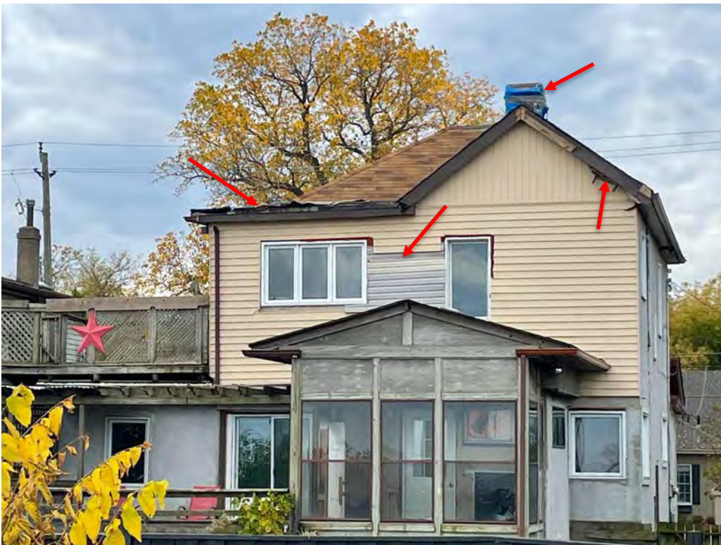
REAR ELEVATION – roof is in very poor condition – shingles lifting and tarp on chimney – rotted soffit & fascia boards – poorly fitted replacement windows – patched siding
