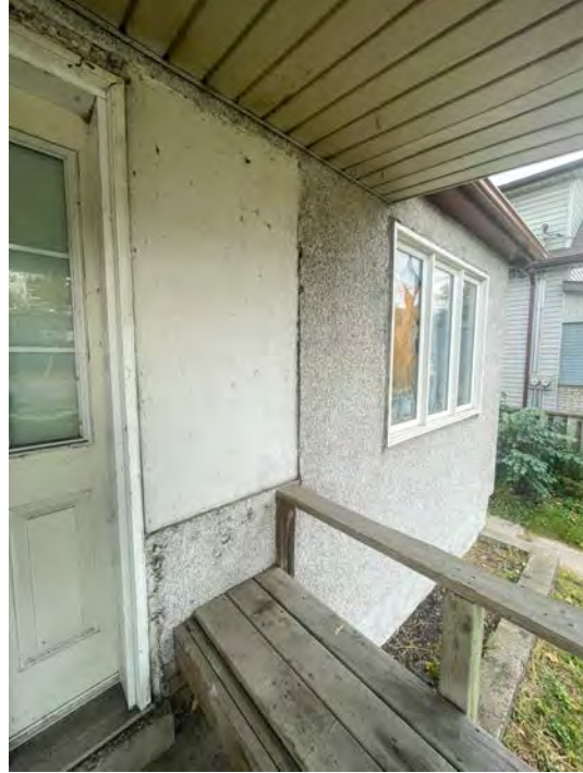
Boarded up openings – vinyl replacement doors and windows – locations and sizes of windows have been changed
