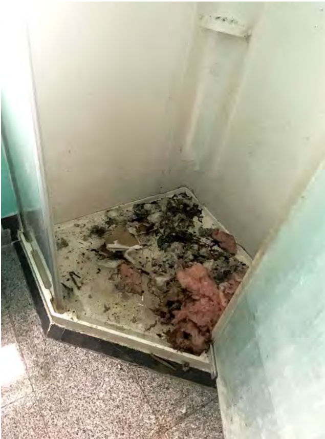
Interior – 1 st floor bathroom – wet insulation and drywall debris where a portion of the ceiling has collapses
