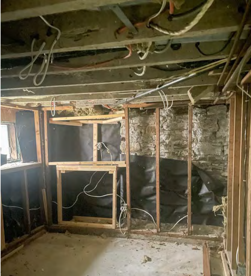
Basement – waterproof membrane installed in some areas of the basement to address damp issues
