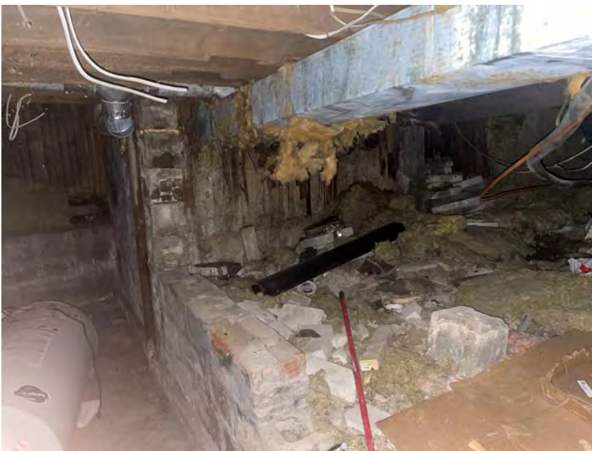
Basement – modern ducting installed through older foundation and wood joists – insulation debris and damp conditions
