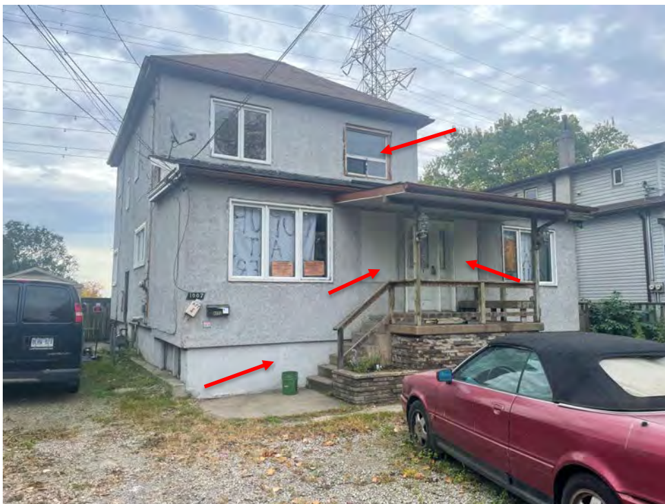
Front entrance – cracks visible in the poured foundation – original openings boarded up – mis-matched replacement windows
