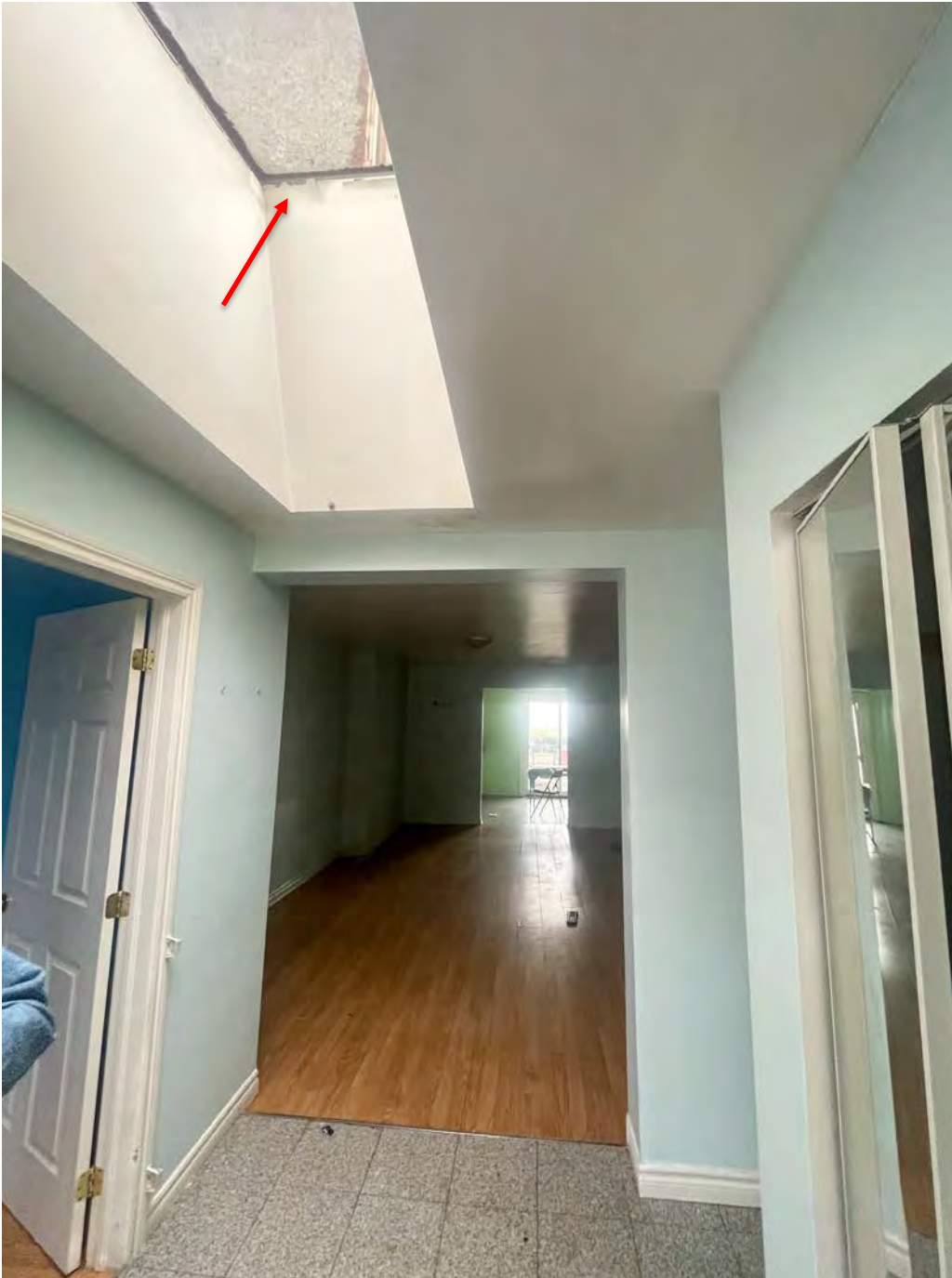
INTERIOR – modern skylight in entrance hall is leaking – modern finishes – no historic features or finishes
