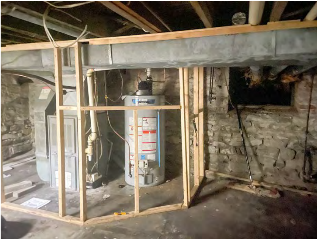
Basement – rubblestone – remnants of a late-19 th or early 20 th century foundation
