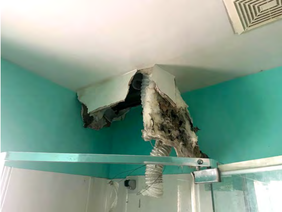
Interior – 1 st floor bathroom – water damage
