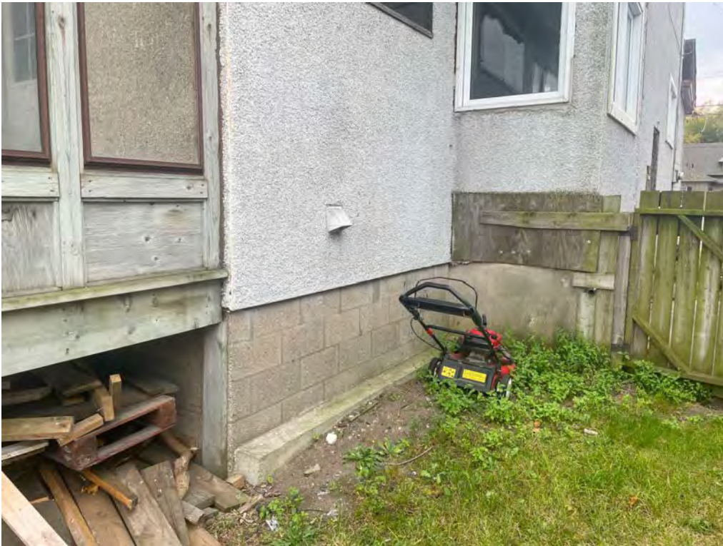
REAR ADDITION – concrete block foundation – cement parging above
