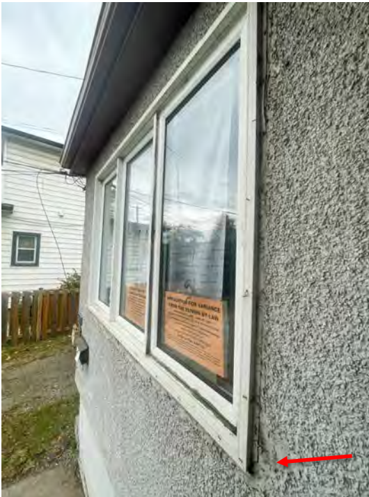
Poorly installed vinyl replacement windows – modern cement parging with patching and gaps around window openings
