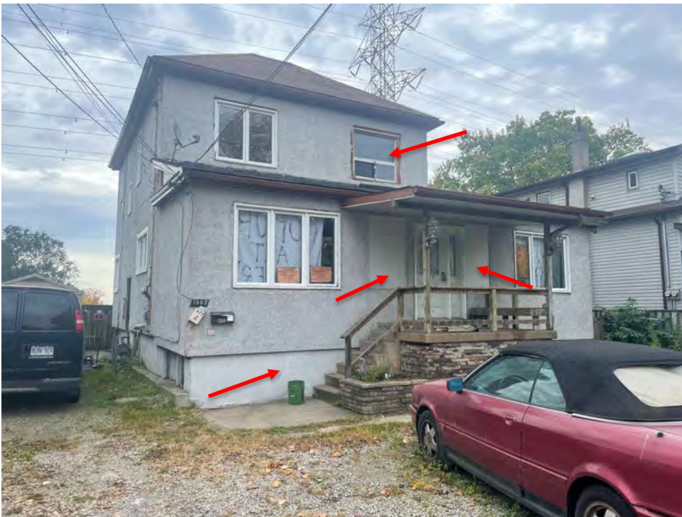
Front entrance – cracks visible in the parged foundation – original openings boarded up – mis-matched replacement windows
