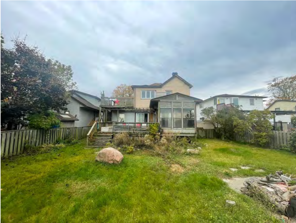
Rear elevation – replacement vinyl doors and windows – vinyl cladding on 2 nd floor – poorly constructed enclosed porch and decks – poorly installed replacement vinyl windows
