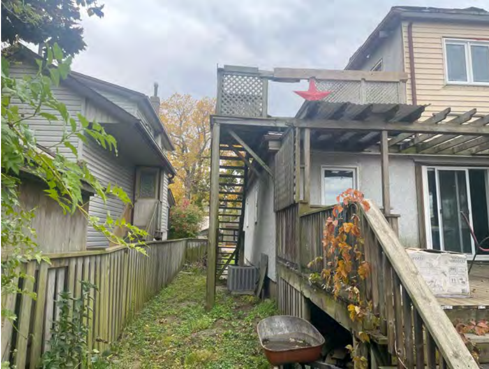
South side yard – poorly constructed deck and exit stair
