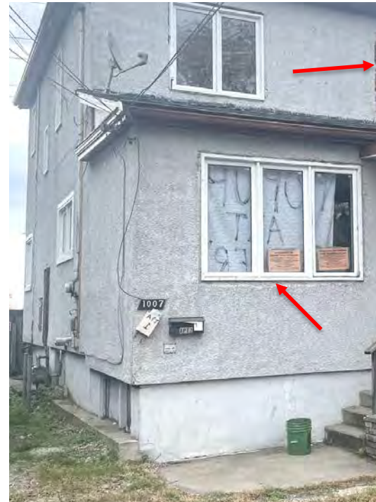
Poorly installed vinyl replacement windows – modern cement parging with patching and gaps around window openings
