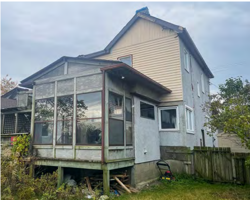
Rear and north side elevation – mish-mash of materials – poorly installed replacement vinyl windows
