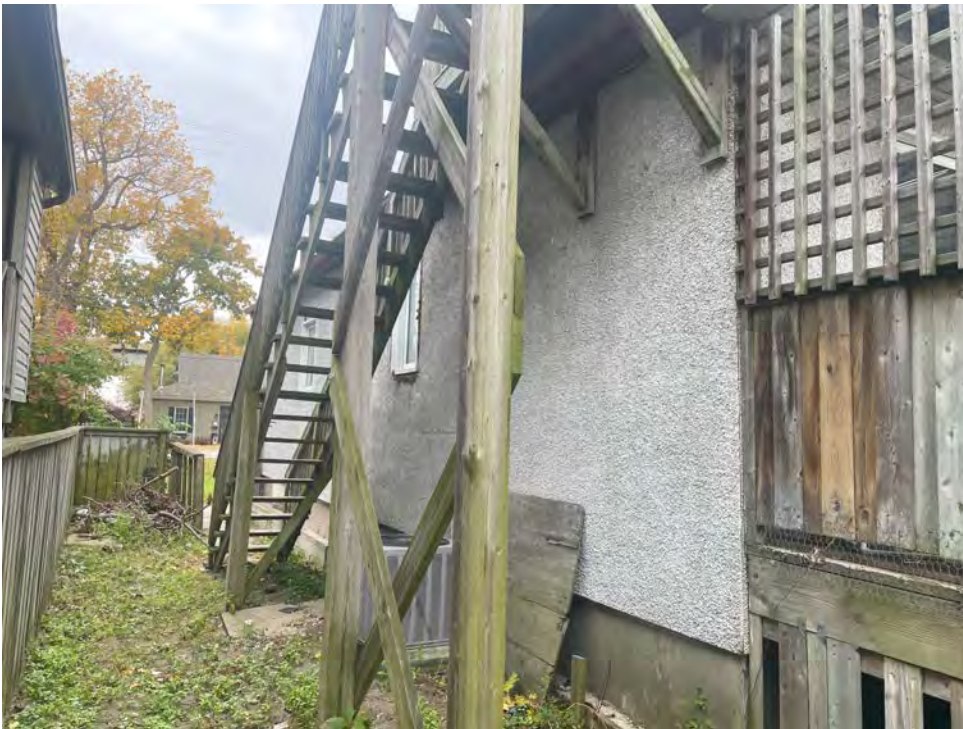
SIDE ELEVATION - parge foundation with cement stucco above – wood fire escape attached to stucco
