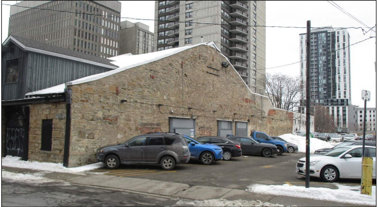
Figure 3: Side (south) elevation of subject property.
