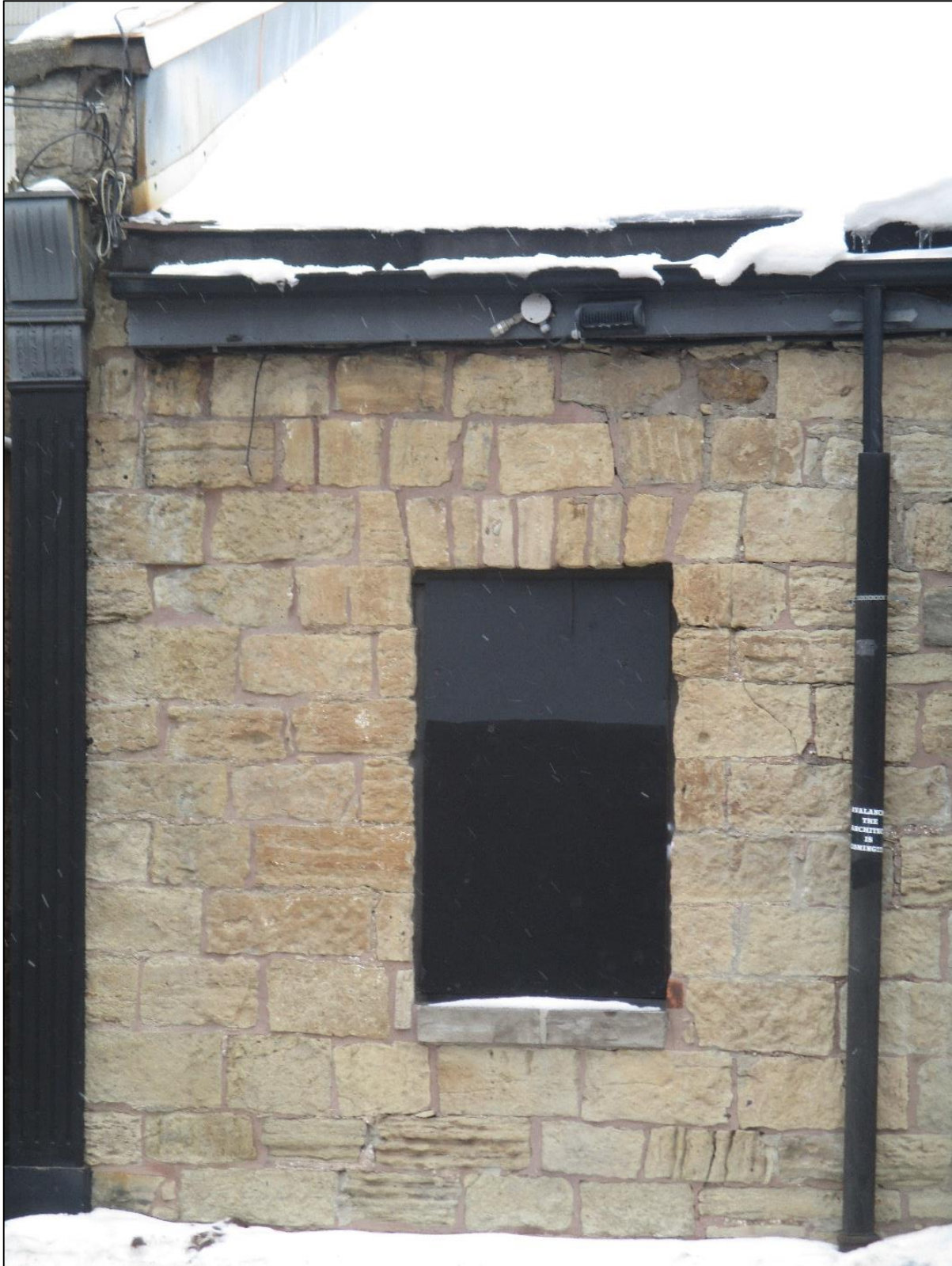
Figure 2: Detail view of window opening on front elevation.
