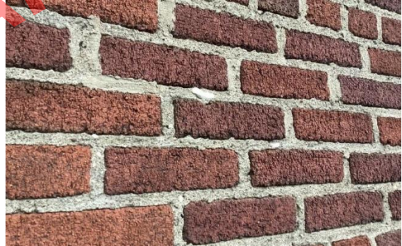
Figure 3: Typical masonry mortar profile overview.
