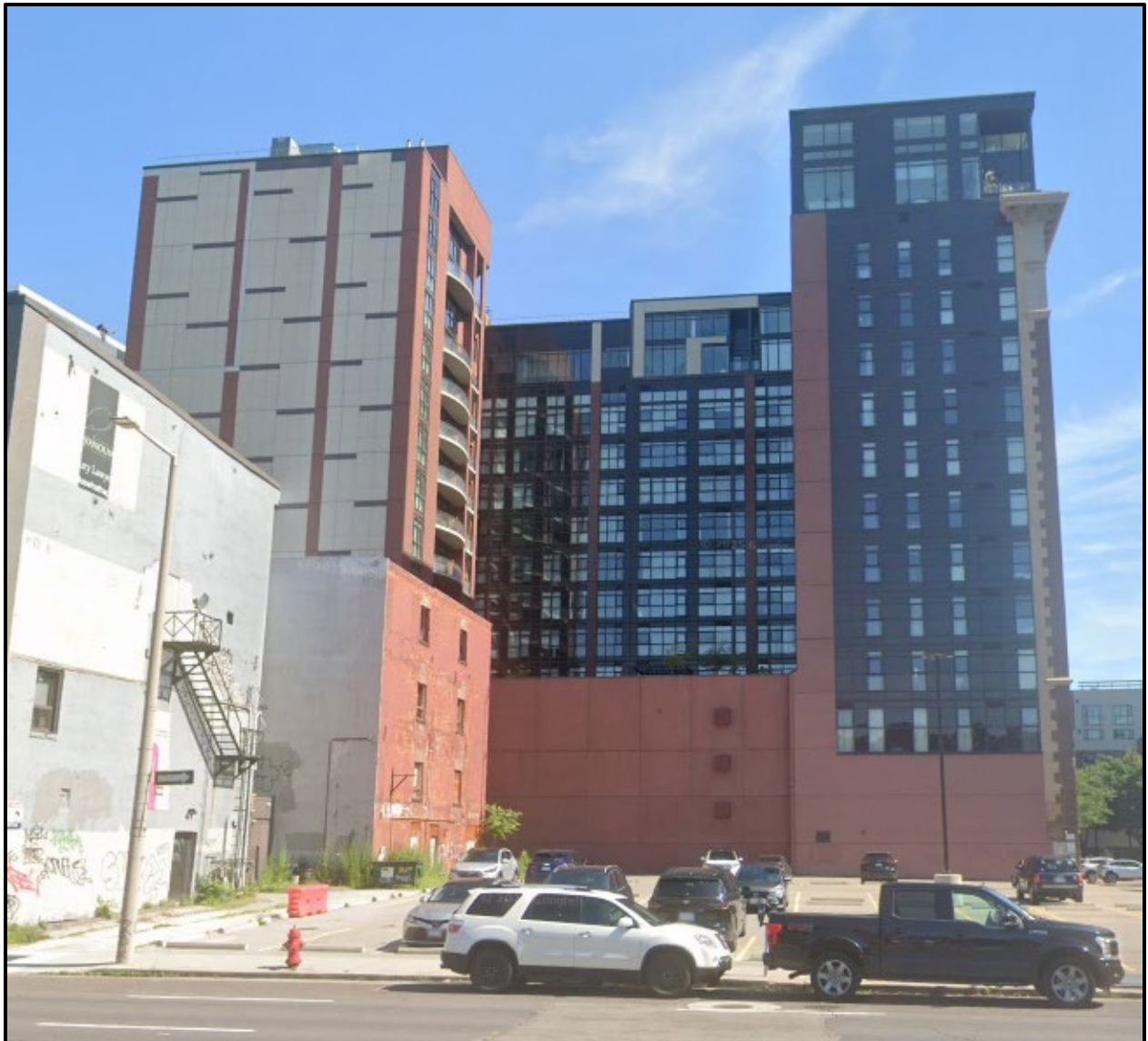
Figure 3: Rear (south) elevation of the Royal Connaught looking north past Main Street East(Google Earth, 2024)
