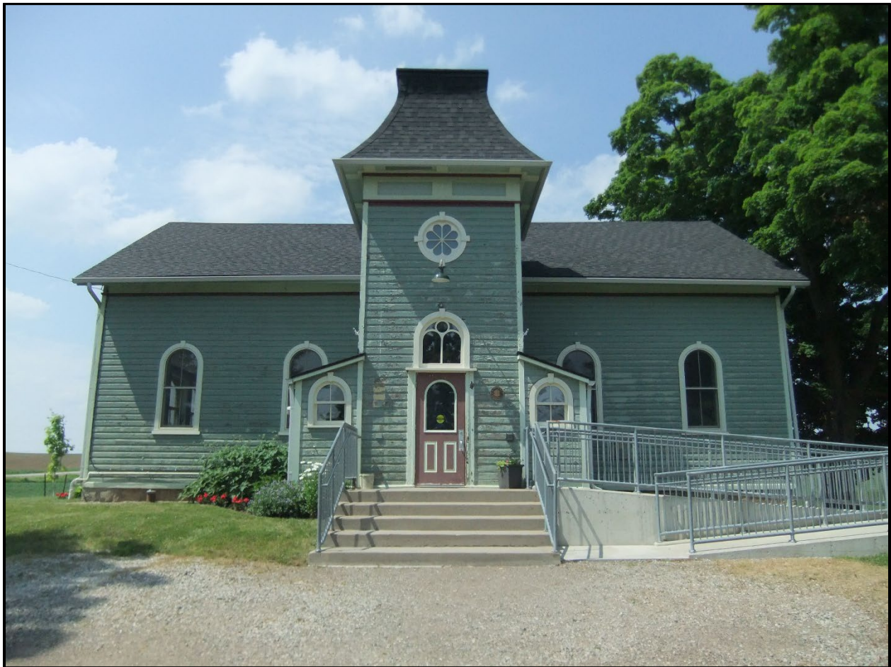
Figure 1: Front (south) elevation of 2295 Troy Road showing the central front tower, accessible entrance and steps (Site Visit, 2024)
