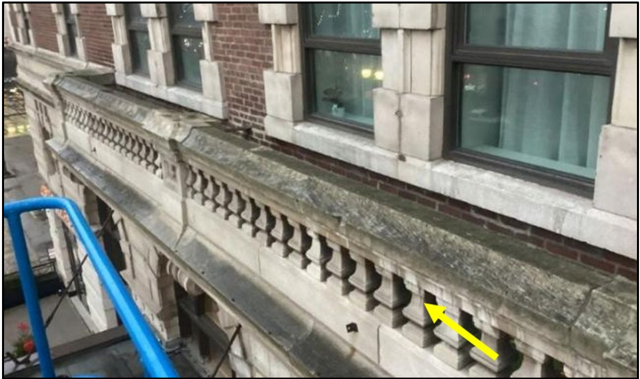
Figure 6: Close up example of cast stone to be cleaned along the north elevation (Proponent Submission, 2026)
