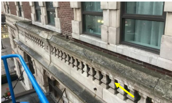
Figure 4: Cast stone cleaning example.
