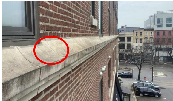
Figure 5: Cast stone crack repair example.
