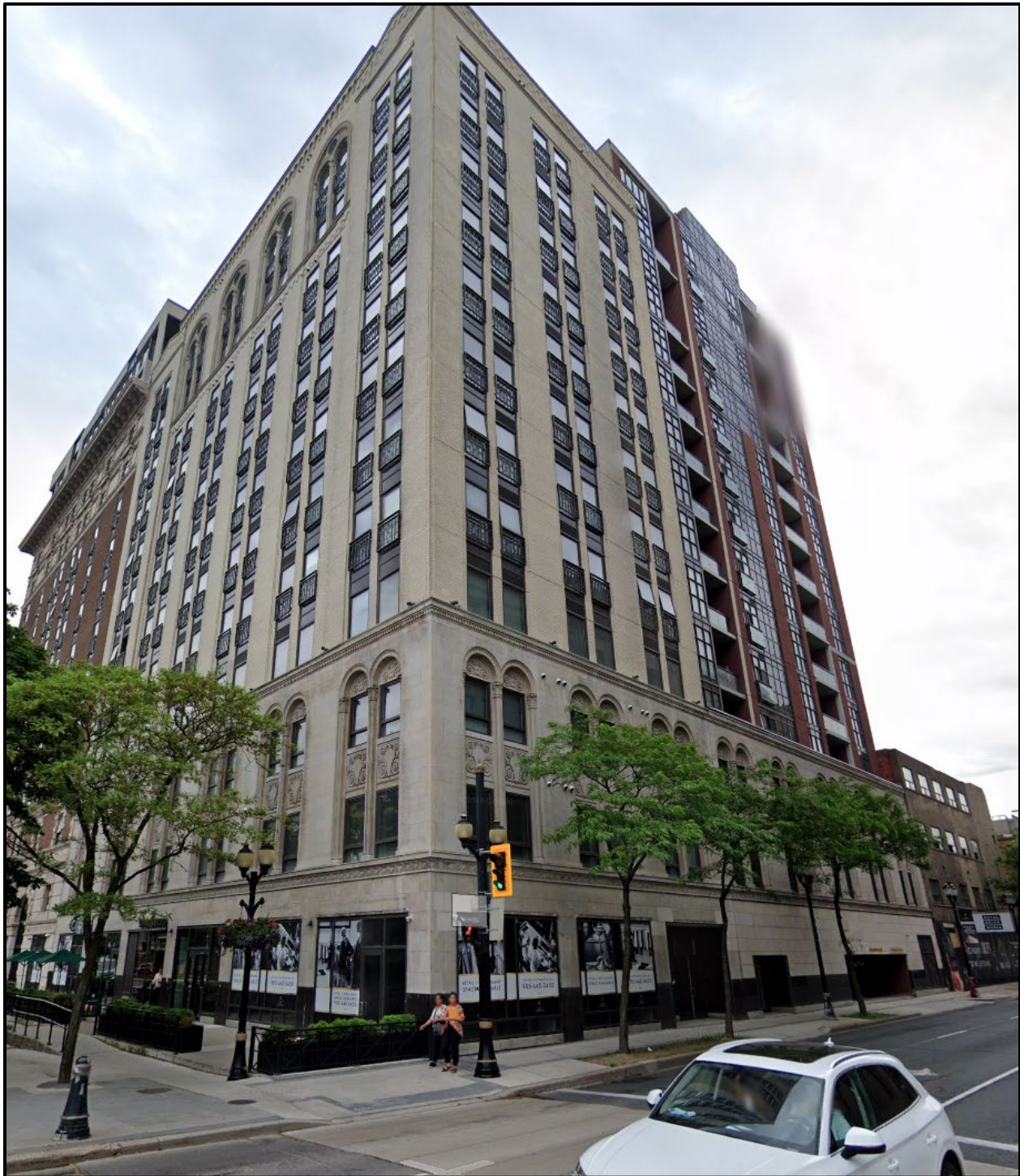
Figure 2: Front (north) and side (west) elevations of the Royal Connaught (Google Earth, 2019)
