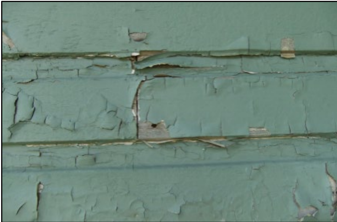
Figure 4: Close up of the deteriorated siding to be replaced, including peeling paint and rotting wood (Site Visit, 2024)
