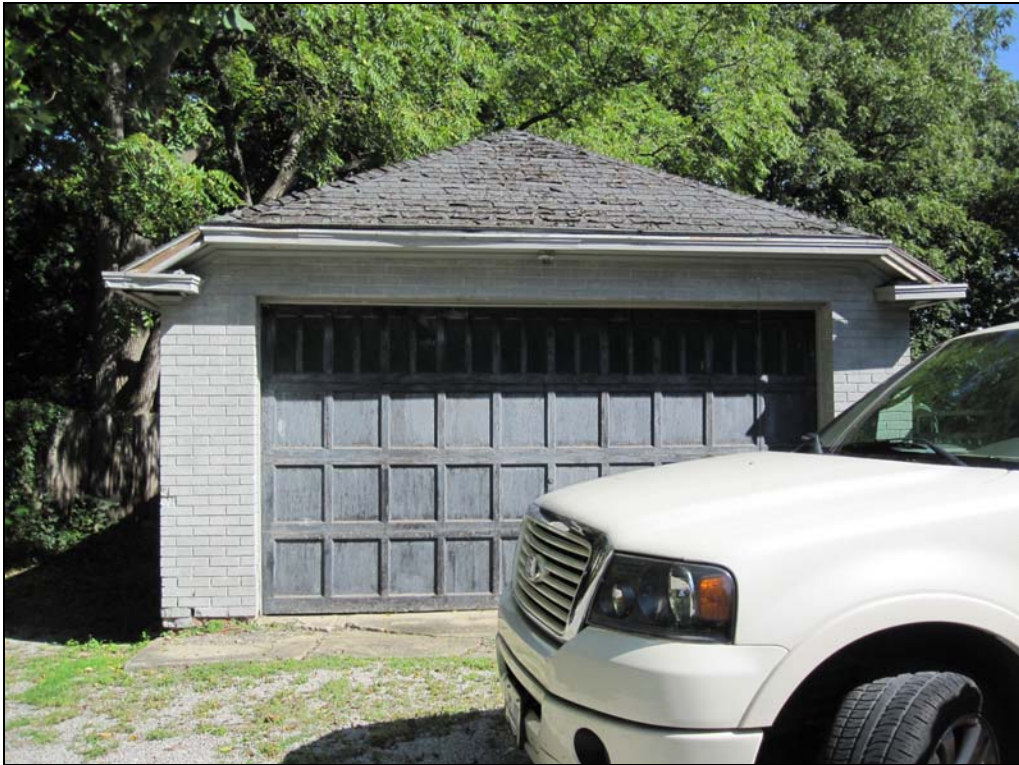
Front elevation of the existing garage (to be demolished)
