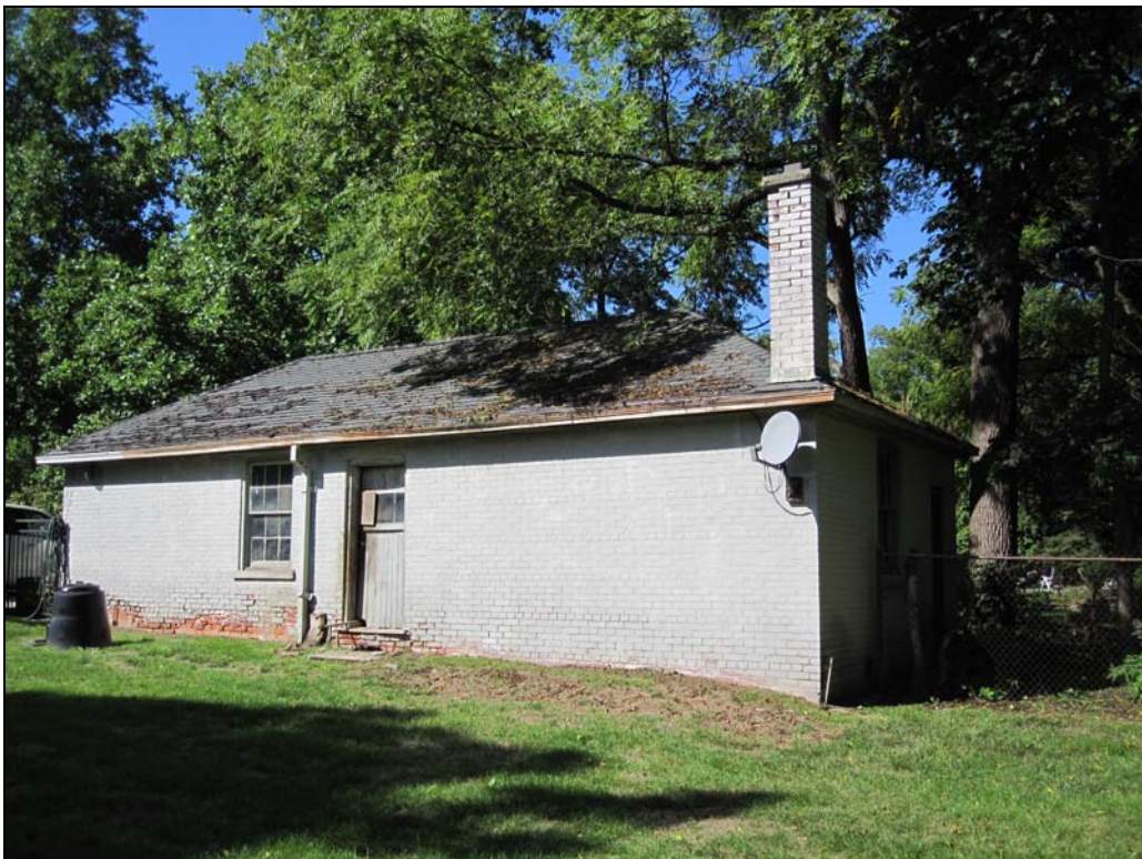
South side elevation of the existing garage (to be demolished)
