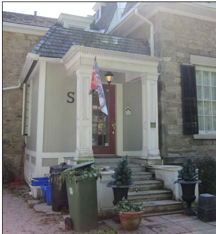
Existing north side entrance (to be removed)
