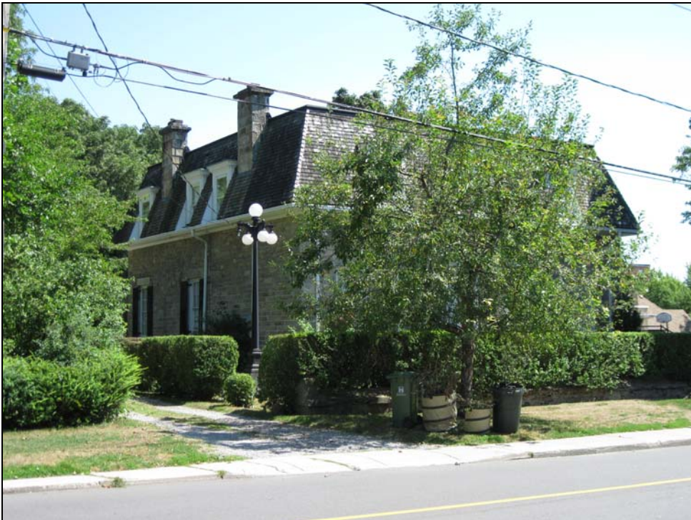
Front and north side elevation of the existing house.
