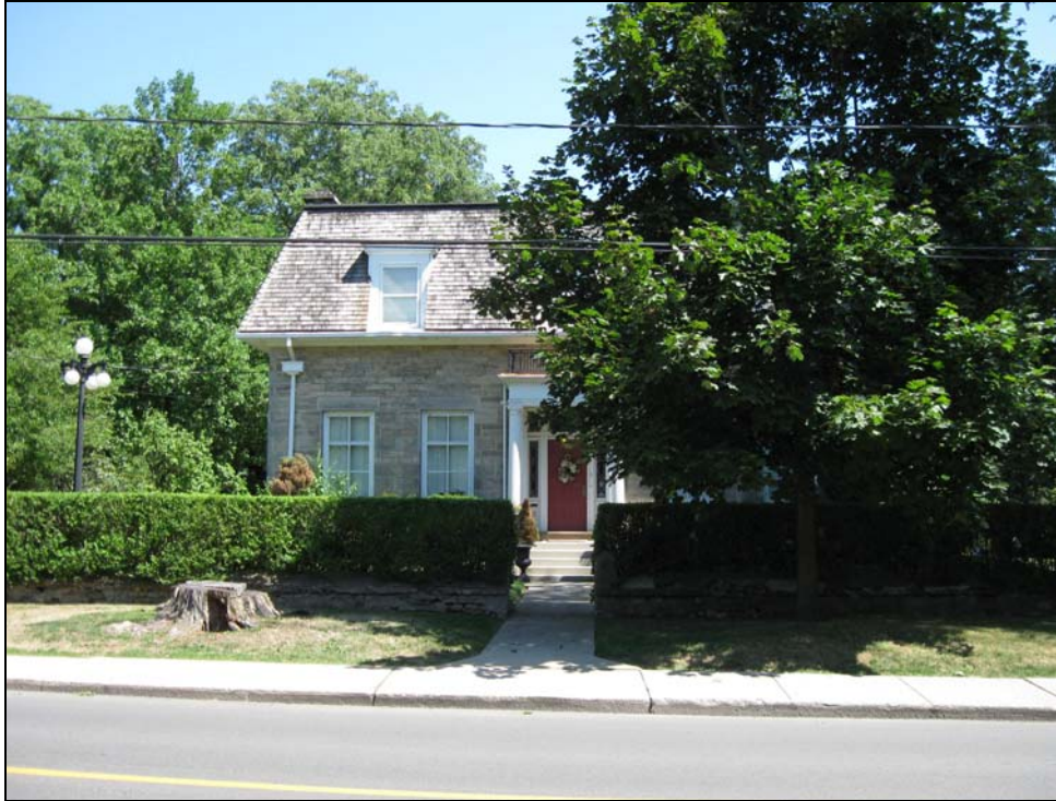
Front façade of the existing house and stone wall.
