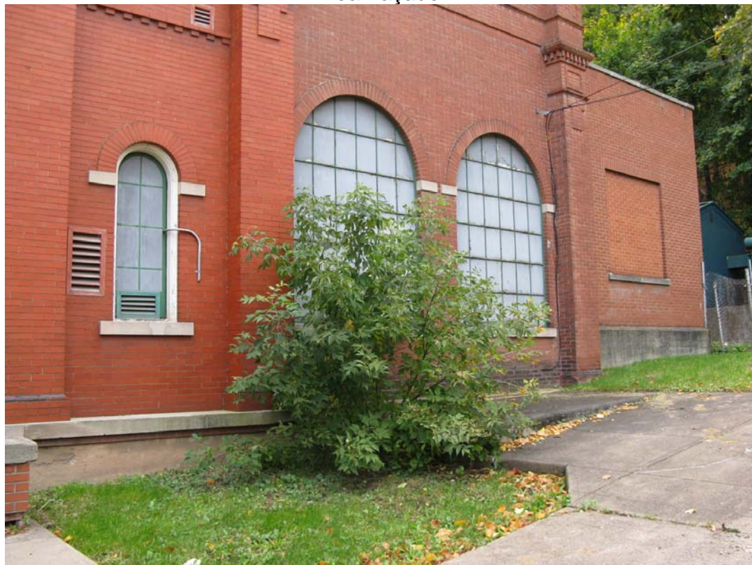
Southerly addition (ca. 1929)
