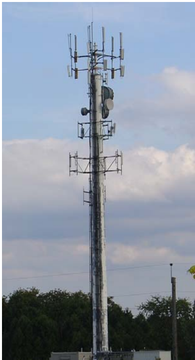
Monopole (Co-location) 18 metres (60 ft) to 45 metres (150 ft)
