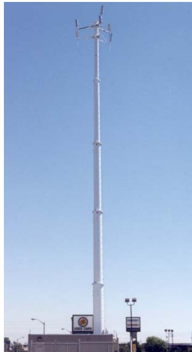
Monopole (Single-Carrier) 18 metres (60 ft) to 45 metres (150 ft)
