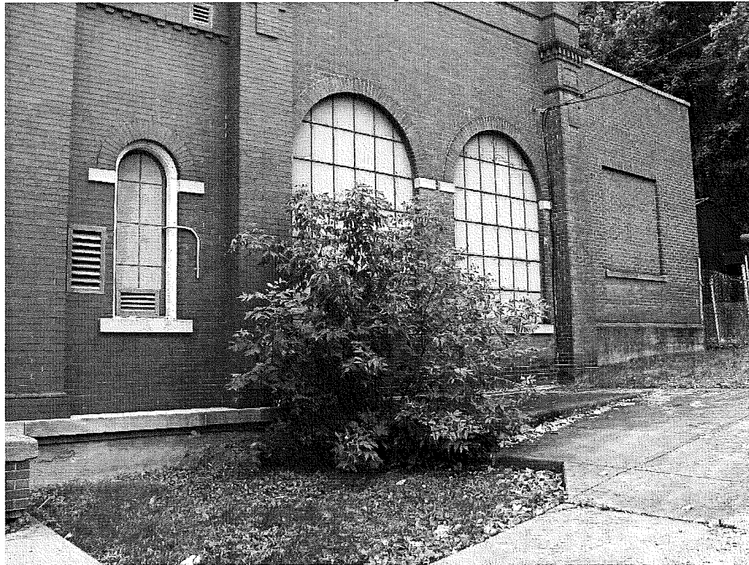
Southerly addition (ca. 1929)
