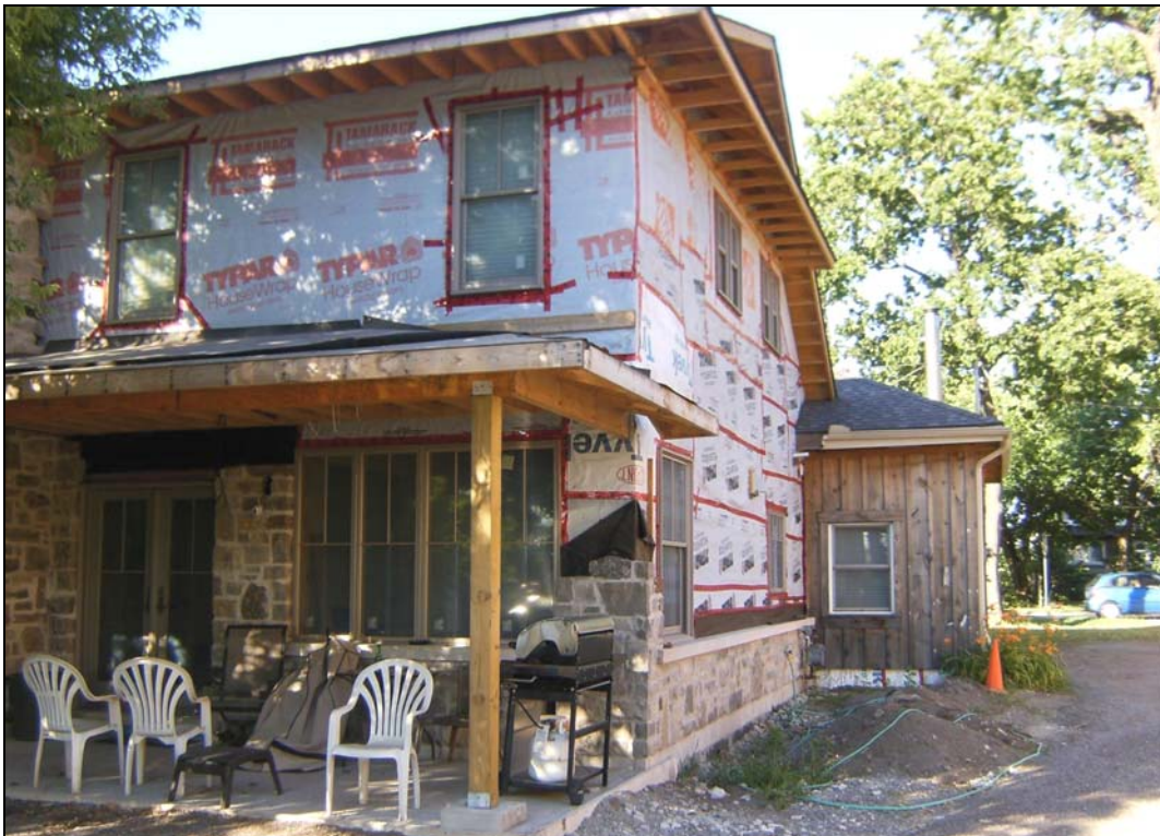
South side and rear of the new addition from the rear
