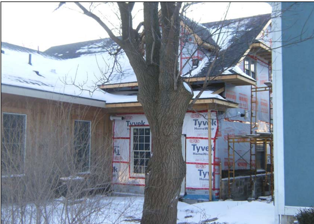
Front and north side of the new addition
