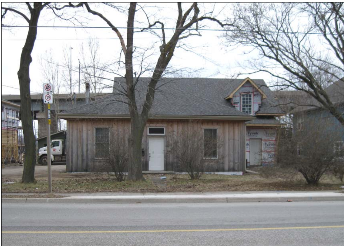
Front façade of the original cottage with the new addition behind
