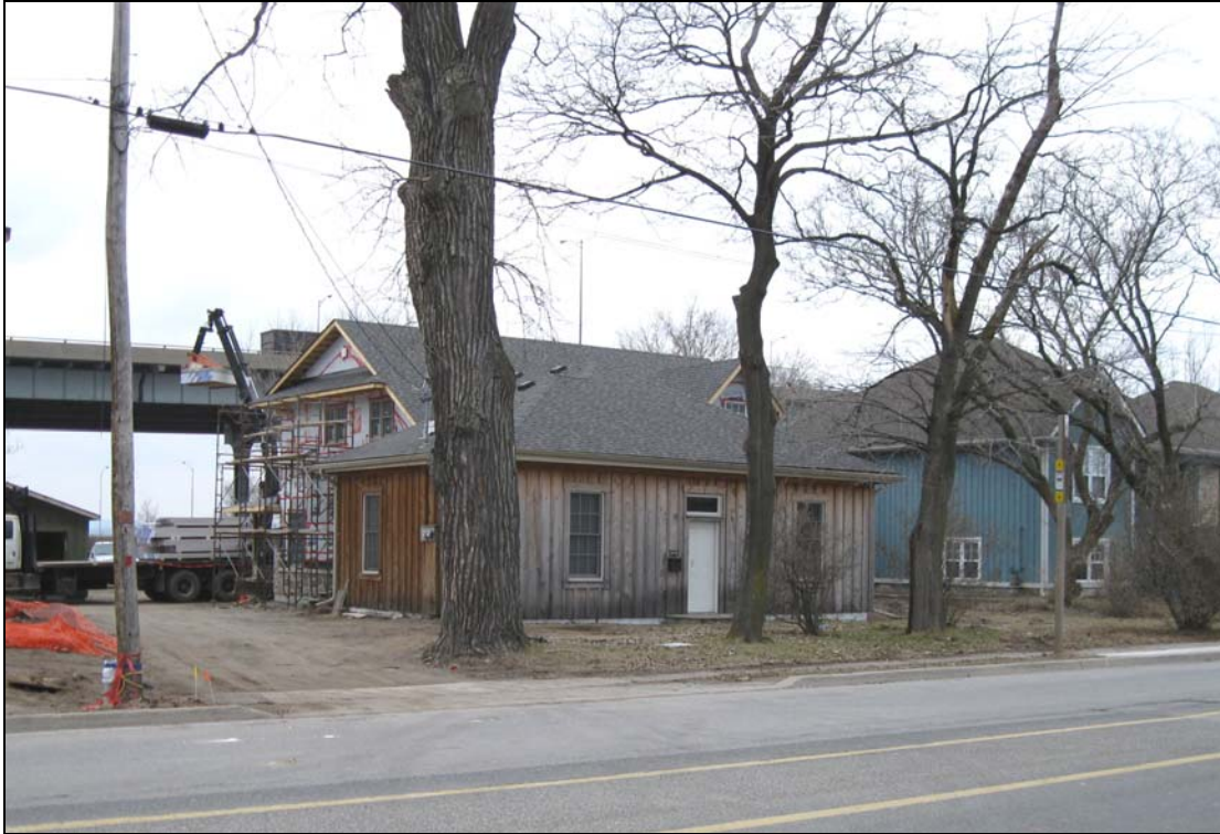
Original cottage and new rear addition from the street (south side)
