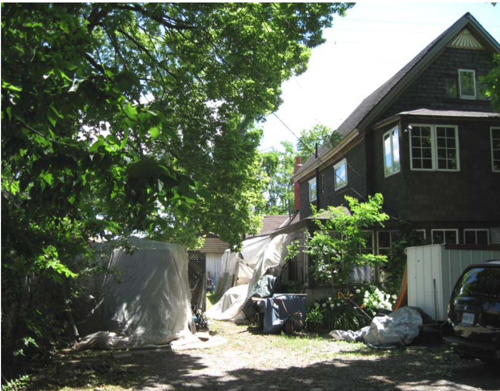
Driveway and side (north) façade of the existing residence.
