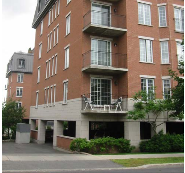
Photo 5.33: Parking within a structure should be screened from view at sidewalk level, and enhanced by architectural detailing, artwork, landscaping or similar treatment that will add visual interest.
