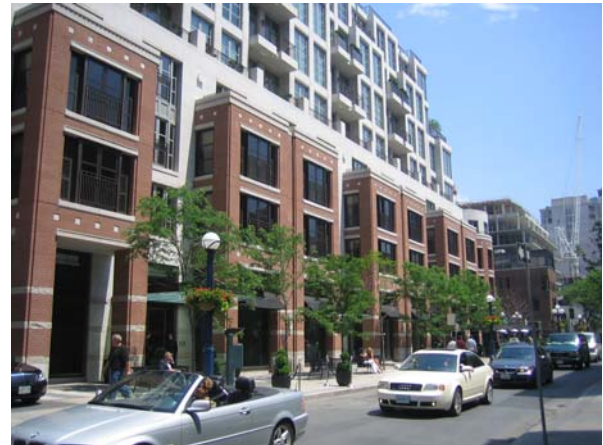
Photo 5.6: Taller buildings (up to 12-storeys) are encouraged provided they are appropriately designed (e.g. stepbacks).
