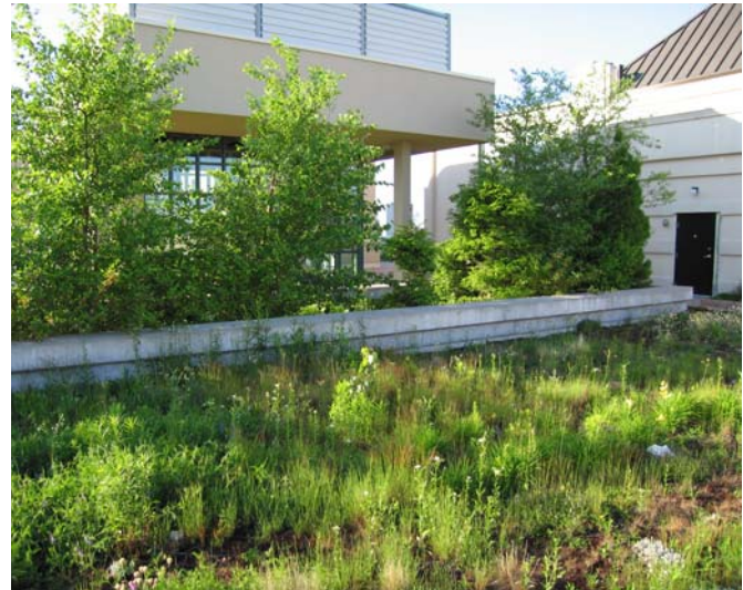
Photo 5.41: Green roofs provide an enjoyable amenity space for building residents and also increase building insulation and minimize run-off.
