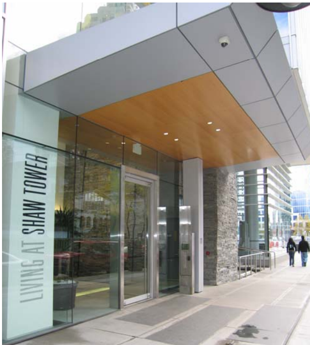
Photo 5.24: Main entrances to buildings should be emphasized through canopies, awnings or taller, non-habitable building structures.
