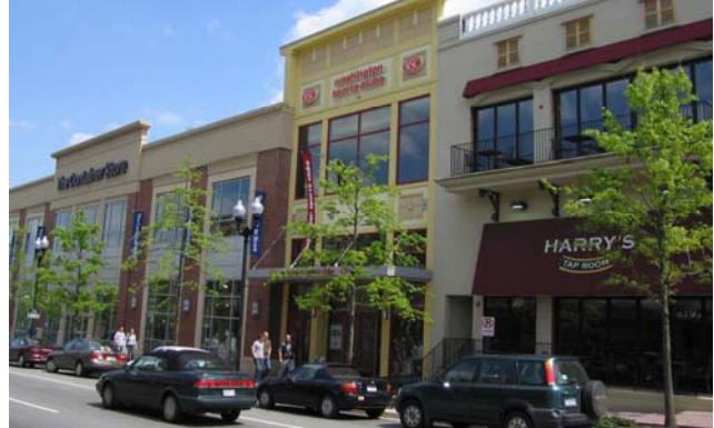
Photo 5.12: Excessively long façades should incorporate architectural detailing, entrance features, recesses and projections along the length of the façade.
