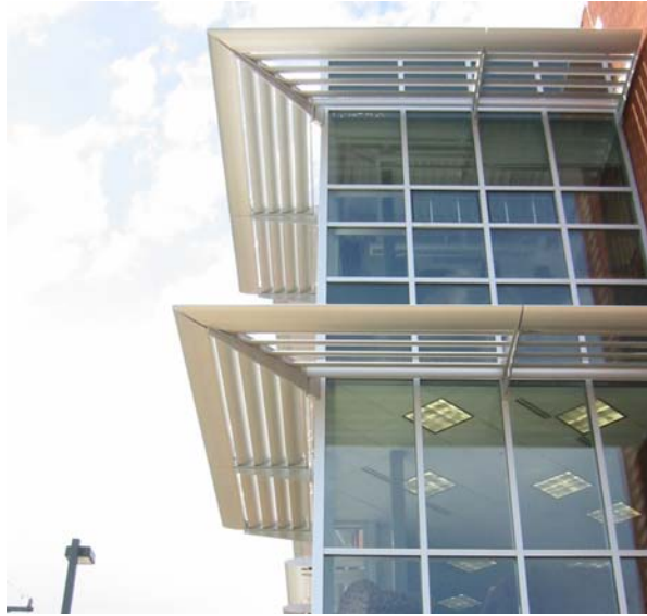
Photo 5.36: Sun shade louvers block the high summer sun but let light in during the winter months.
