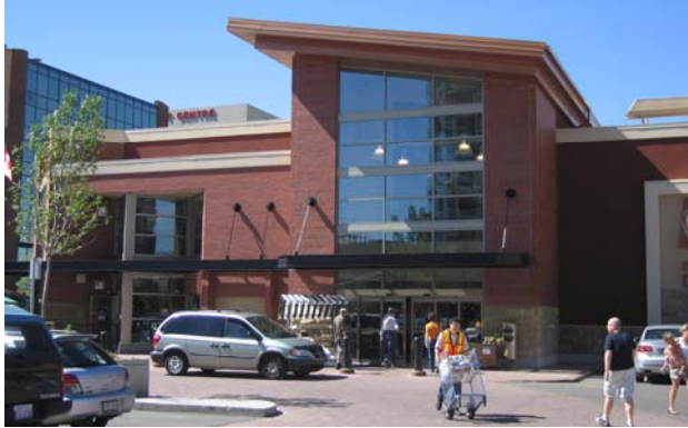
Photo 5.11: The primary entrance design should incorporate high-quality architectural treatments such as clerestory windows and materials.
