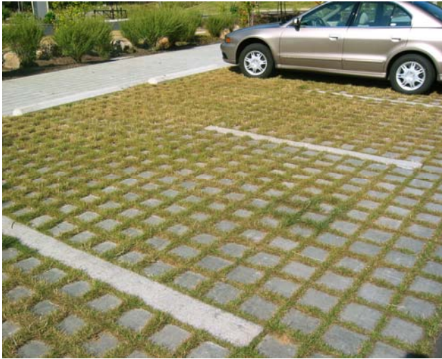
Photo 4.11 & 4.12: Sustainable site design practices, such as permeable paving (Photo 4.11) and swales (Photo 4.12) are encouraged in development adjacent to natural features.
