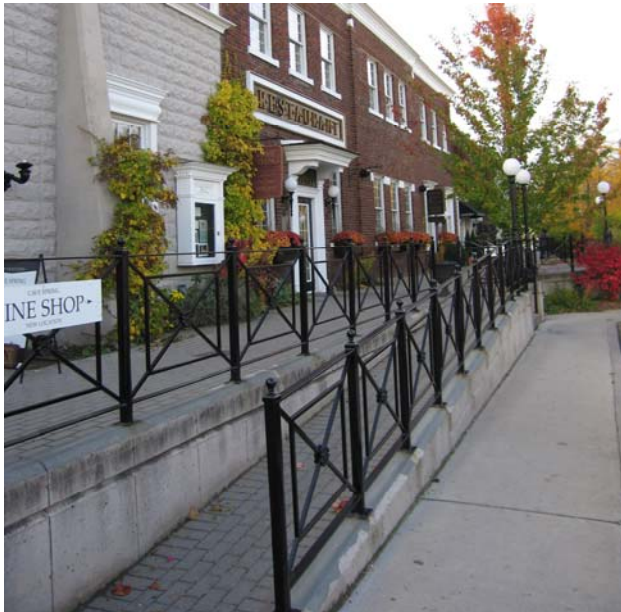
Photo 5.20: Barrier-free accessibility should provide access to the ground level of all buildings.
