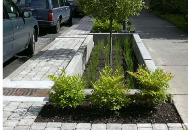
Photo 3.27: Bioswales and/or bio-retention areas can be used to maximize water infiltration and should be incorporated into the design of boulevards.
