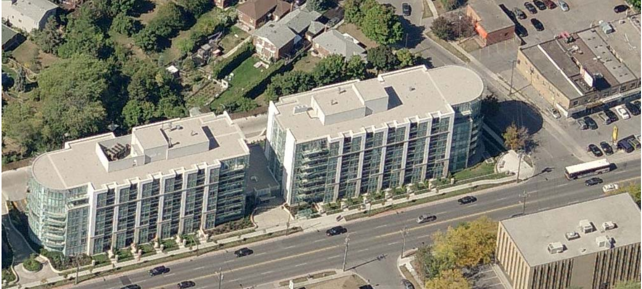
Photo 5.7: The photo above shows how wider sites (i.e. greater than 60 metres) can minimize excessively long façades through well articulated building frontages, or breaking the building into multiple buildings.
