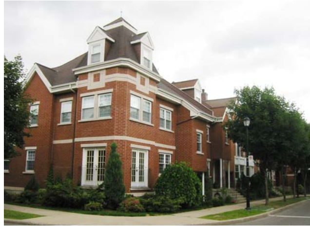
Photo 4.10: On corner lots, the main entrance should be located on the longer side of the dwelling.
