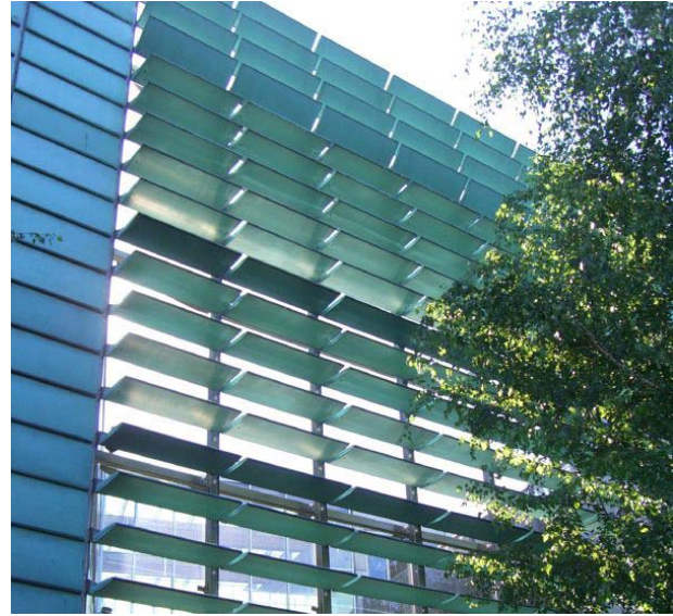
Photo 5.37: Louvers eliminate harsh direct sunlight while maximizing desirable indirect daylighting.
