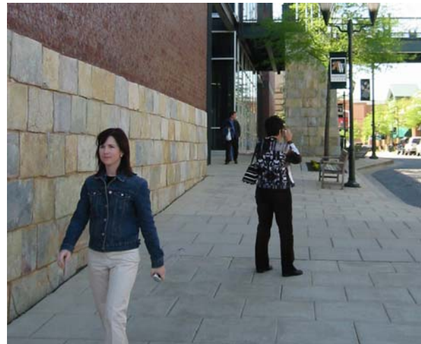
Photo 5.23: Changes in cladding materials provide vertical and horizontal transition.
