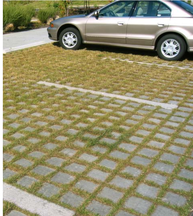
Photo 5.39: A variety of 'green' parking lot design is possible through pavers, planted edges and trees.
