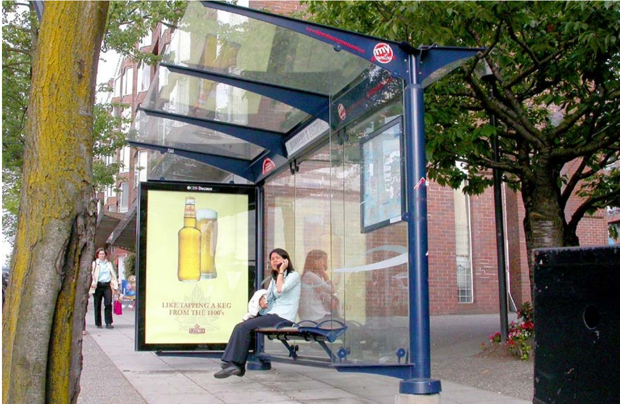
Photo 3.21: As demonstrated in the example above, transit shelters should be weather protected and should provide seating, trash receptacles and route information (Source: www.flickr.com , Spacing Magazine).
