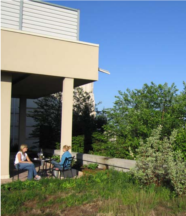
Photo 5.38: Rooftop gardens lower the local temperature, retain water and can provide amenity space.
