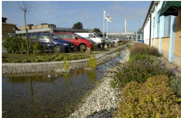
Photos 5.34 & 5.35: Bioswale filters rainwater, prevents run-off and ensures slow percolation into the ground.
