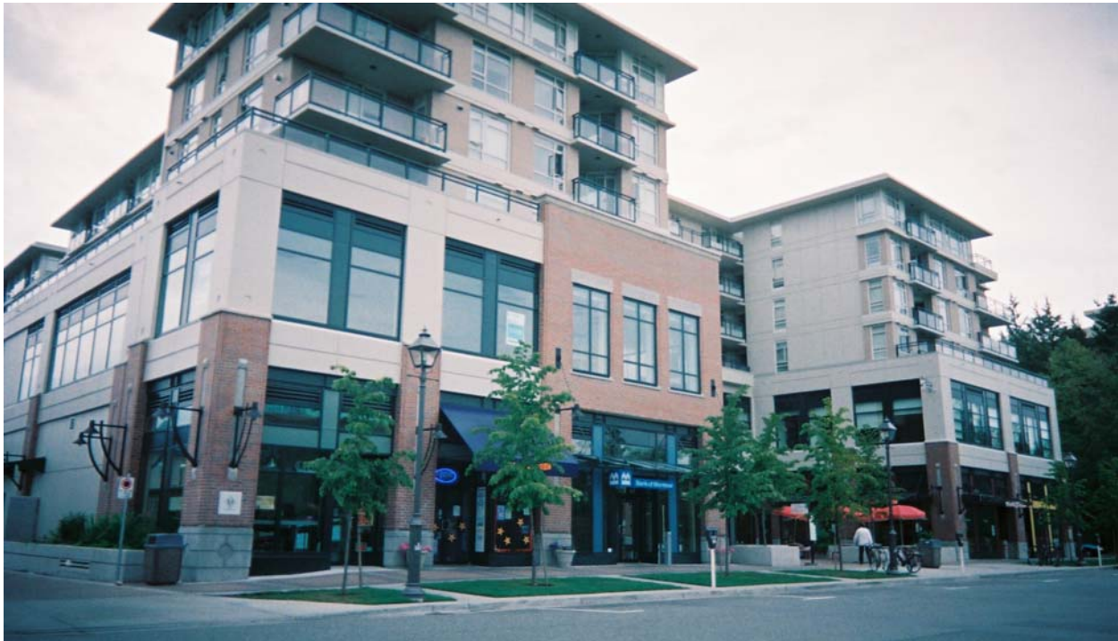
Photo 5.2: A range of residential, commercial and institutional uses should be accommodated in the Mixed Use Medium Area.
