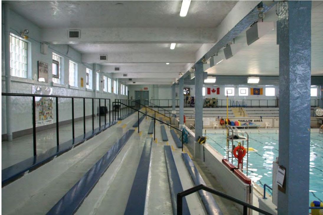
Figure 33: Bleachers on west side showing window patterns, roof posts and beams and 2004 emergency escape door
