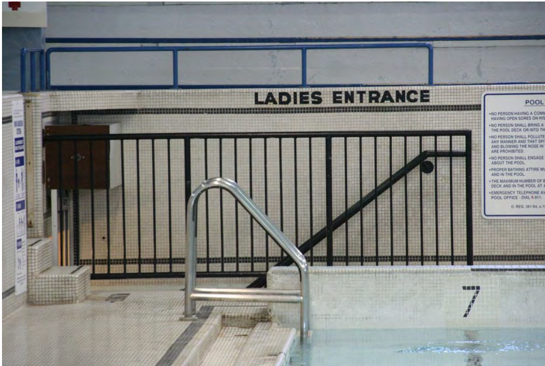
Figure 37: Ladder, barrier tiles, gutter, staircase to women's change room at north west side. The letters are painted
