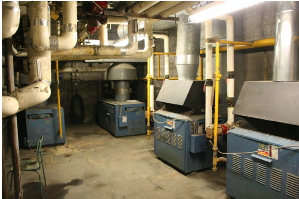
Figure 28: Furnace room containing modern furnaces. The exterior chimney is outside the wall at the furthest furnace.
