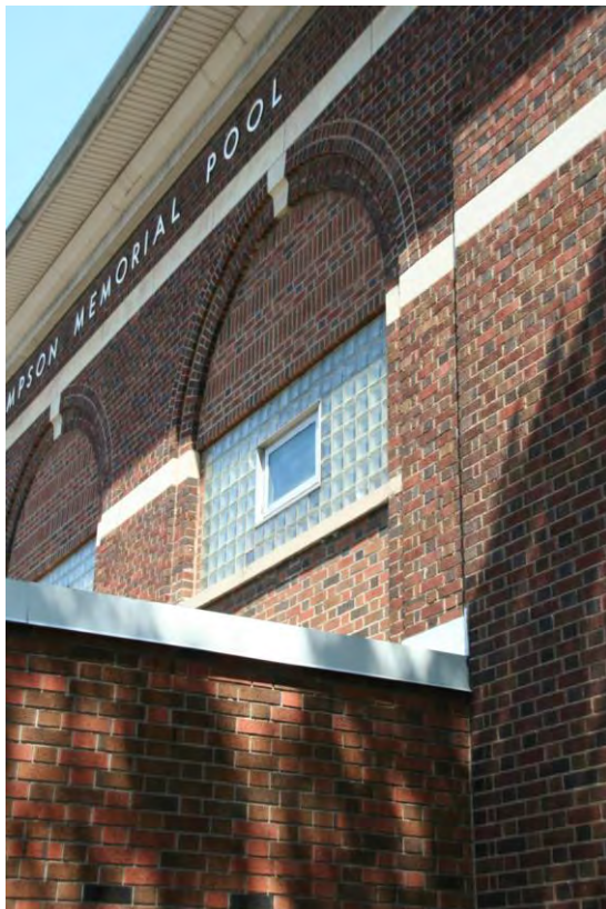
Figure 11: Front (south) Facade detail of brickwork on new addition and original building. Note the decorative brick pattern in the arches.
