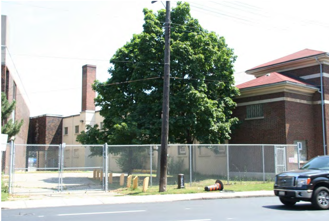
Figure 15: West facade showing brick “bridge” to Scott Park School in rear, behind chimney
