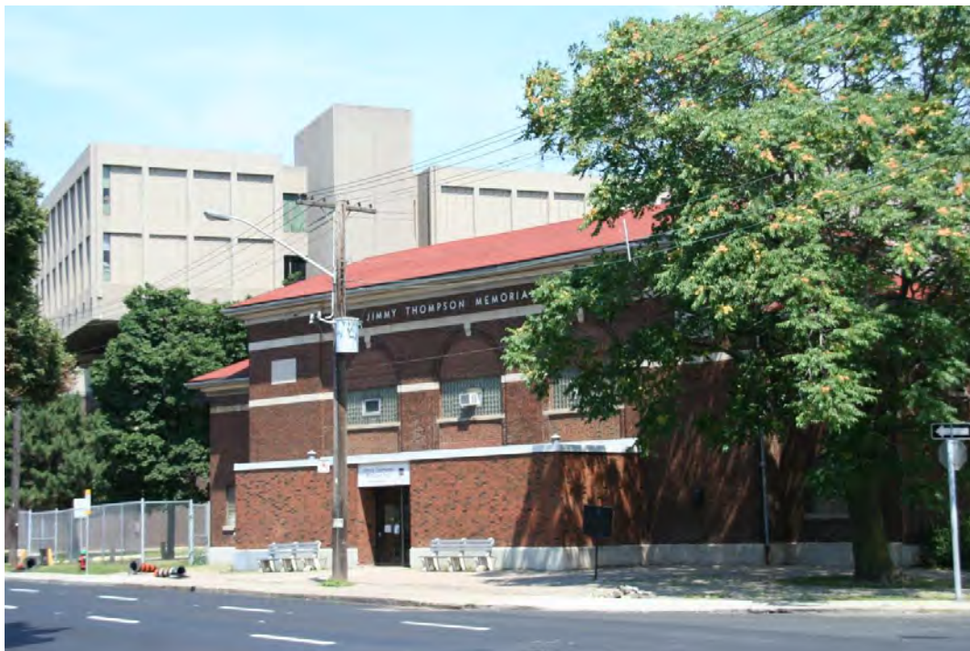
Figure 7: Scott Park Secondary School rising behind the Memorial Pool with King Street in the foreground.
