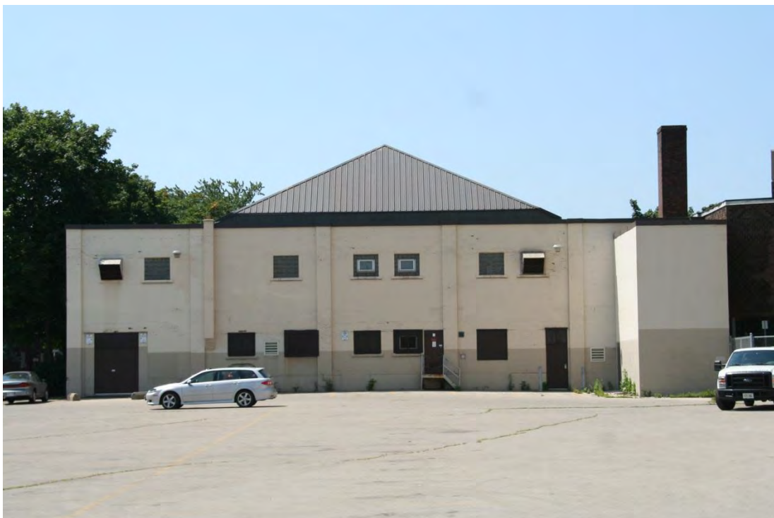
Figure 14: North facade showing hipped roof of skylight, new fire escape extension of right and furnace room chimney
