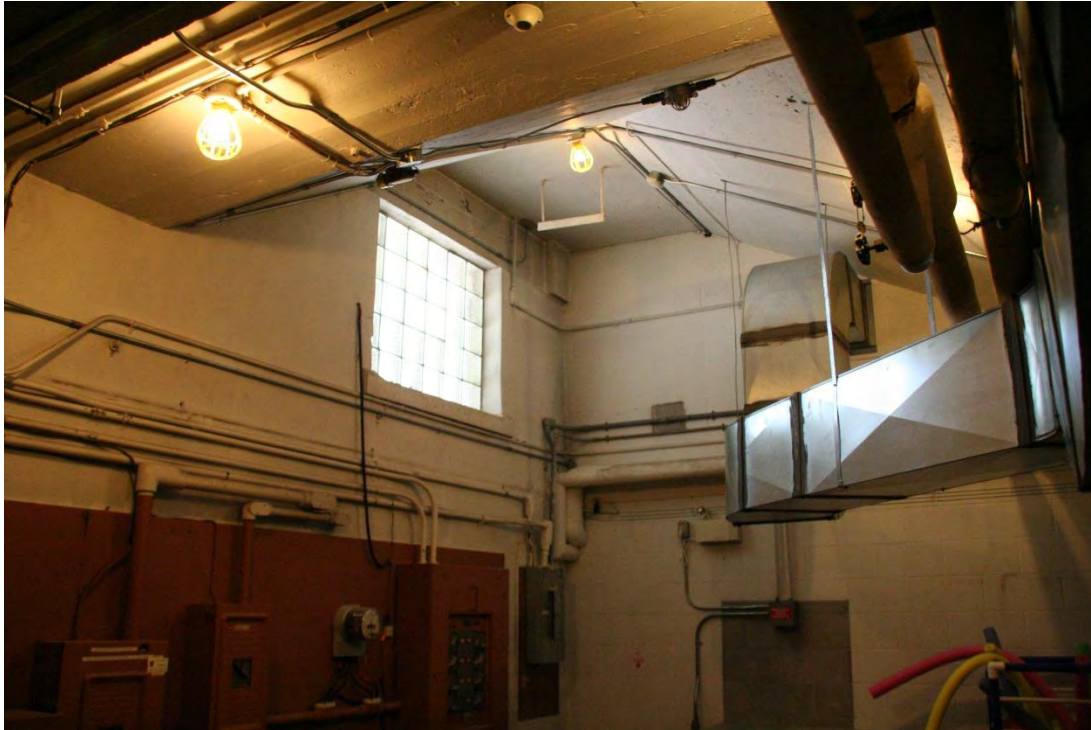
Figure 26: Electrical room showing ground-level windows.
