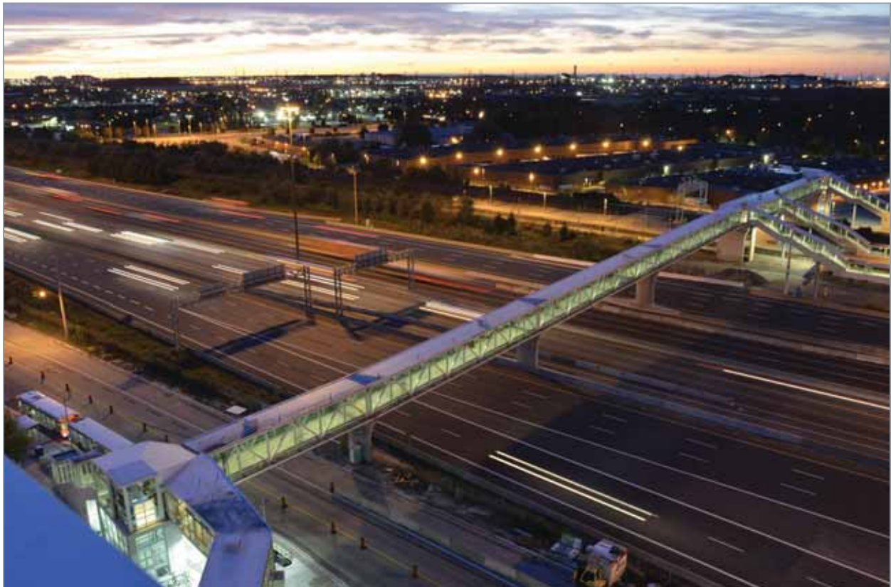
The new pedestrian bridge at Pickering GO Station connects office development to regional transit
