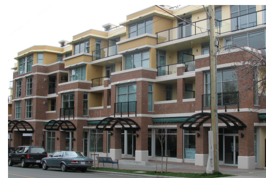
Buildings that are taller than 2 storeys should consist of a base of 2-3 storeys, and the additional floors should be set back from the front face
