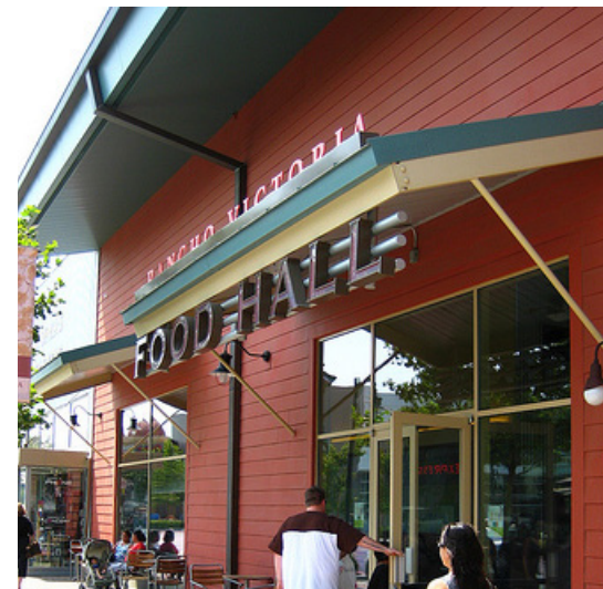
Horizontal building projections such as canopies should be employed for pedestrian comfort
