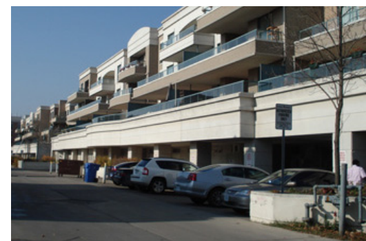
Parking lots should be located internally. Rear yard parking is highly encouraged
