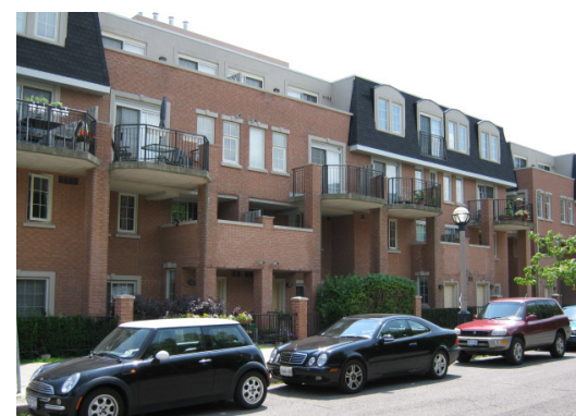
Low to medium density residential intensification should address the existing residential neighbourhood
