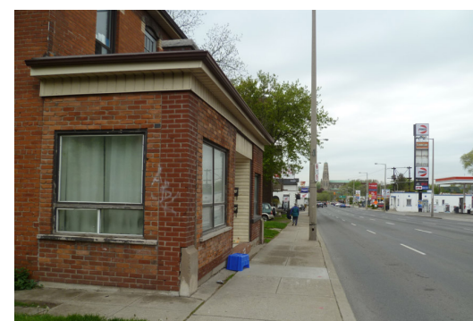
View of Cathedral of Christ the King from King Street West
