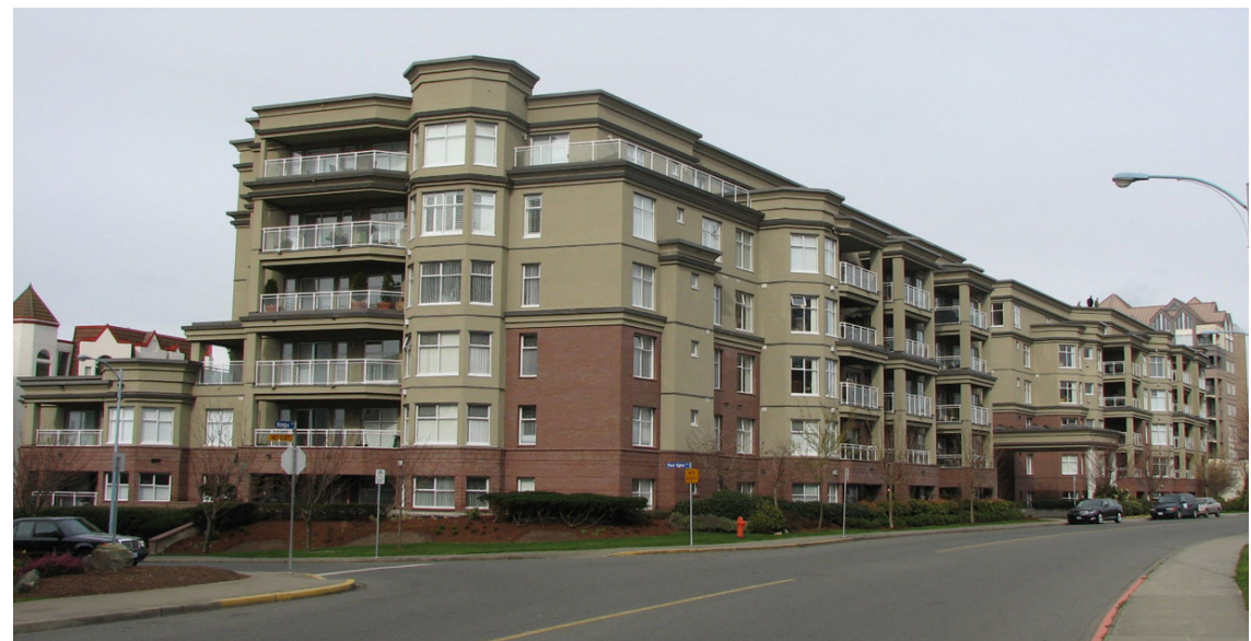
Changes in exterior wall material and colours should articulate a transition between a base and a top for high density high rise residential development
