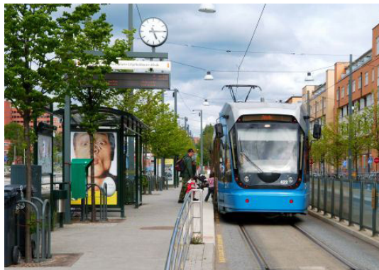
With a higher order rapid transit system proposed along King Street West, street parking or front yard parking will not be permitted
