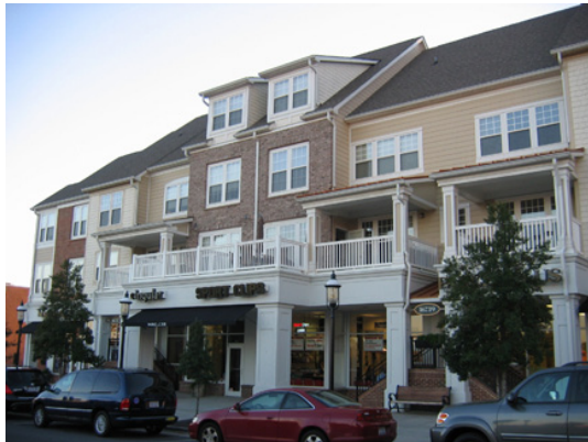
Balconies should be designed as integral parts of the building design
