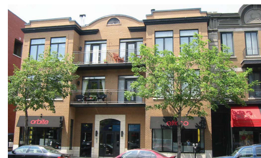
A portion of the building mass should be set back further from the primary face of the built form to accommodate pedestrian spaces
