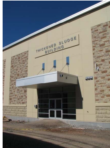
Biogas Enhancement Project Sludge Thickening Building Warranty Period 2013
