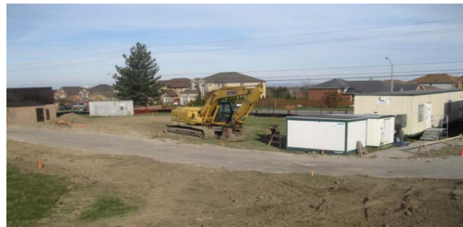
Highland Road Reservoir & Pumping Station Upgrades Construction 2013/2014
