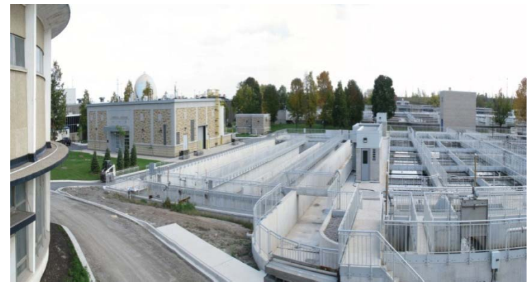
Chlorine Contact Tank
