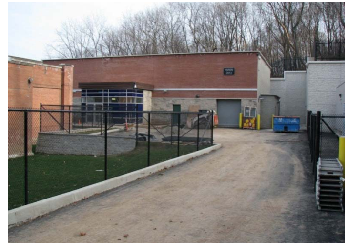
Ferguson Pumping Station 2013
