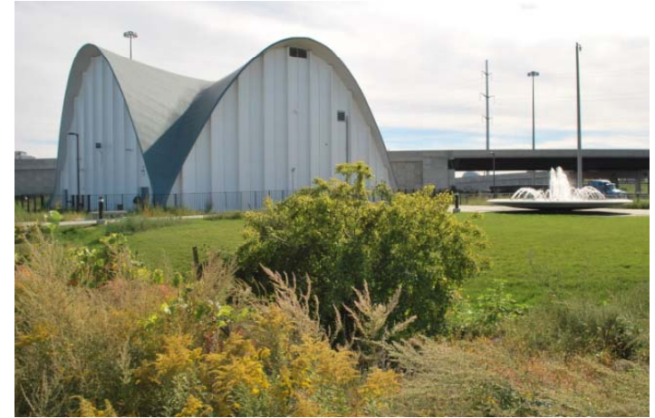
Low Lift Pumping Station
