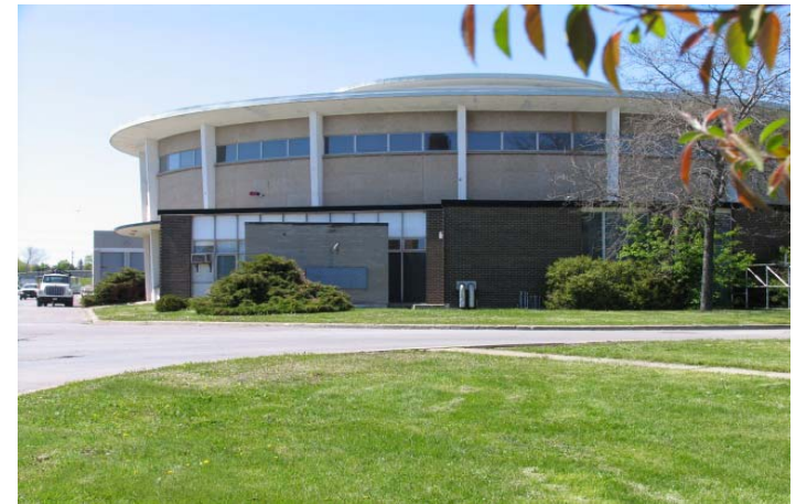
Main Pump House
