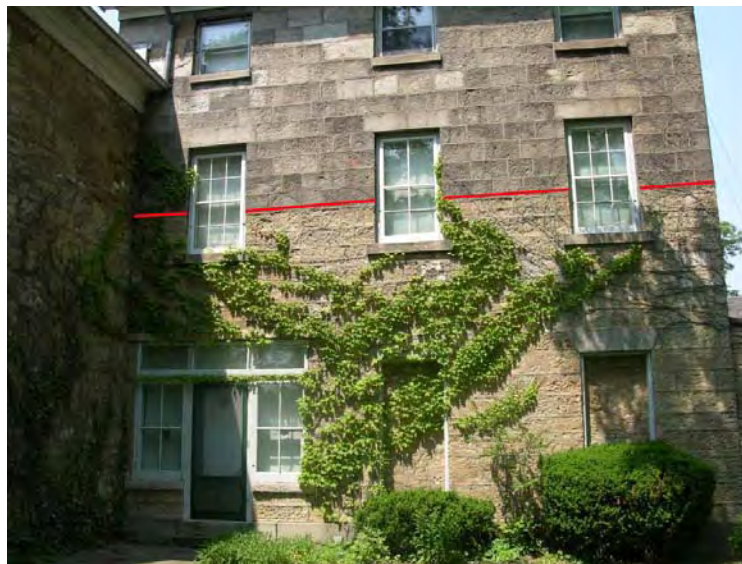
East Wing (south elevation) – Line indicates 1850s addition. There is also eluvial erosion of the limestone below the line
