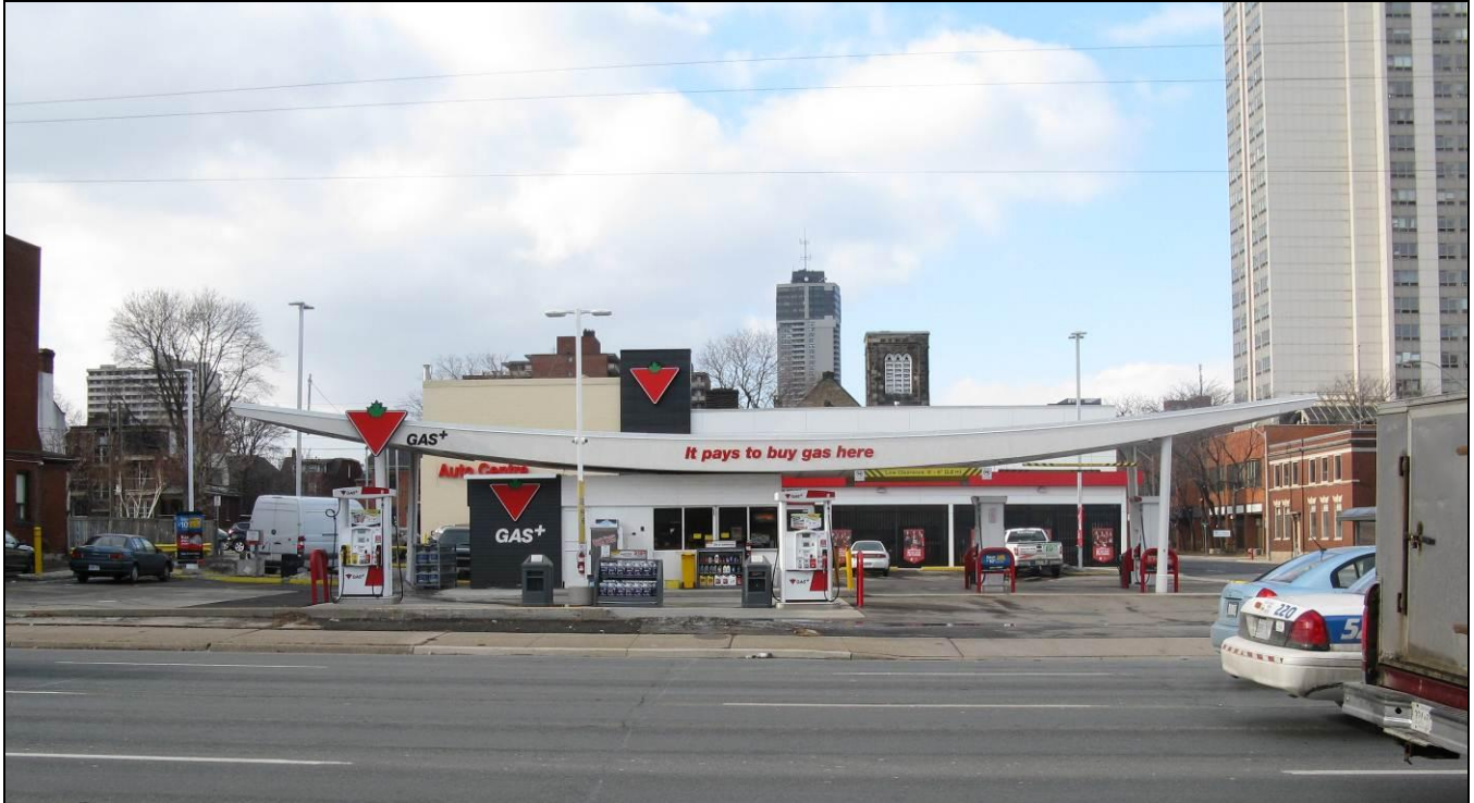
View of the gas bar from Victoria Avenue South
