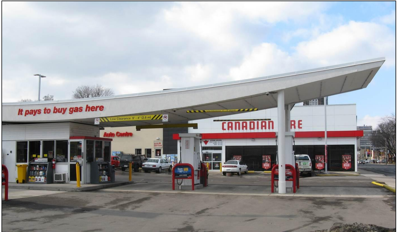
Detail of gas bar
