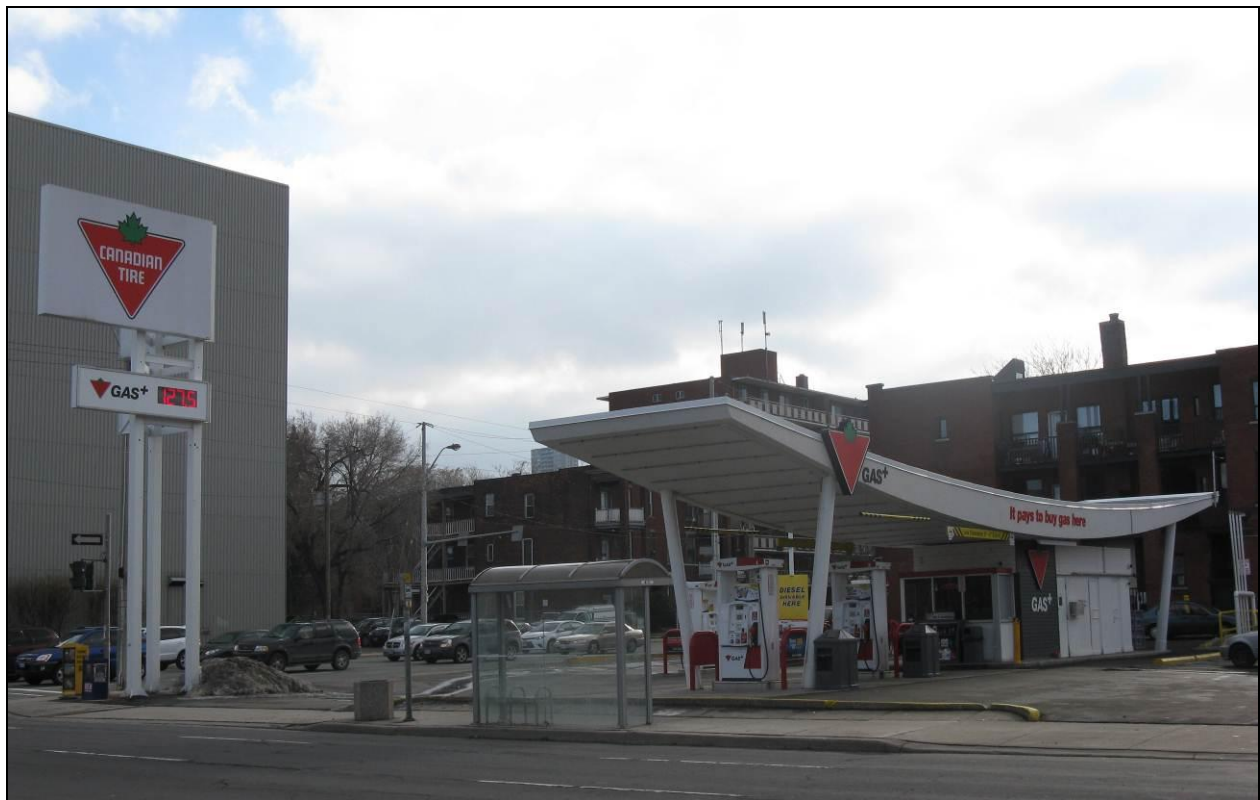
View of gas bar from Main Street East
