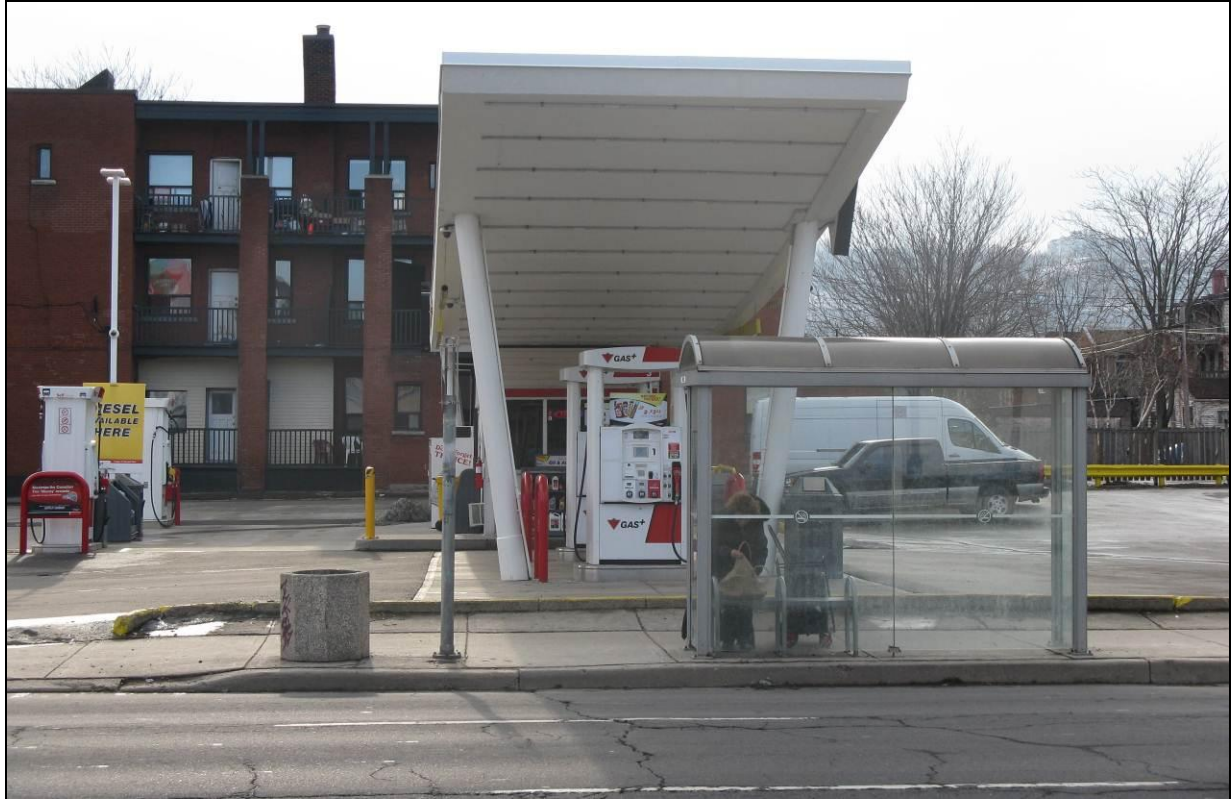
Detail of gas bar canopy showing lighting and angled support columns.
