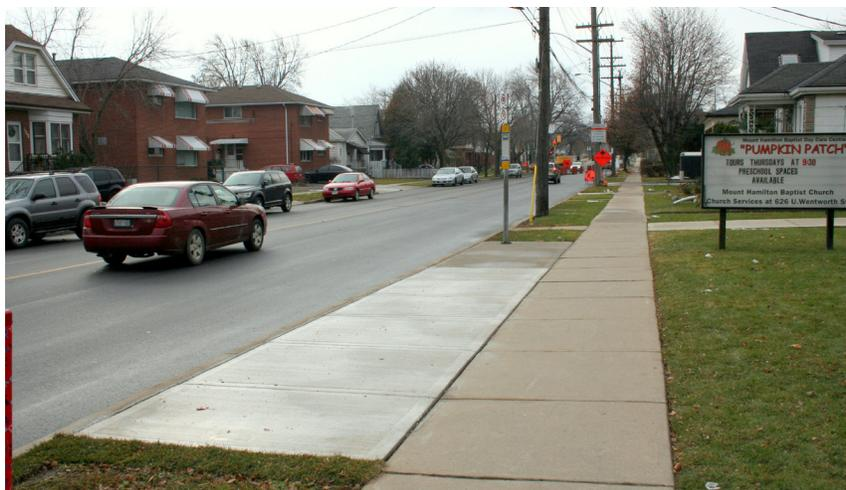
Bus stop on an urban road with a landing pad connected to the sidewalk
