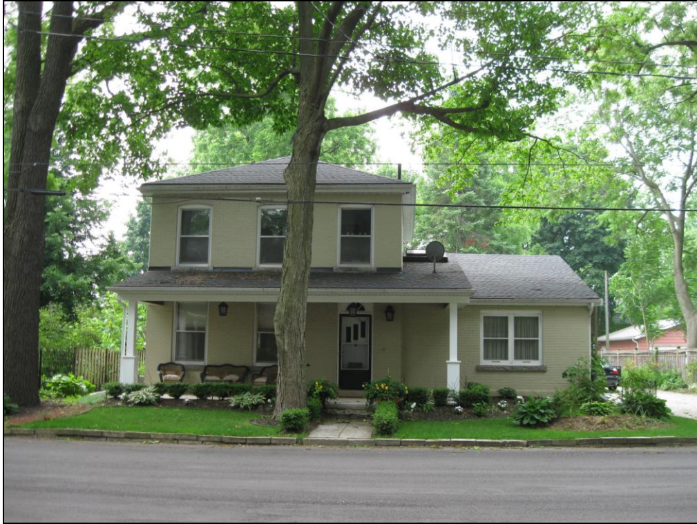
Front (north) façade of the existing house
