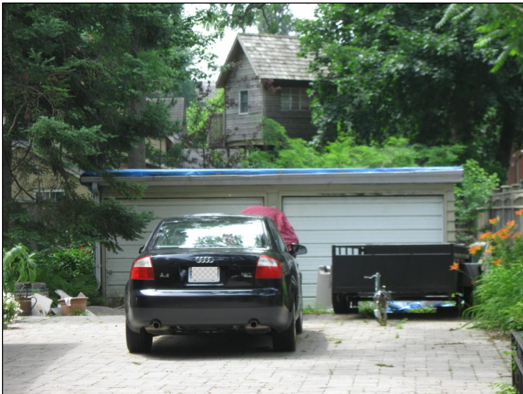
Front (north) elevation of the existing garage.
