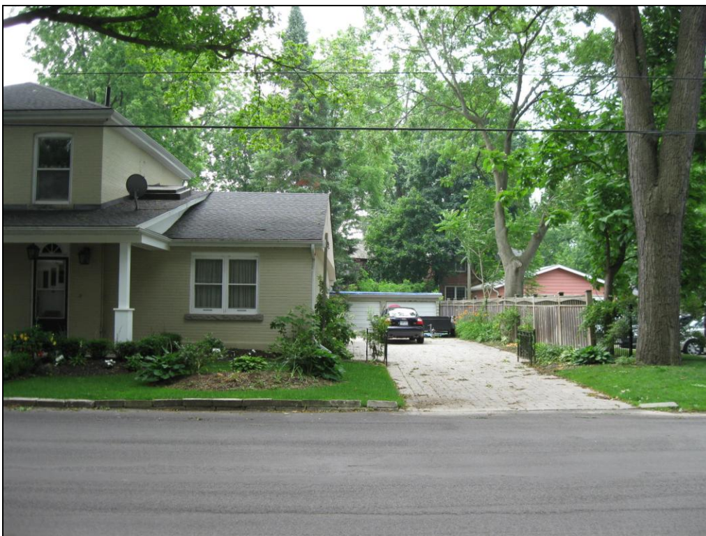
Front (north) and side (west) of the existing house, showing the existing detached garage and driveway
