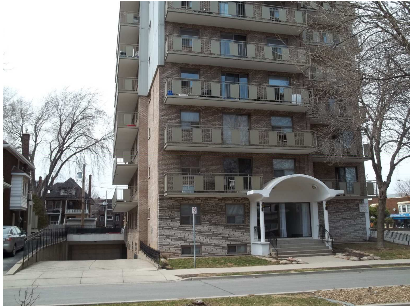
Photo 2 - View of Parking Garage Entrance (West)
