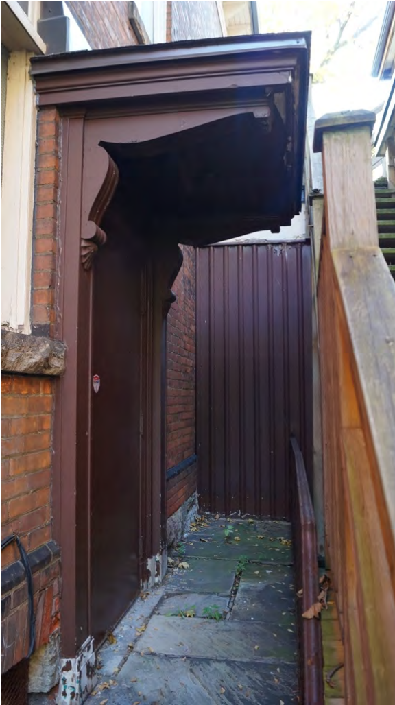
Fig. 52 Canopy over side entrance on west elevation
