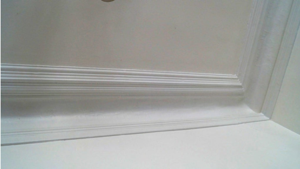
Fig. 76 Plaster moulding at cove ceiling in parlour, curving to round turreted bay
