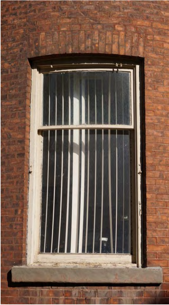
Fig. 36 Ground-floor window in turreted bay. Note sill with parging covering red sandstone.
