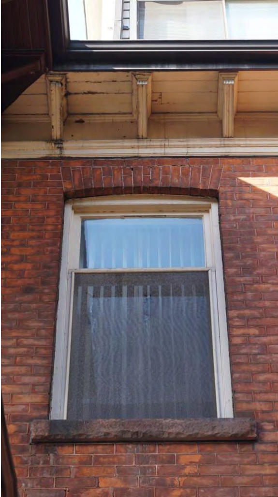
Fig. 46 East elevation's upper window in middle bay
