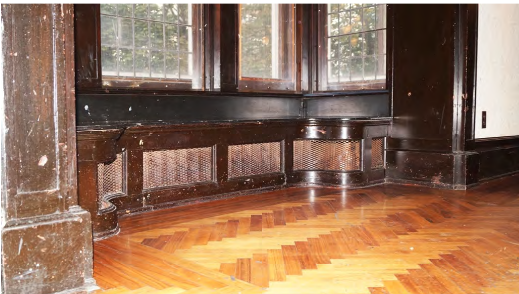
Fig. 195 Bench below oriel window and parquet floor
