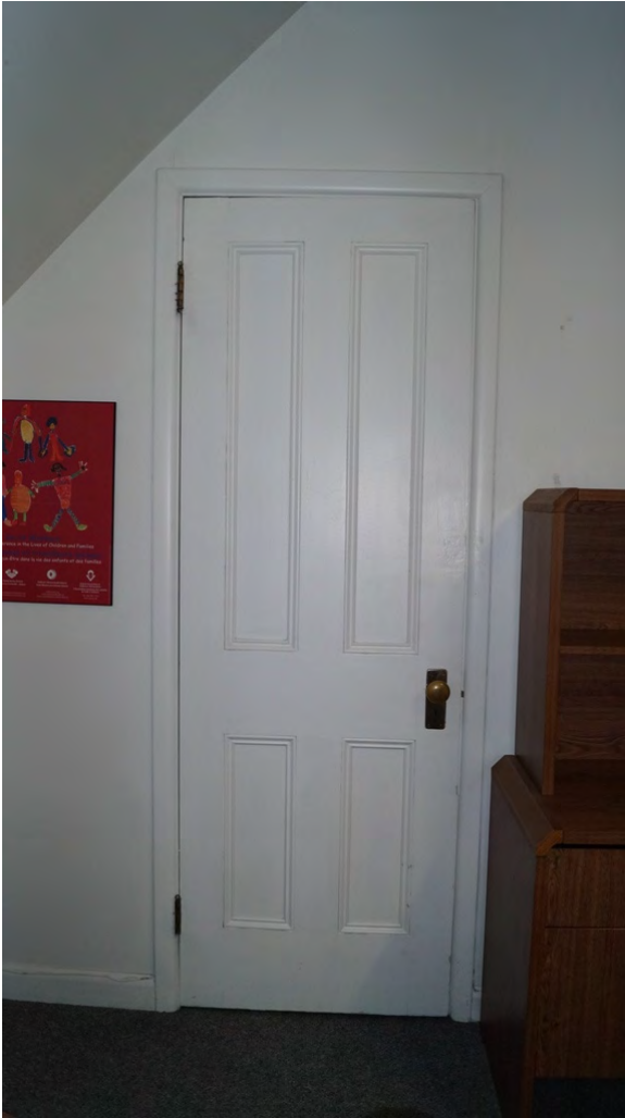
Fig. 122 Four-panelled closet door in attic-floor middle room
