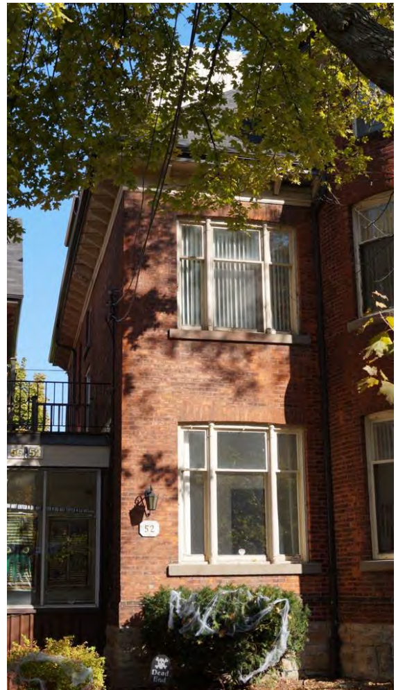
Fig. 39 West bay of front facade
