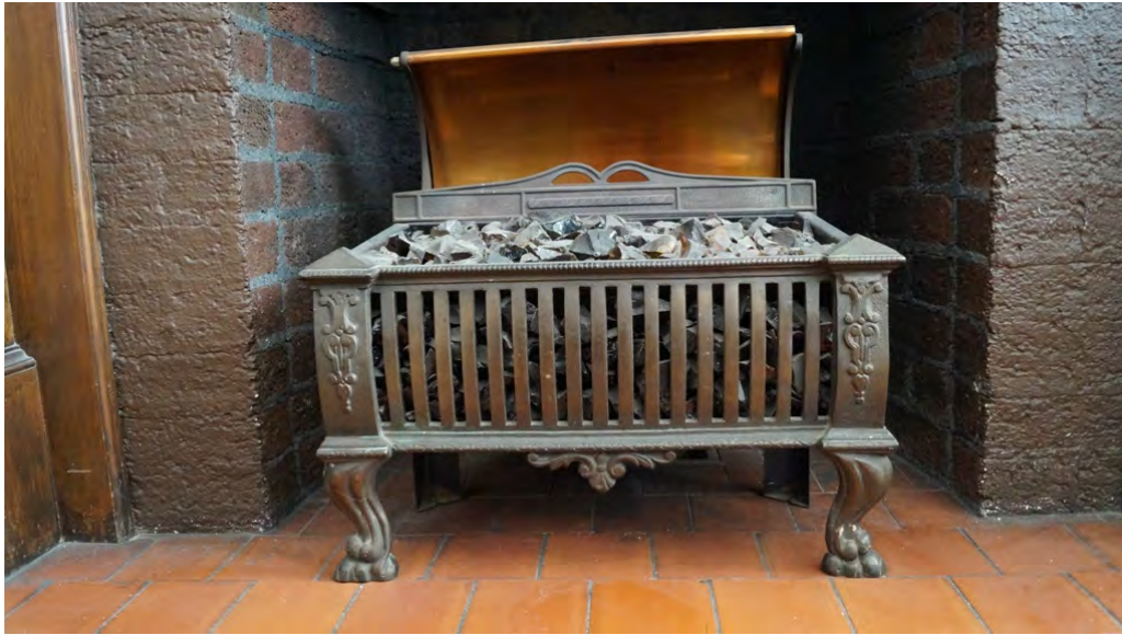
Fig. 74 Electric fireplace grate
