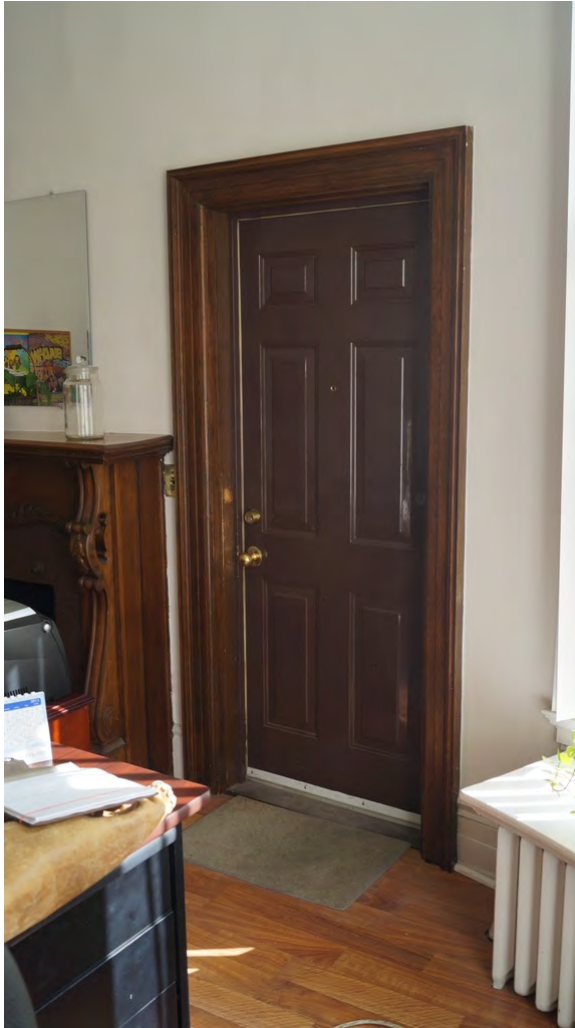
Fig. 72 Doorway between parlour and porch. Note door is also a replacement.
