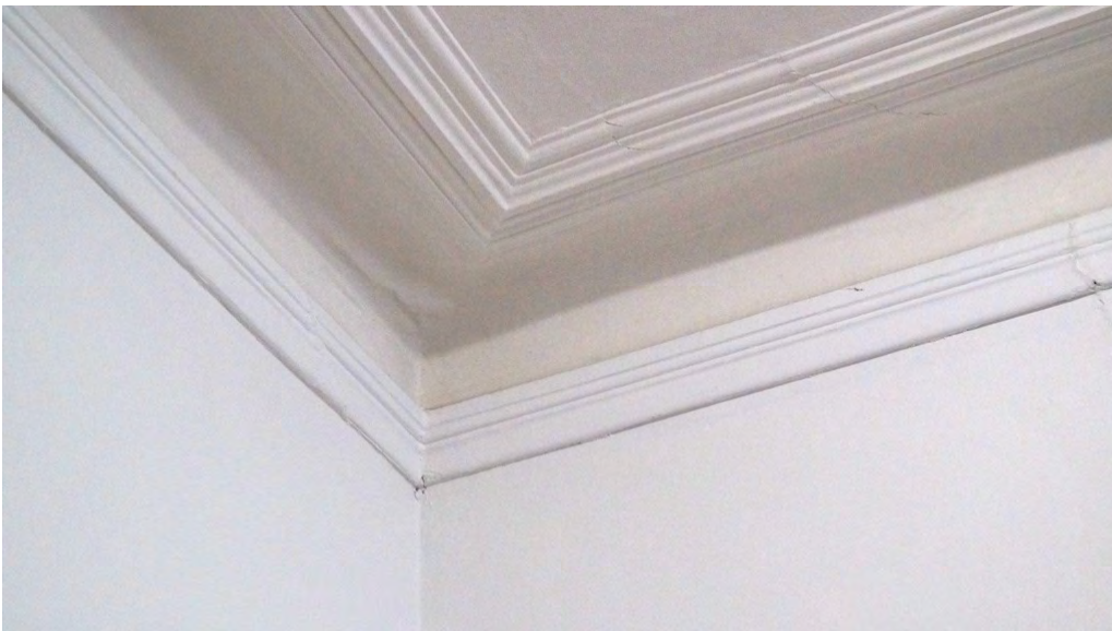
Fig. 91 Silk-covered plaster moulding at cove ceiling in dining room
