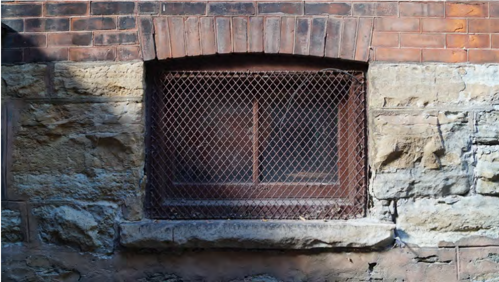
Fig. 44 East elevation's basement window in middle bay
