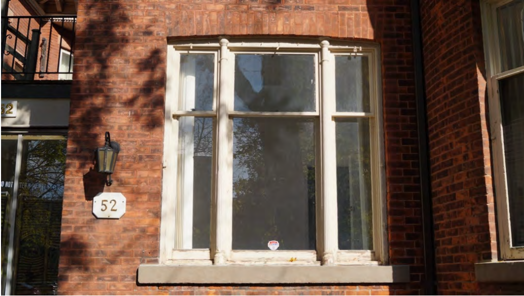
Fig. 40 Ground-floor tripartite window in west bay
