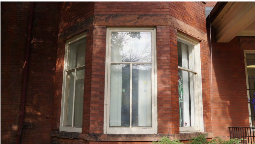
Fig. 137 Ground-floor windows of bay window
