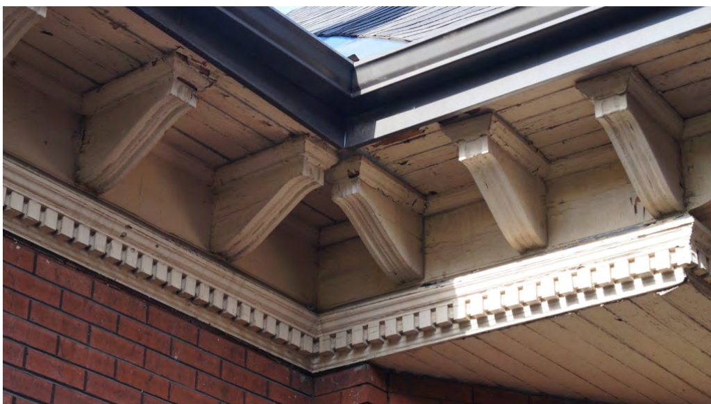
Fig. 149 Detail of east elevation's cornice with dentils and moulded brackets
