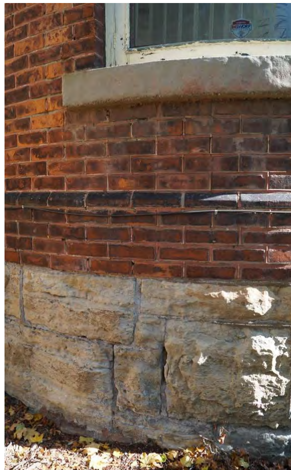
Fig. 29 Detail of rock-faced limestone foundation and red pressed brick wall above – the red brick laid in stretcher bond with red-tinted raised mortar joints and white lime taping
