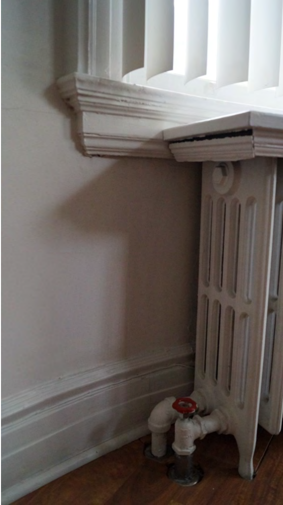
Fig. 102 Curving baseboard, cast-iron radiator and window surrounds in upper-floor turret room
