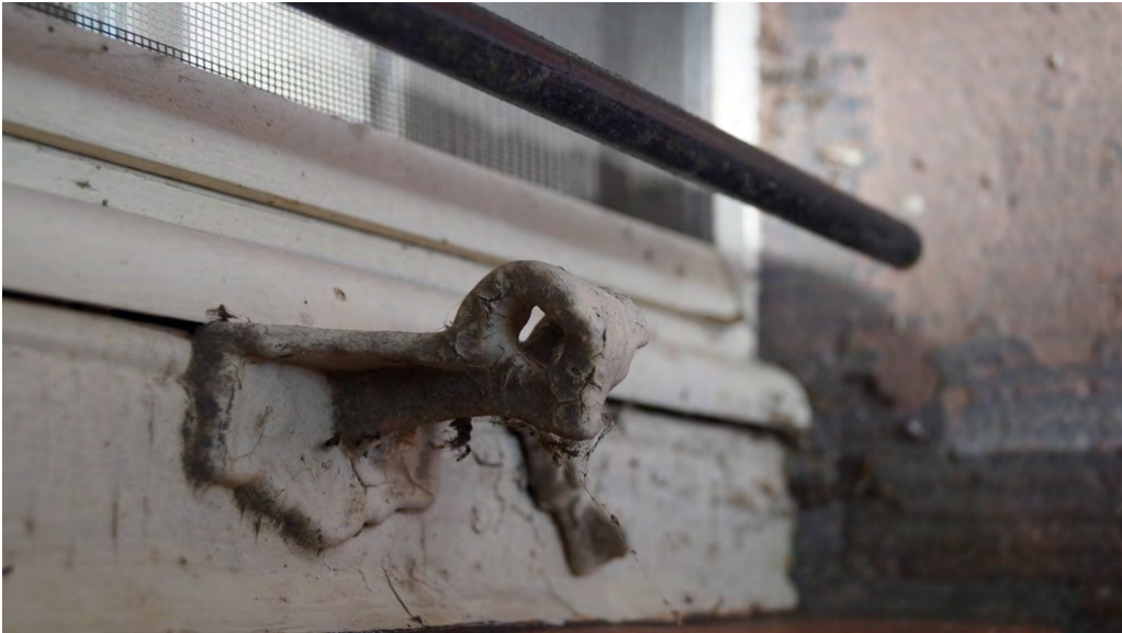
Fig. 134 Ground-floor tripartite window shutter bracket
