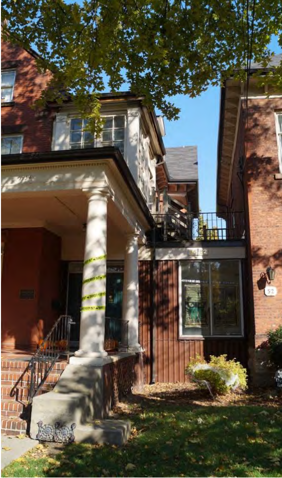
Fig. 26 Exterior of link between 56 Charlton Avenue West on the left and 52 Charlton Avenue West on the right
