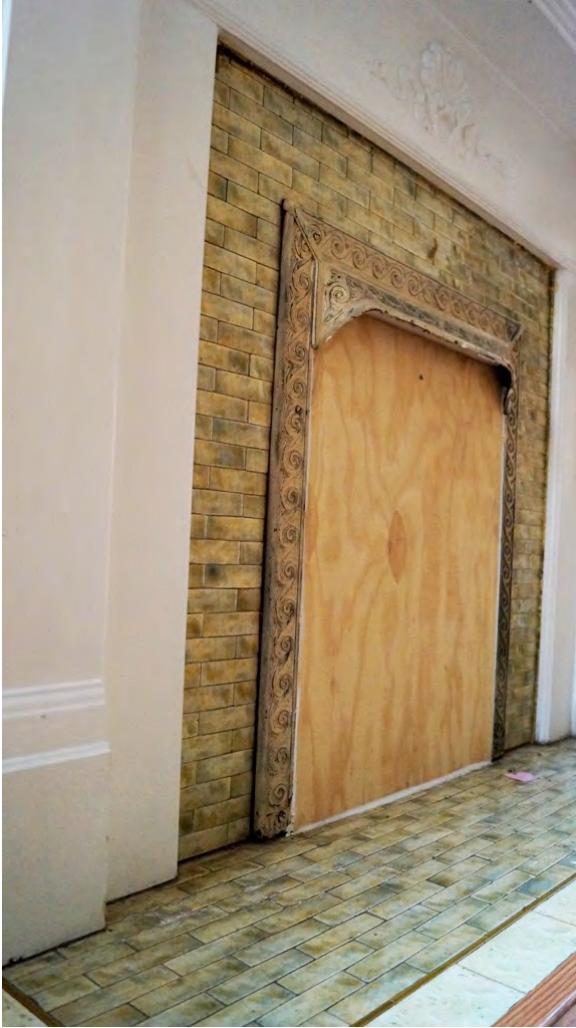
Fig. 226 Detail of hearth, surrounds and floor at northeast bedroom's fireplace
