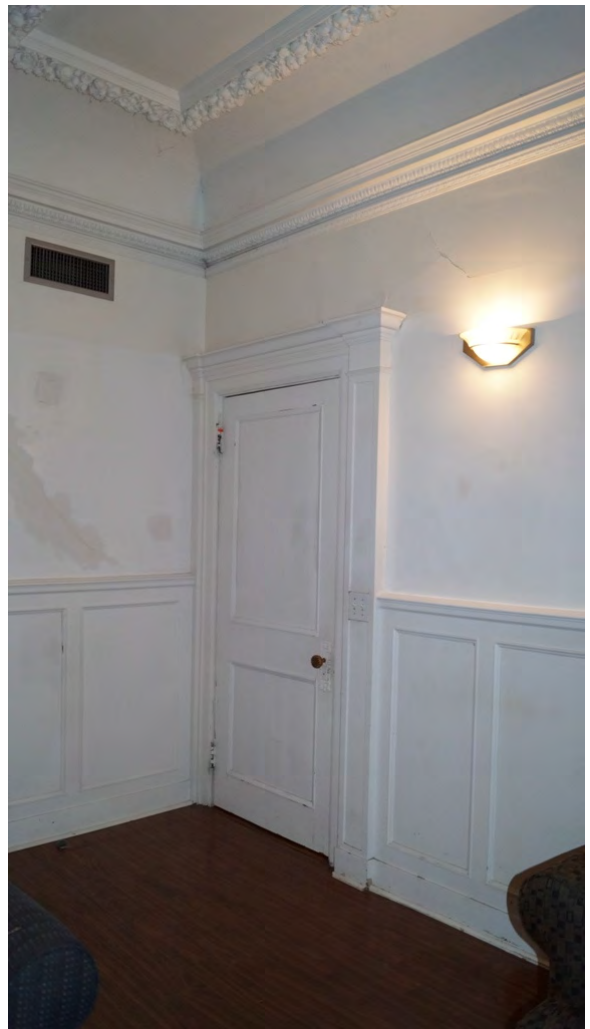
Fig. 177 Northeast corner of connecting room, showing inside face of door, wainscoting, plaster and plaster beamed ceiling
