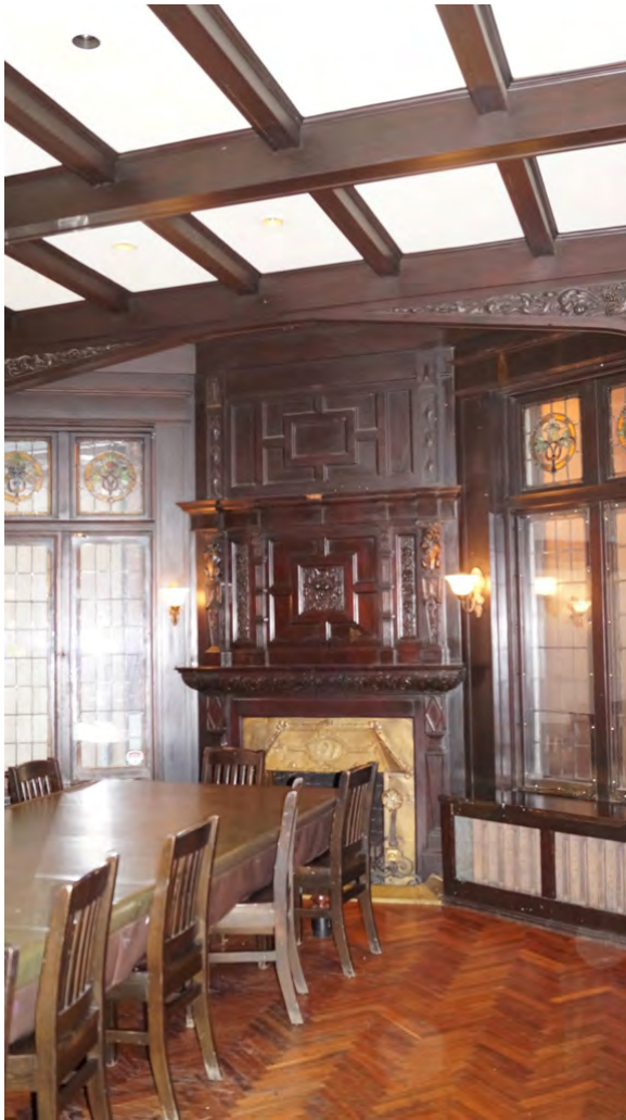
Fig. 188 Detail of dining room's east bay wall. Note herringbone parquet floor.
