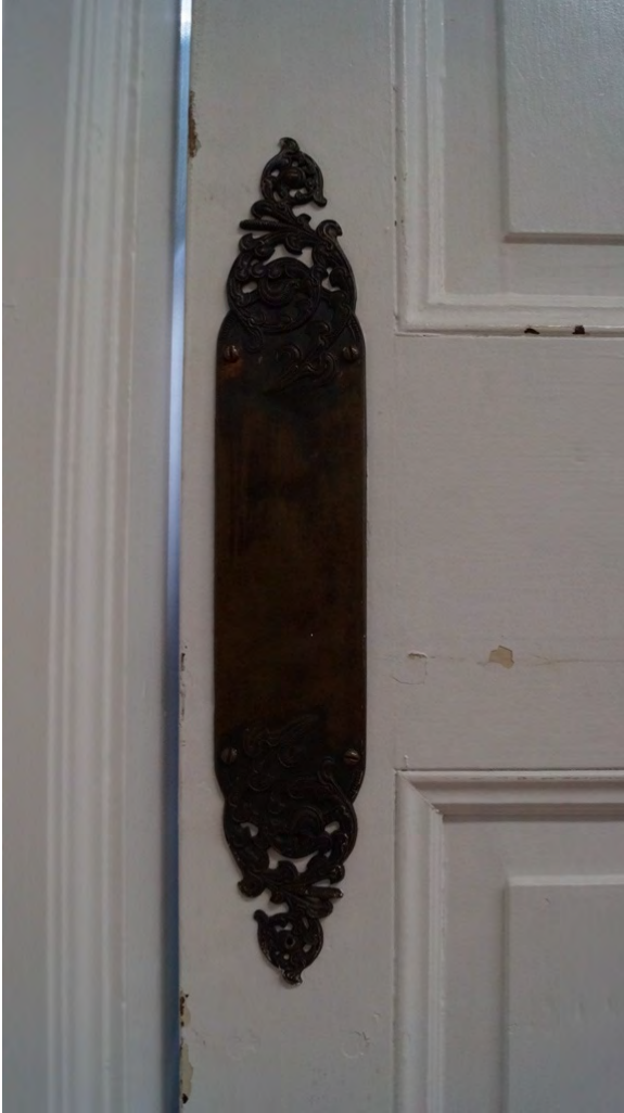
Fig. 90 Escutcheon on dining room swing door
