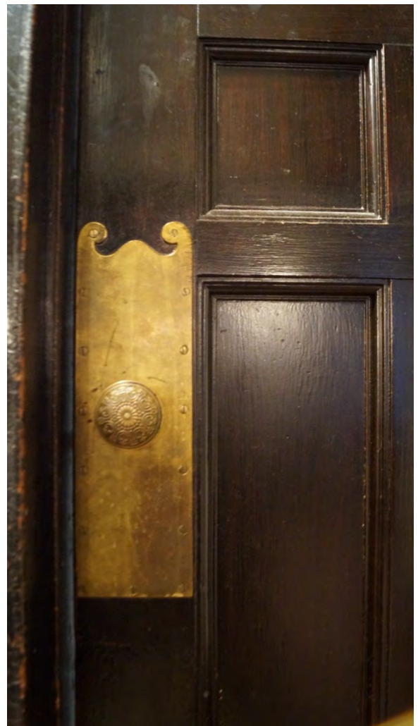
Fig. 199 Escutcheon and door knob on dining room's door to kitchen
