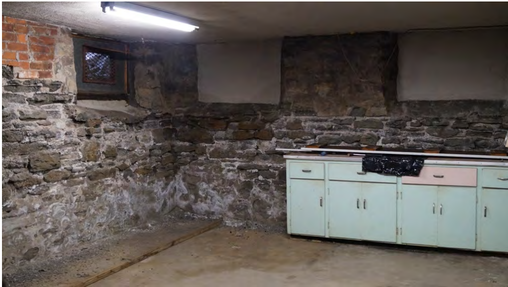
Fig. 63 Basement boiler room
