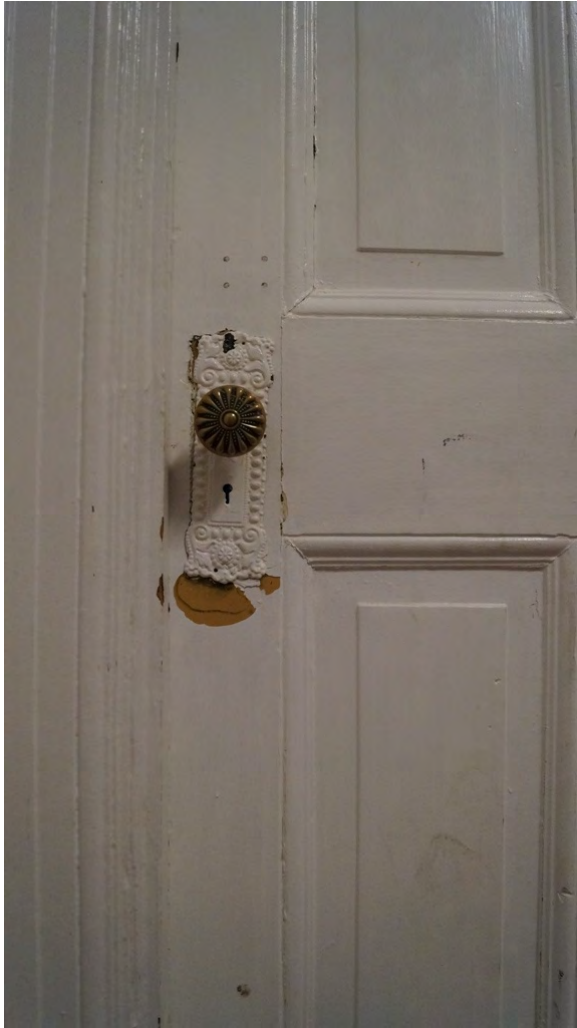
Fig. 176 Door hardware on front entry stair hall door to connecting room
