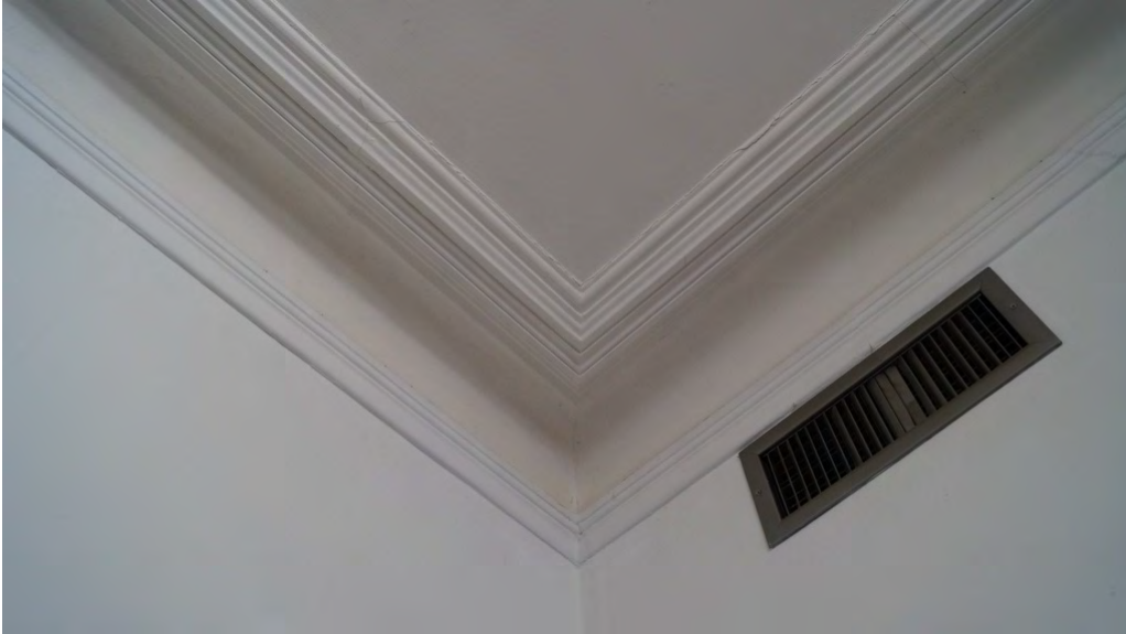
Fig. 68 Plaster moulding at cove ceiling in entry hall
