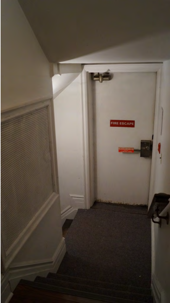
Fig. 61 Stairs to basement
