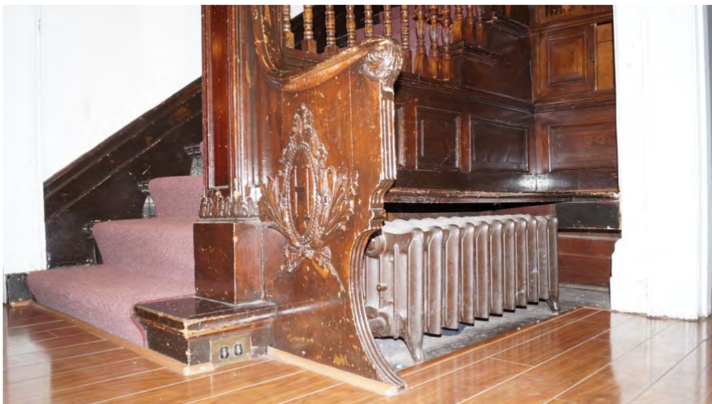
Fig. 205 Staircase bench embossed with the initial "H" for Hobson and cast-iron radiator below
