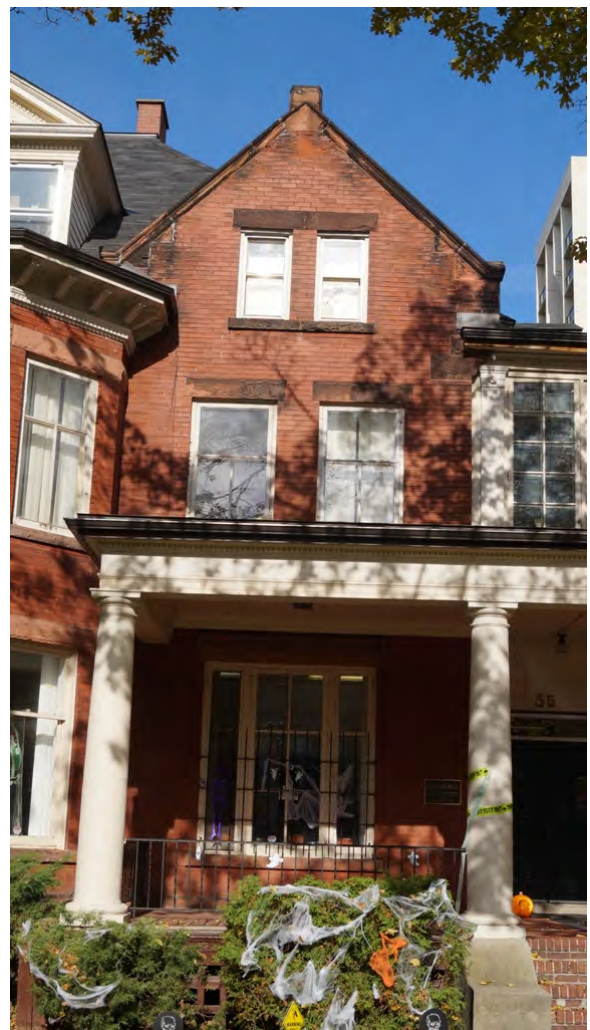
Fig. 131 Front facade's gable bay
