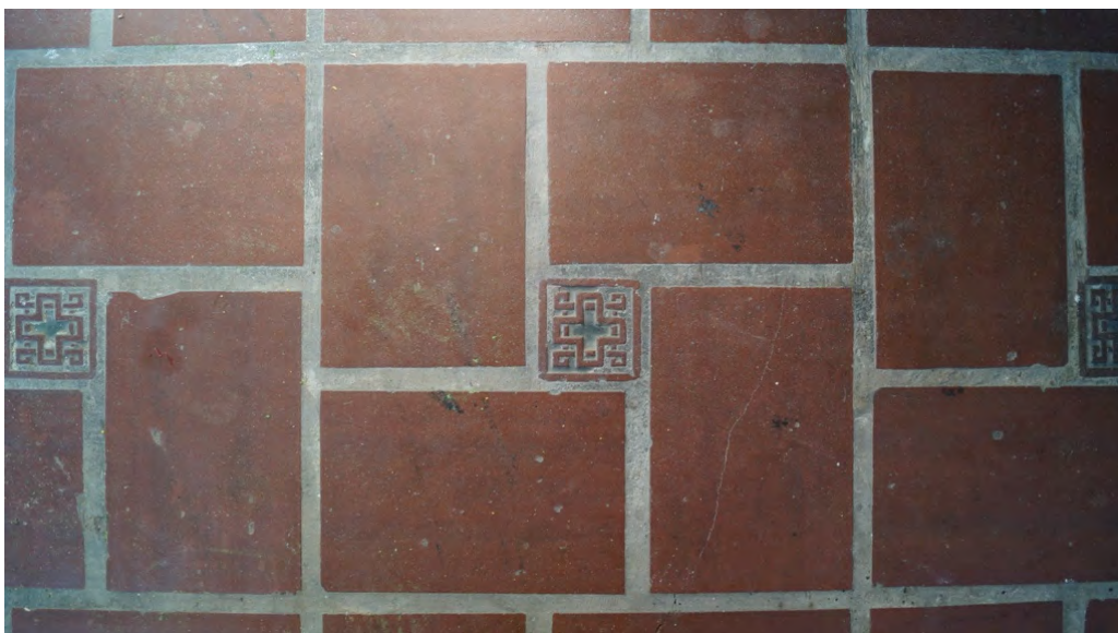
Fig. 219 Detail of quarry tile floor in sun porch
