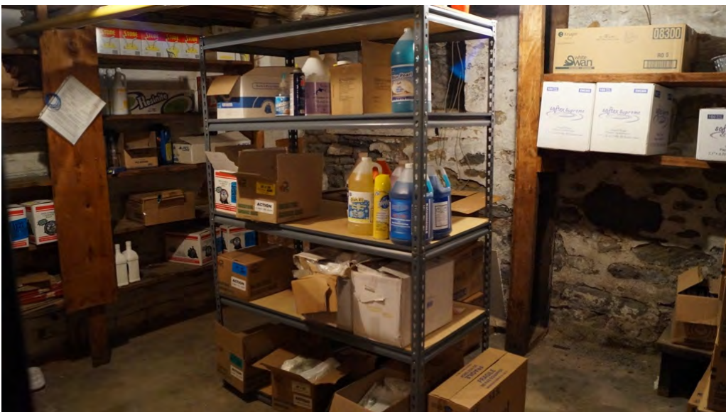
Fig. 159 Food storage vault in basement. Note parged rubble stone foundation walls.
