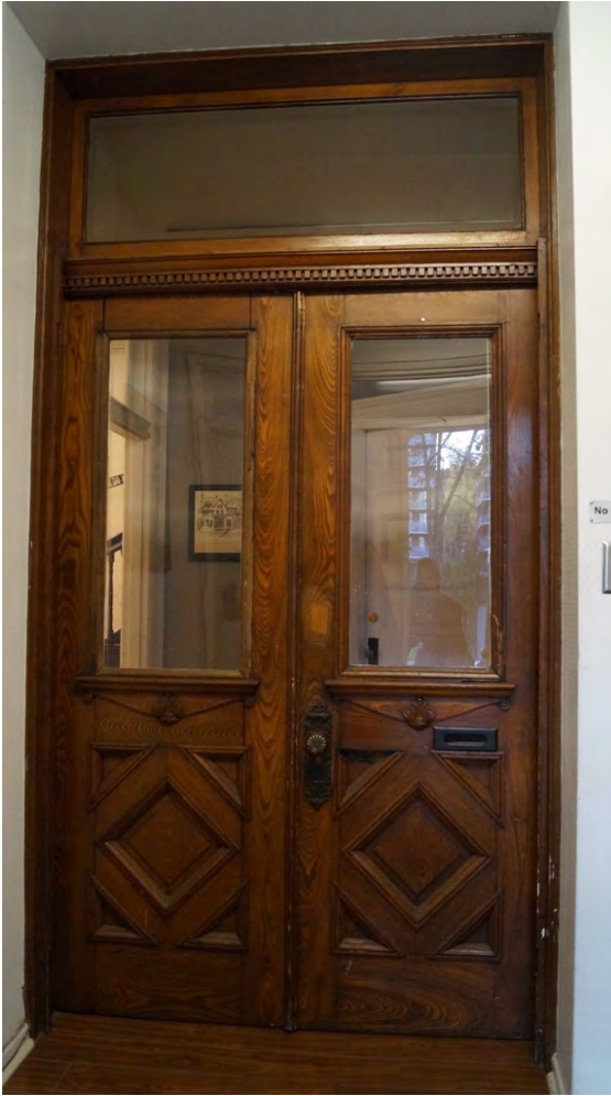
Fig. 162 Original front doorway with transom light over double leaves
