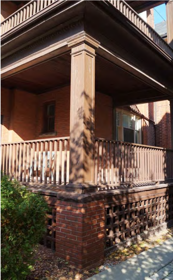
Fig. 32 Detail of porch as seen from the ground
