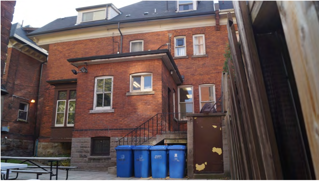
Fig. 150 Rear elevation. Note red brick back wing on concrete block foundation.
