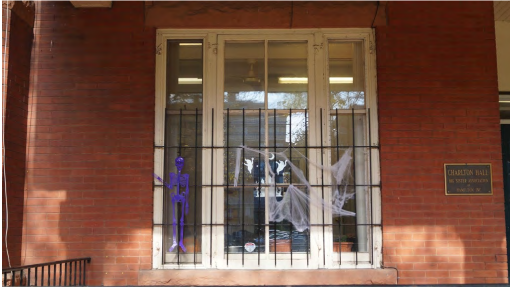
Fig. 132 Ground-floor tripartite window with sandstone sill and lintel
