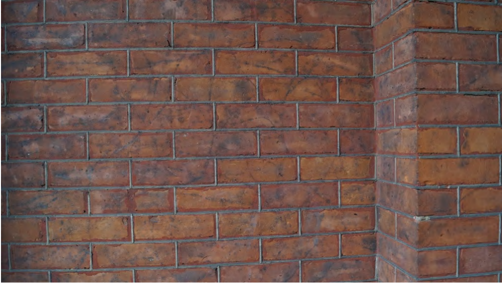
Fig. 30 Detail of brickwork as seen from upper floor of porch
