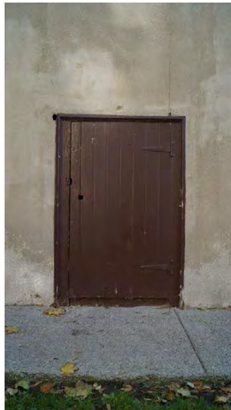
Fig. 59 Coal chute door in back wing
