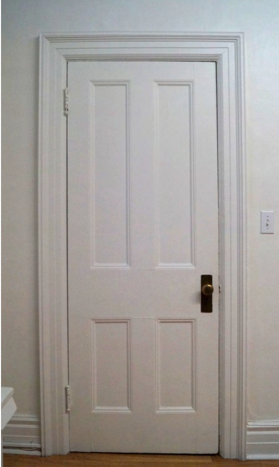
Fig. 106 Baseboard and four-panelled door in middle room on upper floor
