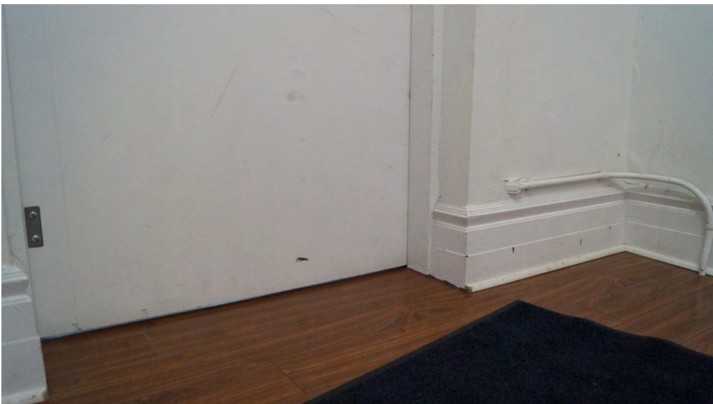
Fig. 67 Baseboard in entry hall
