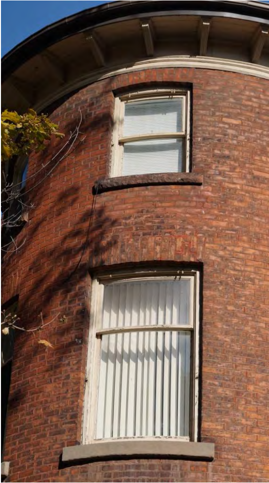
Fig. 38 Upper windows in turreted bay. Note the lower one has a parged sill, while the attic window sill is red sandstone.
