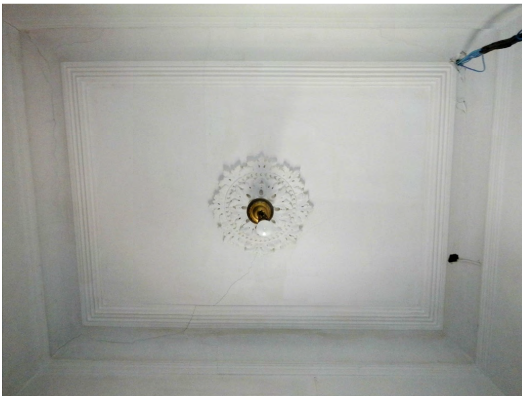
Fig. 83 Plaster moulding at cove ceiling and plaster medallion for light fixture in closet, indicating the original use of closet as the vestibule
