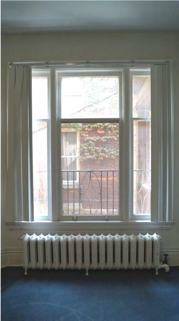
Fig. 80 Tripartite window lighting middle room
