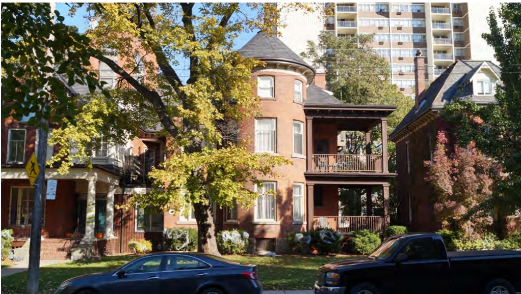
Fig. 6 56 Charlton Avenue West on the left, 52 Charlton Avenue West in the middle, and 44 Charlton Avenue West on the right
