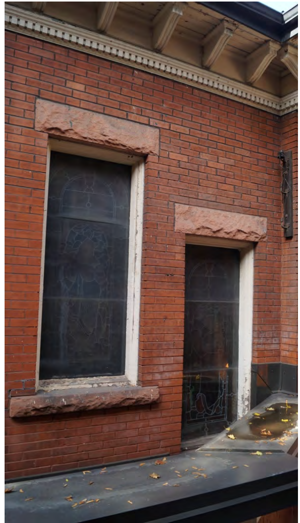
Fig. 143 East elevation's stained glass windows lighting staircase inside
