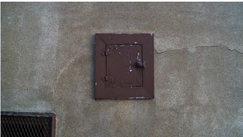
Fig. 57 Milk box door in one-storey back wing. Note parged walls.
