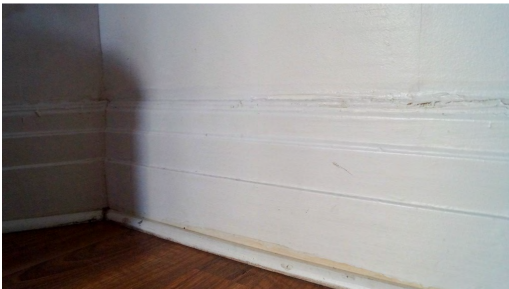
Fig. 223 Northeast bedroom's baseboard
