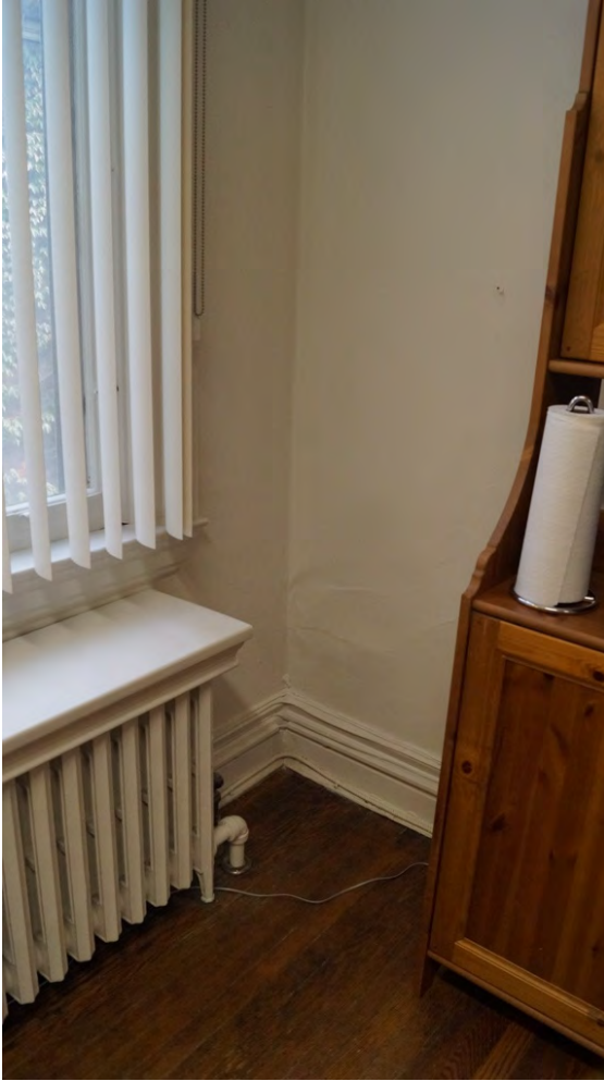
Fig. 110 Upper floor's north room oak floor, baseboard and cast-iron radiator
