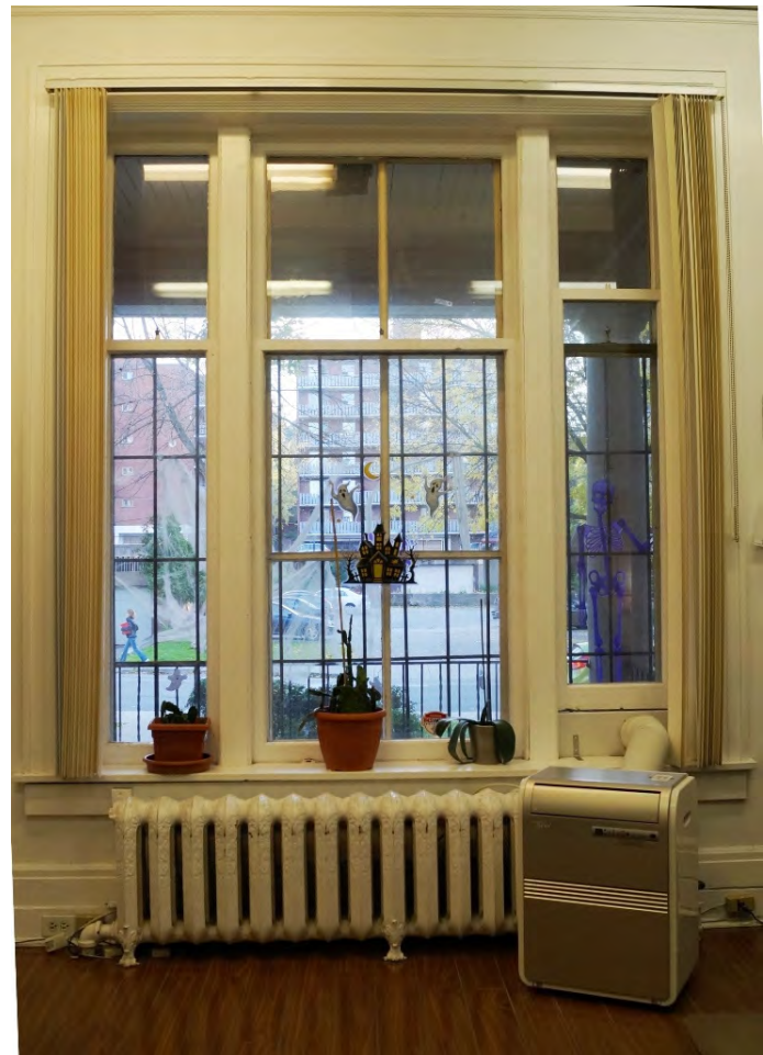
Fig. 171 Drawing room's large tripartite window with cast-iron radiator below
