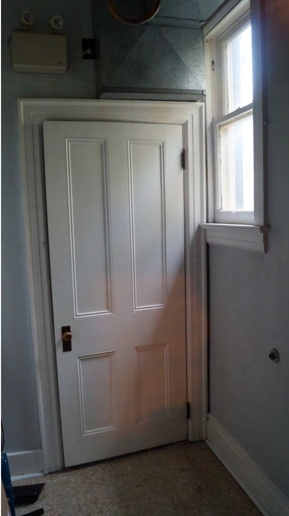
Fig. 114 Four-panelled door at back exit on upper floor
