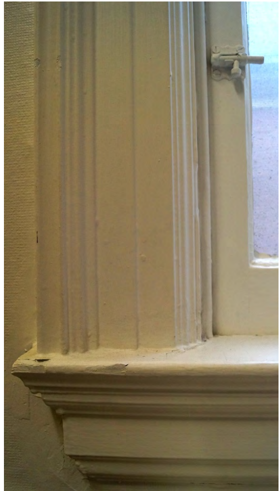
Fig. 111 Upper floor's north room window surrounds
