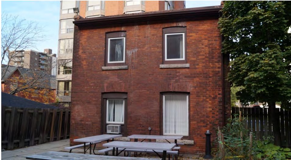
Fig. 11 South elevation of garage
