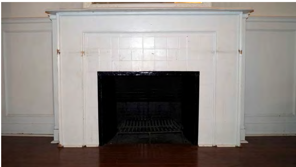
Fig. 181 Connecting room's fireplace matching the fireplace in the drawing room
