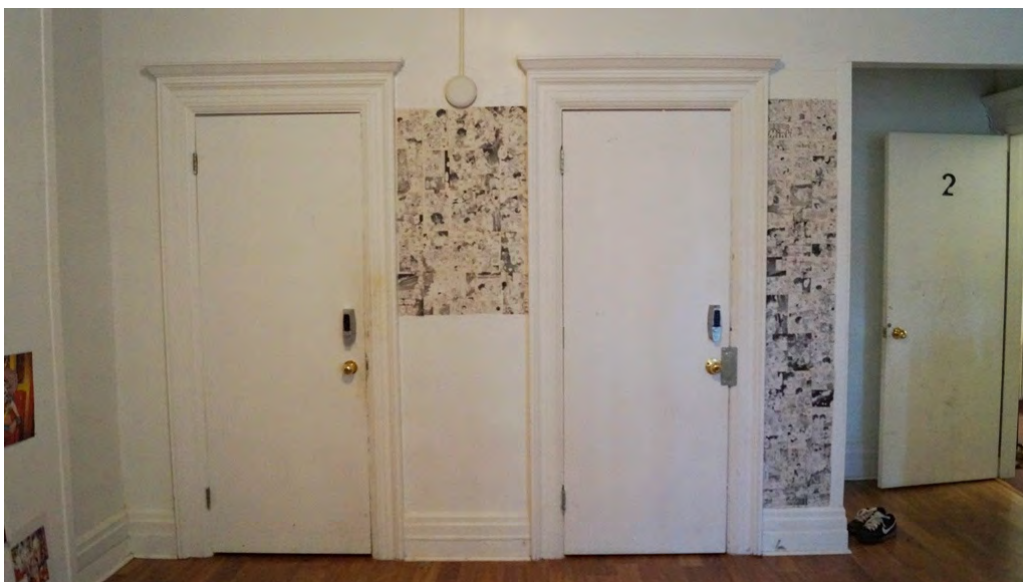
Fig. 221 Southwest bedroom's double closet doors
