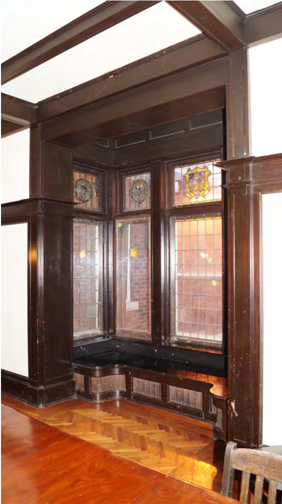
Fig. 194 Dining room's north oriel leaded and stained glass window with bench below
