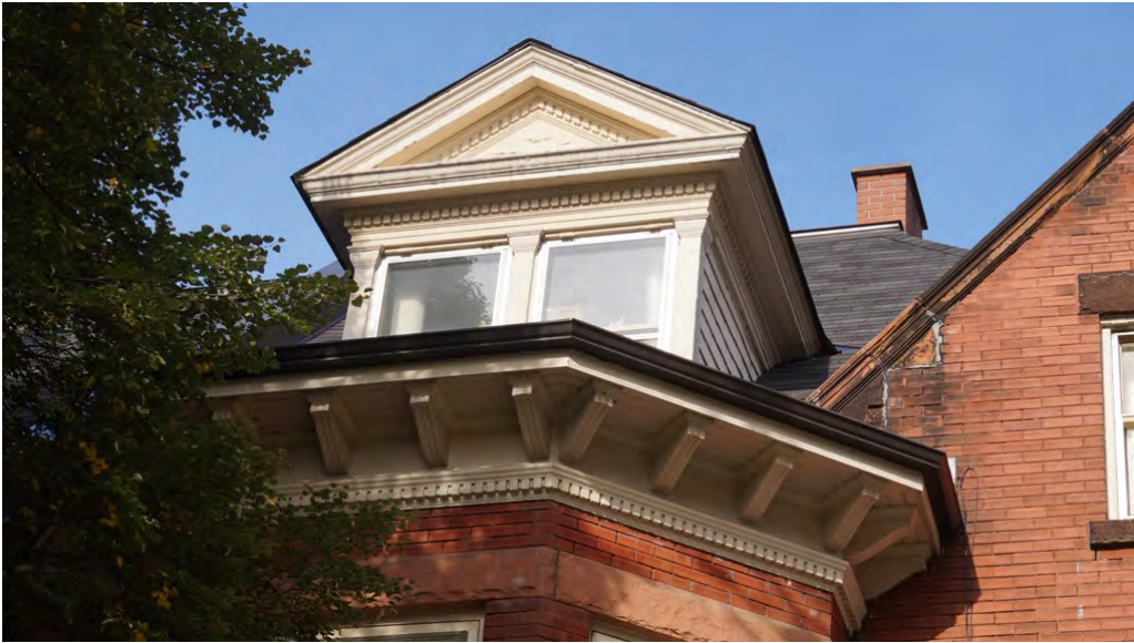
Fig. 138 Bay window's cornice with dentils and moulded brackets and pedimented dormer window above
