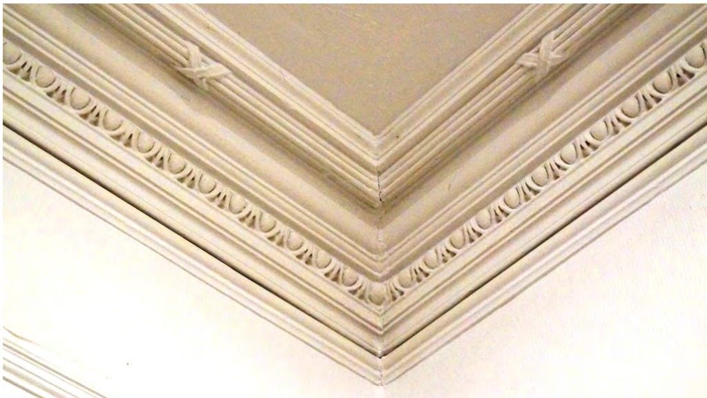
Fig. 169 Front entry stair hall's plaster cornice with egg-and-dart moulding
