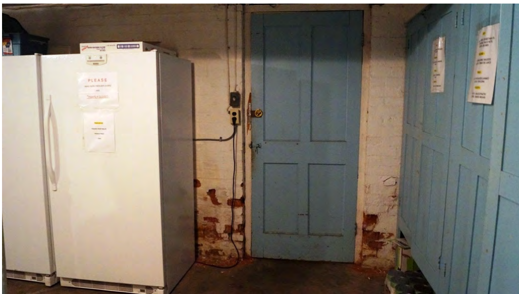
Fig. 157 Southeast basement room with cupboards and refrigerators. Note brick partition wall.
