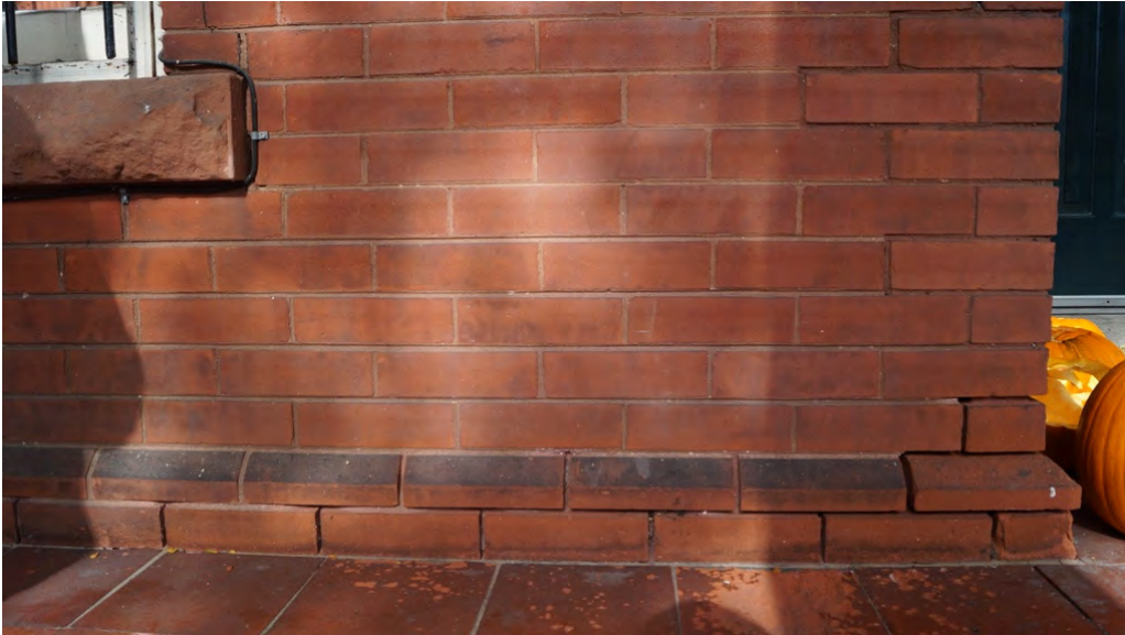
Fig. 128 Detail of brickwork as viewed from porch
