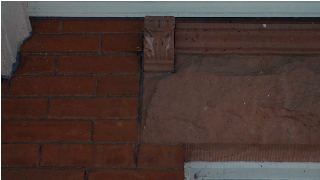
Fig. 133 Detail of ground-floor tripartite window's lintel and corbel
