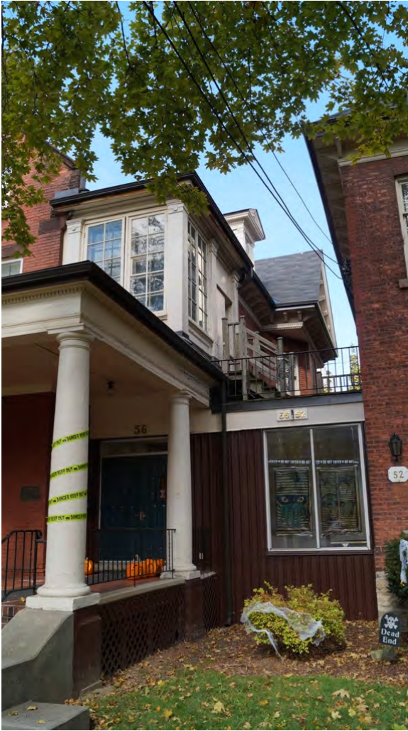
Fig. 140 East elevation as seen from front yard
