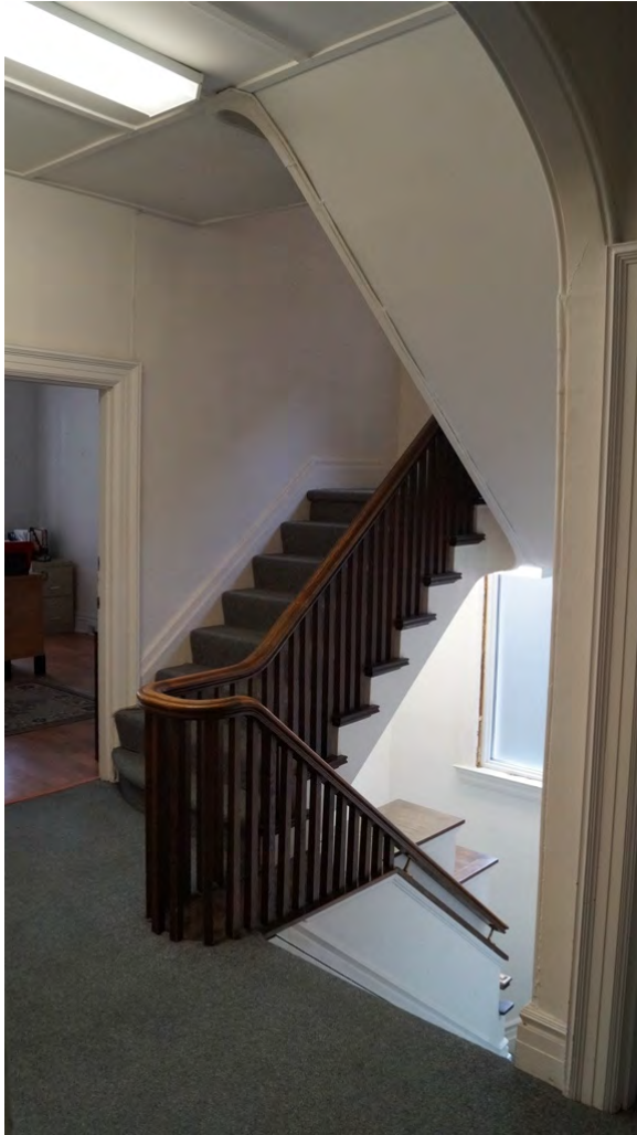
Fig. 98 Staircase at upper floor
